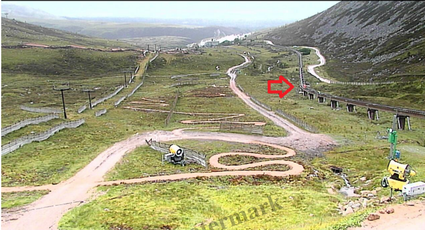
Two people working on the funicular structure on a Thursday evening
