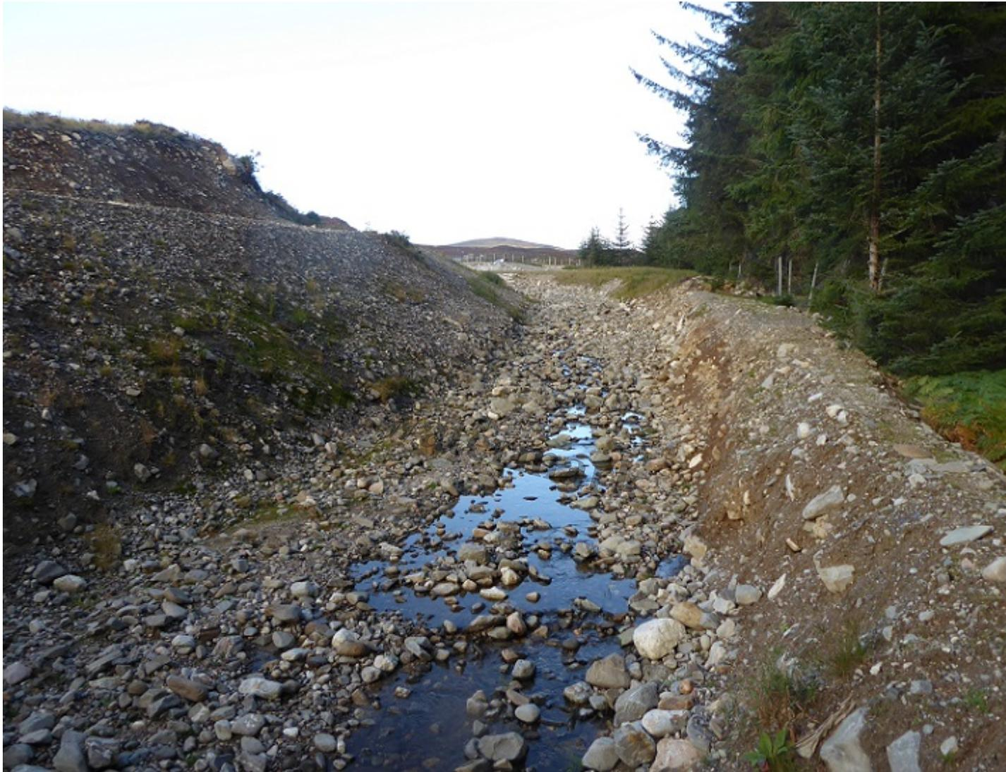
View of the upper section of the overflow from the bridge September 2020 showing eroded bank on right
