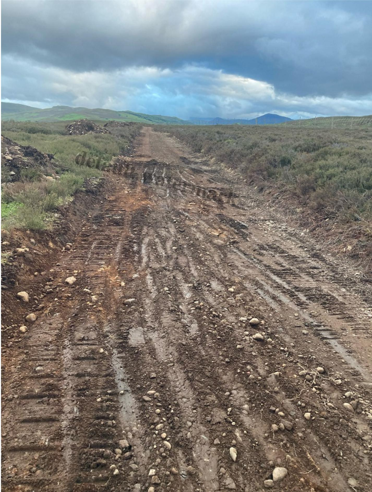
The "repairs" to the road to Far Ralia. Note how the footprint of the former military road has been widened. Photo credit parkswatch reader
