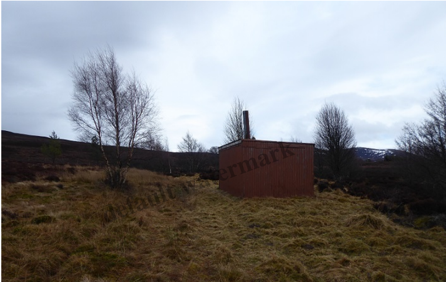
The existing Ralia estate hut within a small area of planted native woodland. 2022
