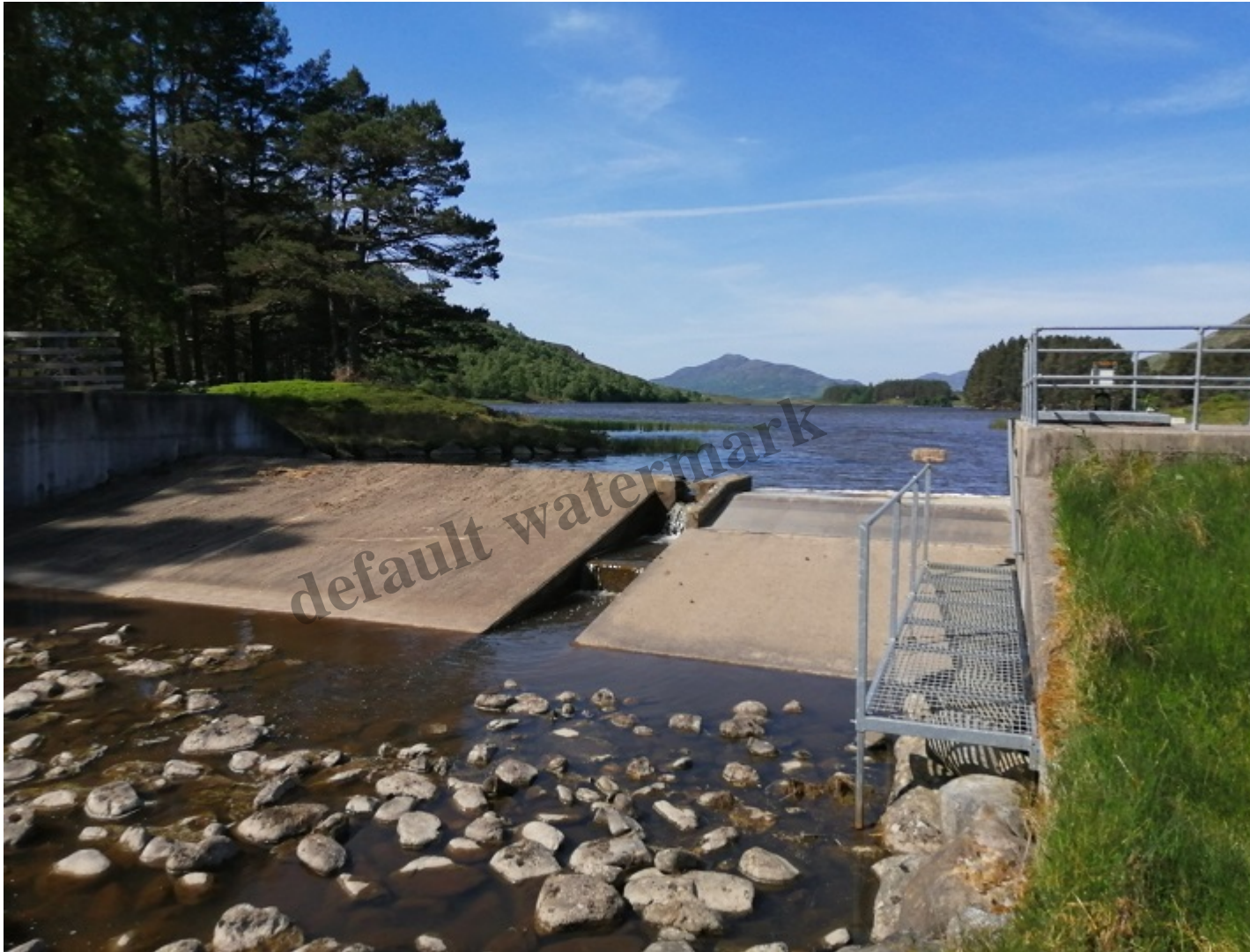
The Loch Gynack outflow, which now also serves as a hydro intake. The water on 9th June appeared slightly murky. Photo credit Parkswatch reader.
