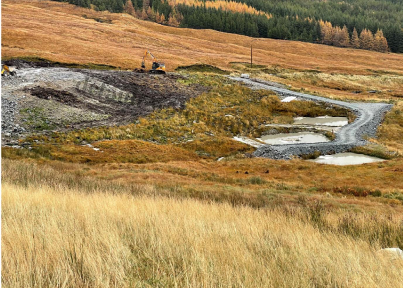
Stack 1 restoration and HEA 2 location, existing ponds to be drained prior to formation of Stack 2
