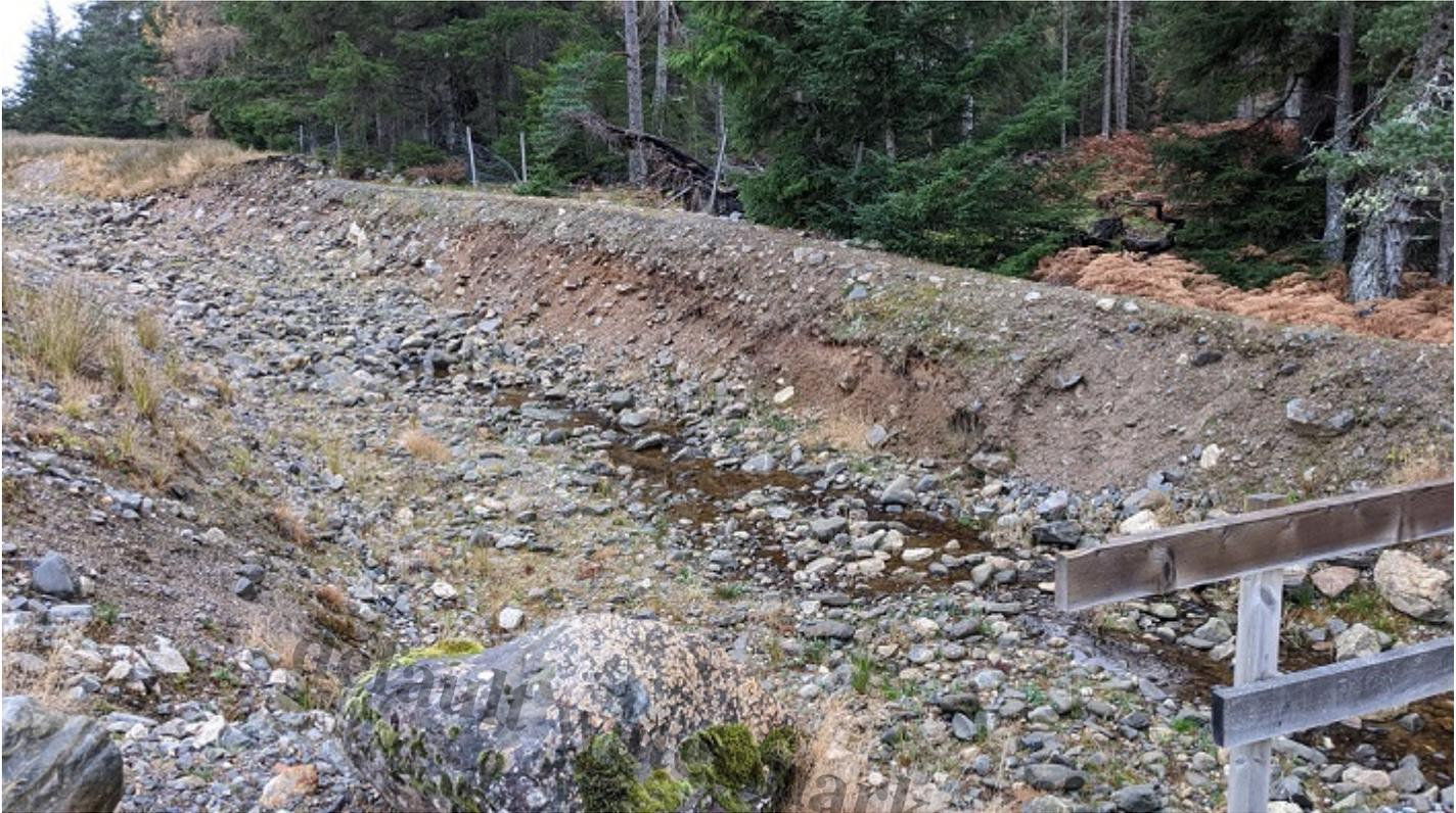
The upper part of the diversion channel with a heavily eroded section of the channel containment bund on the right. Photo Nov 2022.
