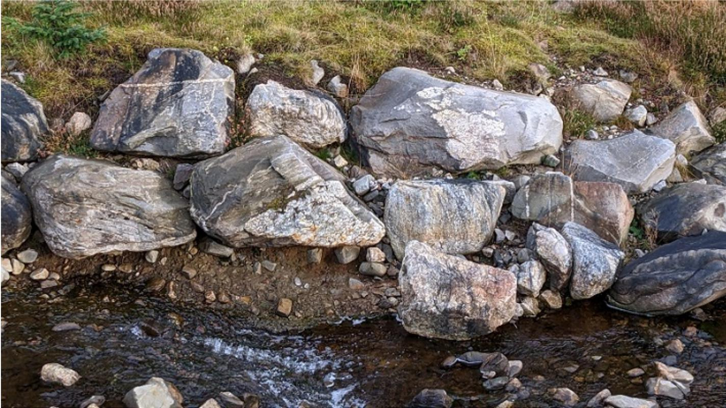
Rip rap bouldering continue to erode away below where the subsidiary burn enters the channel.
