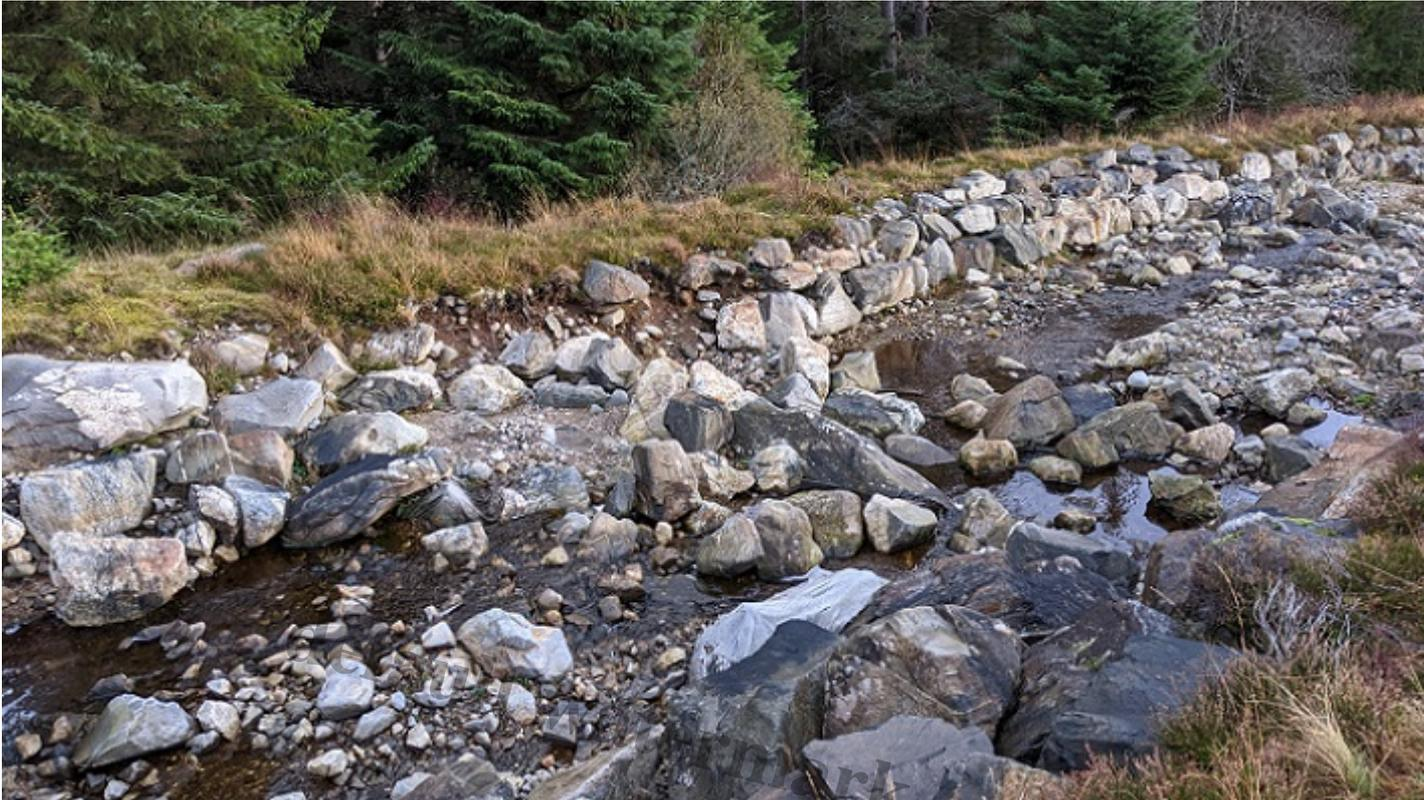
A section of failed rip rap bouldering with boulders which once formed the embankment now lying in the bed of the channel. The channel was blocked off to prevent sections like this failing and flooding the woods and Pitmain Lodge below.
