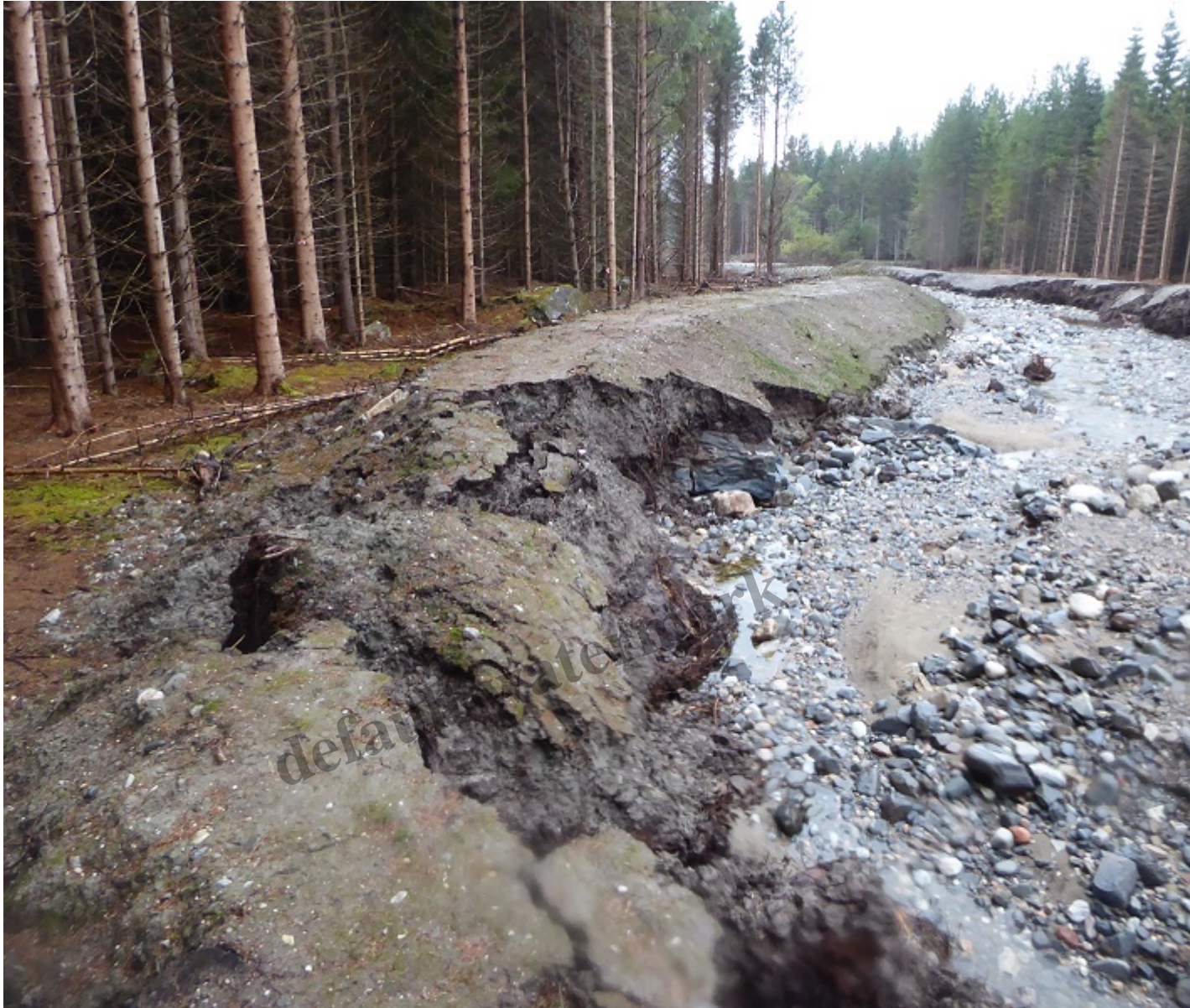
Photo of peaty sections of embankment November 2018
