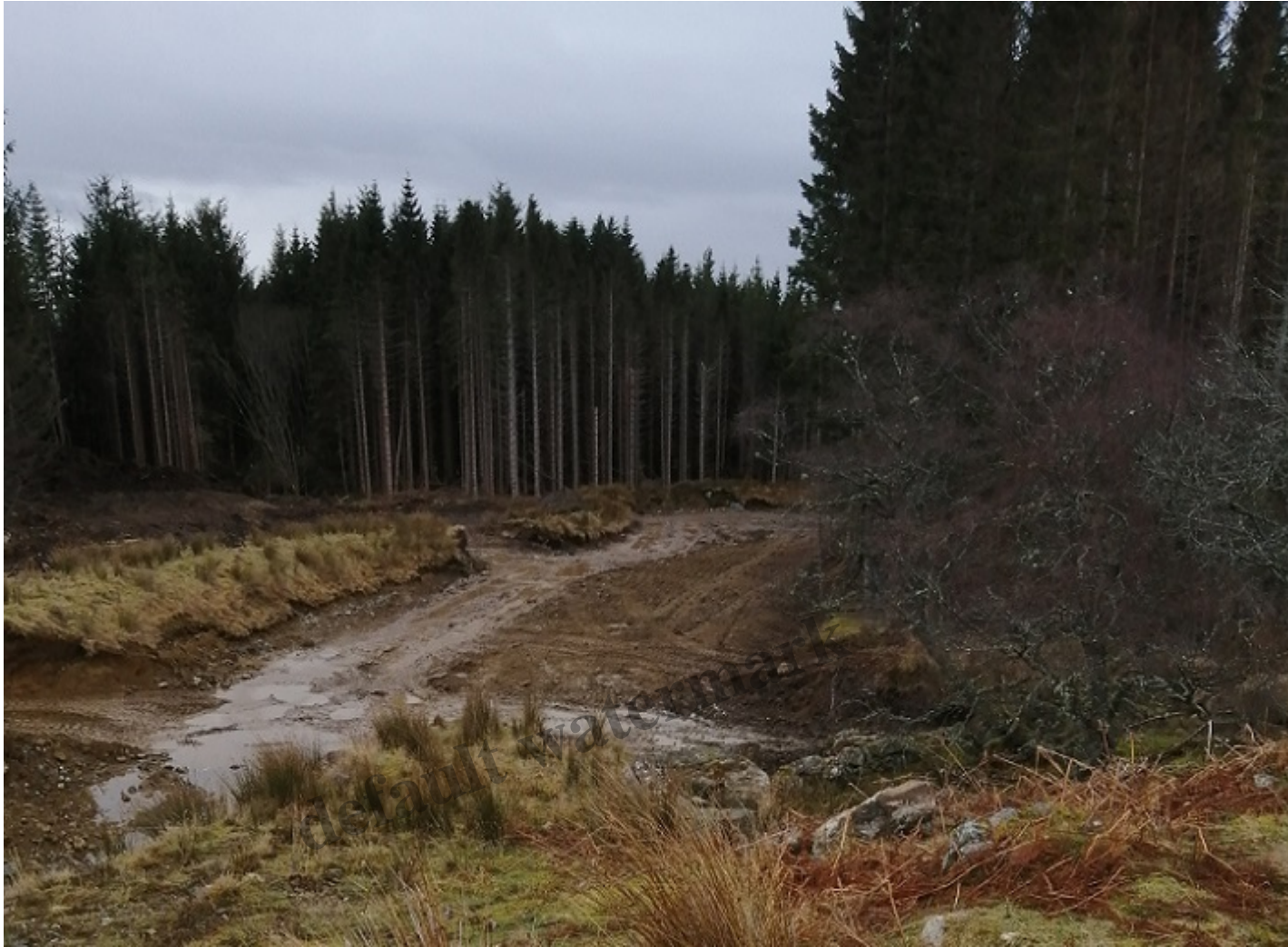
Early – preparatory? – work alongside the channel April 2023. Photo credit parkswatch reader
