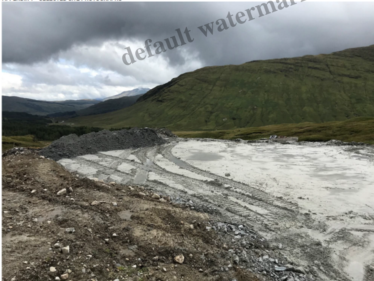
Stack 1 ongoing construction/deposition of tailings – Stack 1 at approx. 55% capacity
