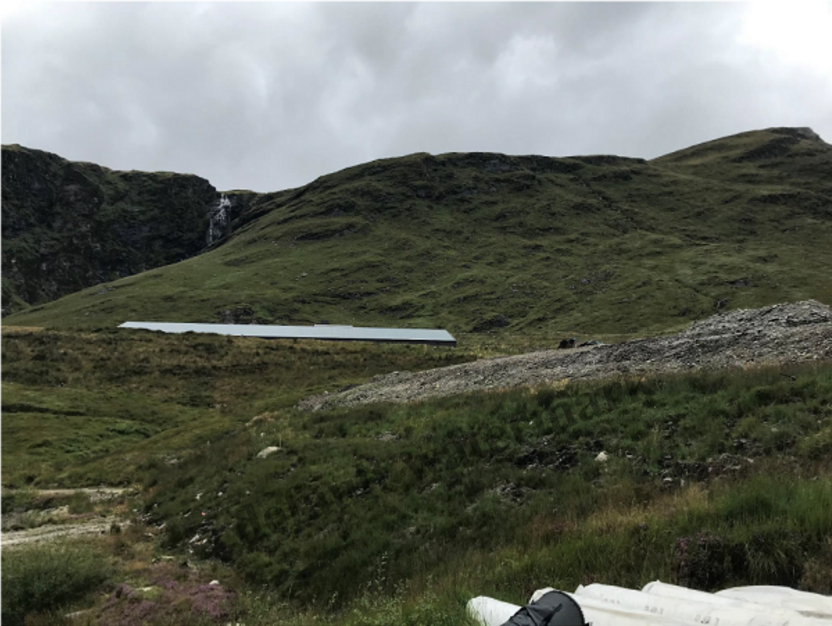
Turf placement establishing well – side of Stack 1
