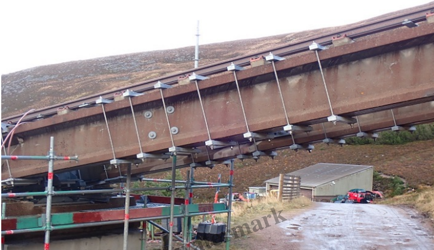
The steel rods as previously featured on parkswatch
