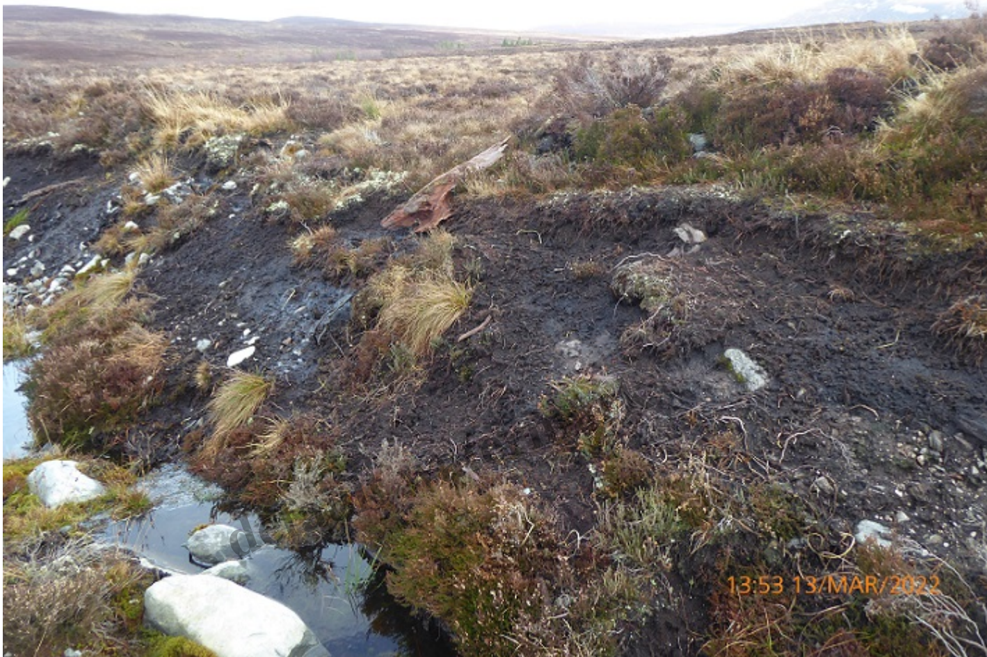
Edge of track as it cuts across the peat bog, illustrating how it has helped drain the bog.
