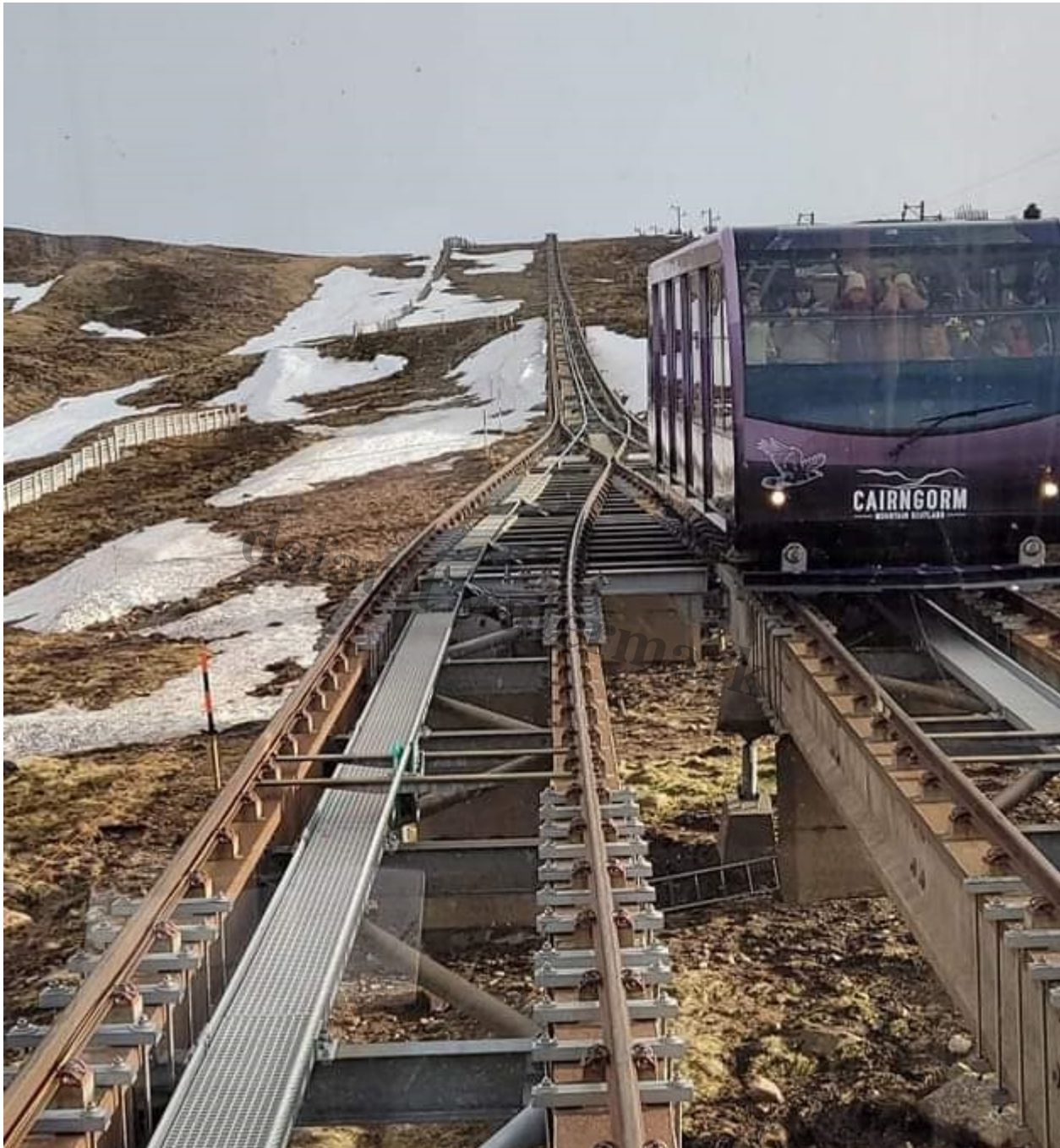
The new walkway and lots of metal brackets. Incidentally, note the state of the ground below! Photo from FB
