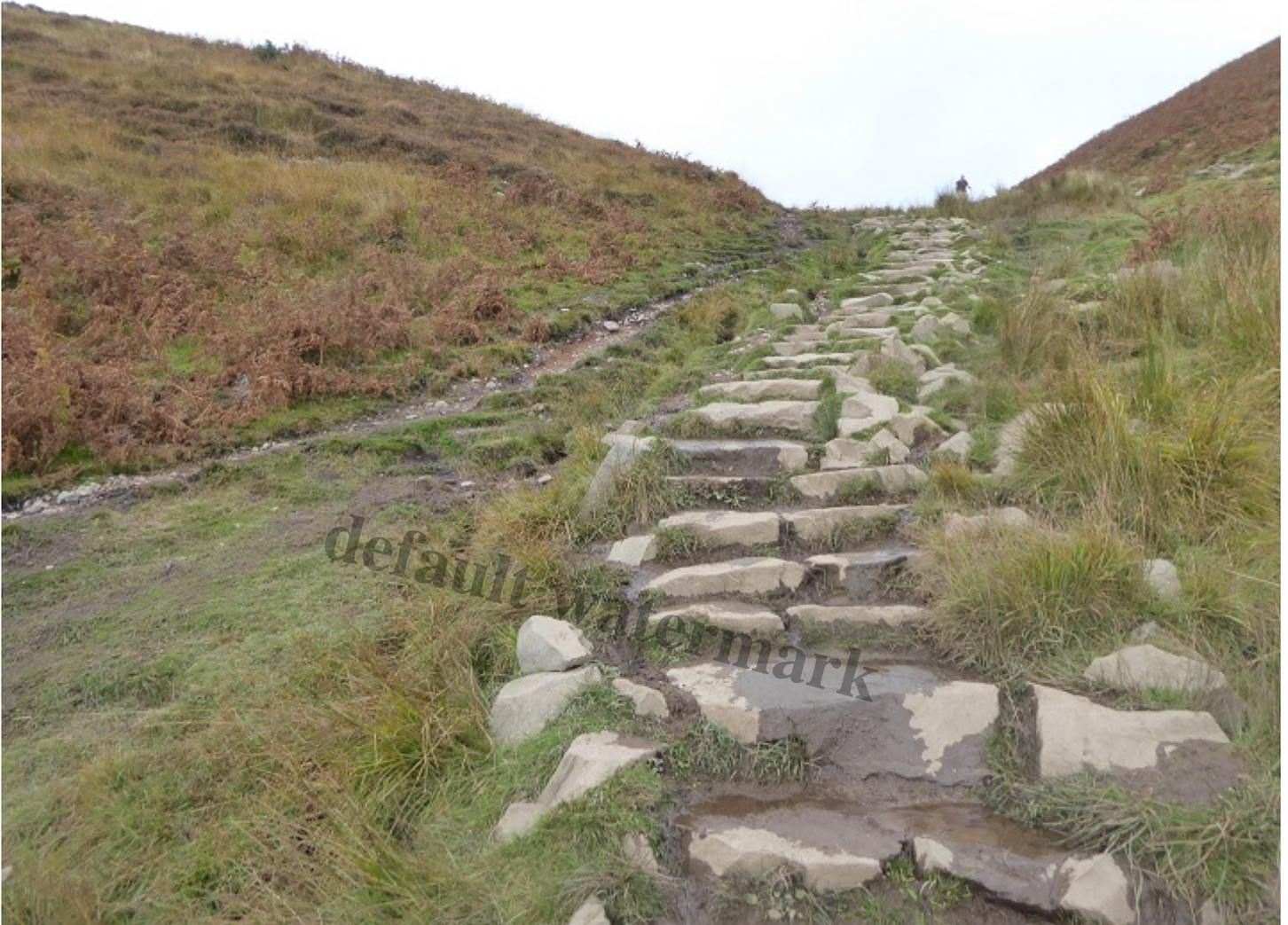
The stone pitched steps on the section of the Conic Hill path below the two photos above has survived much better. This is despite the narrowness of the path and high volume of use which makes passing people difficult and would normally force people to step onto the ground on either side (note the rocks on the right hand side designed to stop this happening). That contrasts with a lower section of stepped path:
