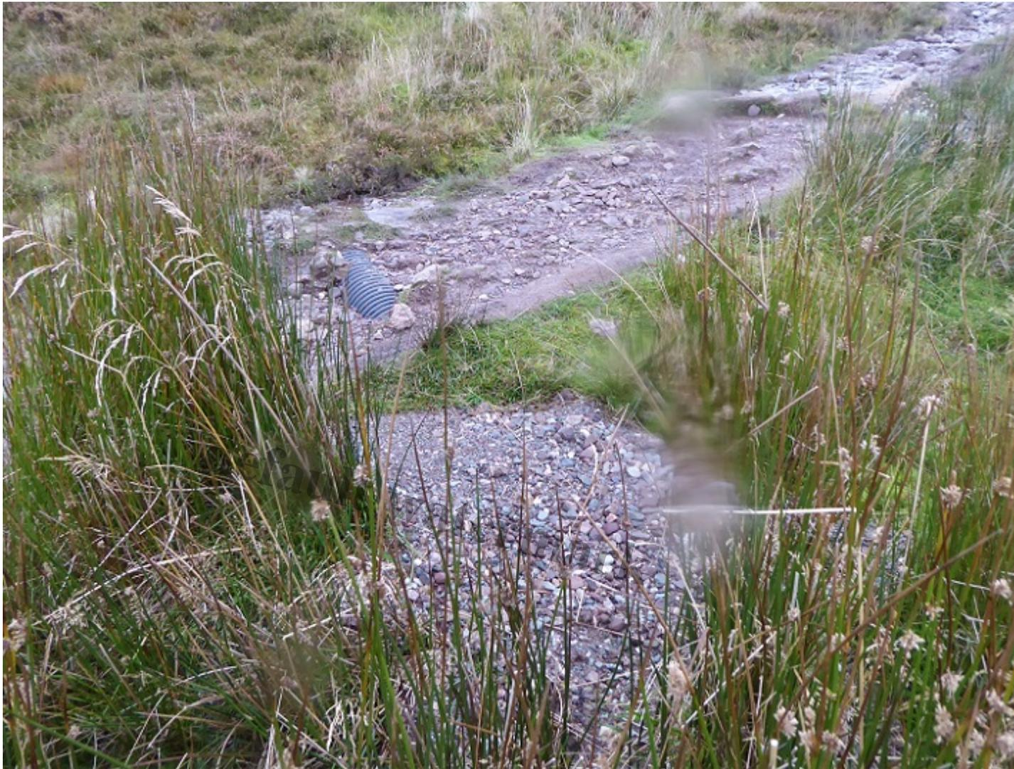
Evidence of surface wash out. Some of the finer material is likely to have found its ways down into the Burn of Mar and the River Endrick Special Area of Conservation
