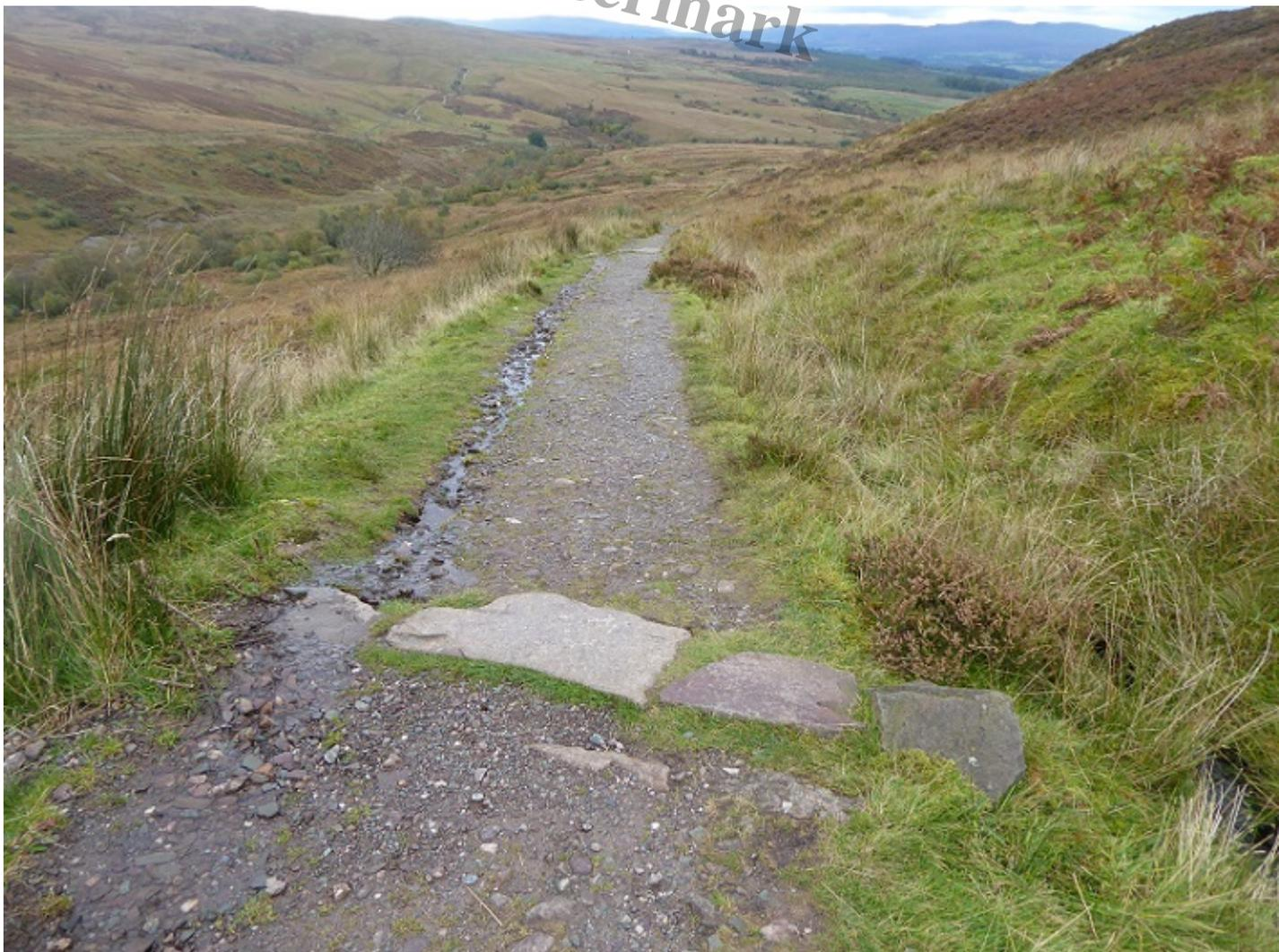
Looking towards Burn of Mar October 2020. The drainage ditch on the right has been successful but lack of maintenance of the step/water bar has allowed the left side of the path to develop into a small burn
