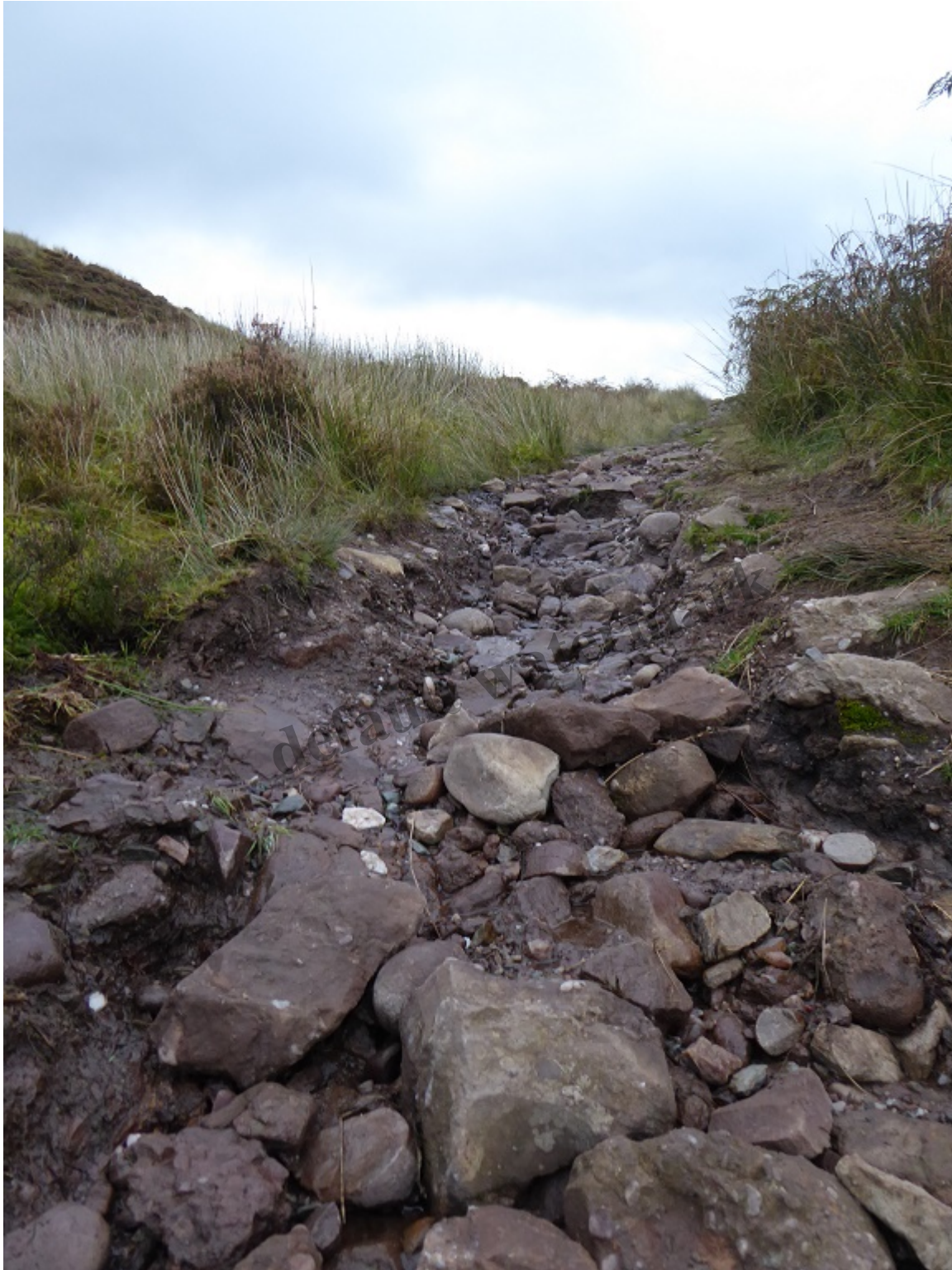
It is not a surprise that in consequence all the path surface has washed away
