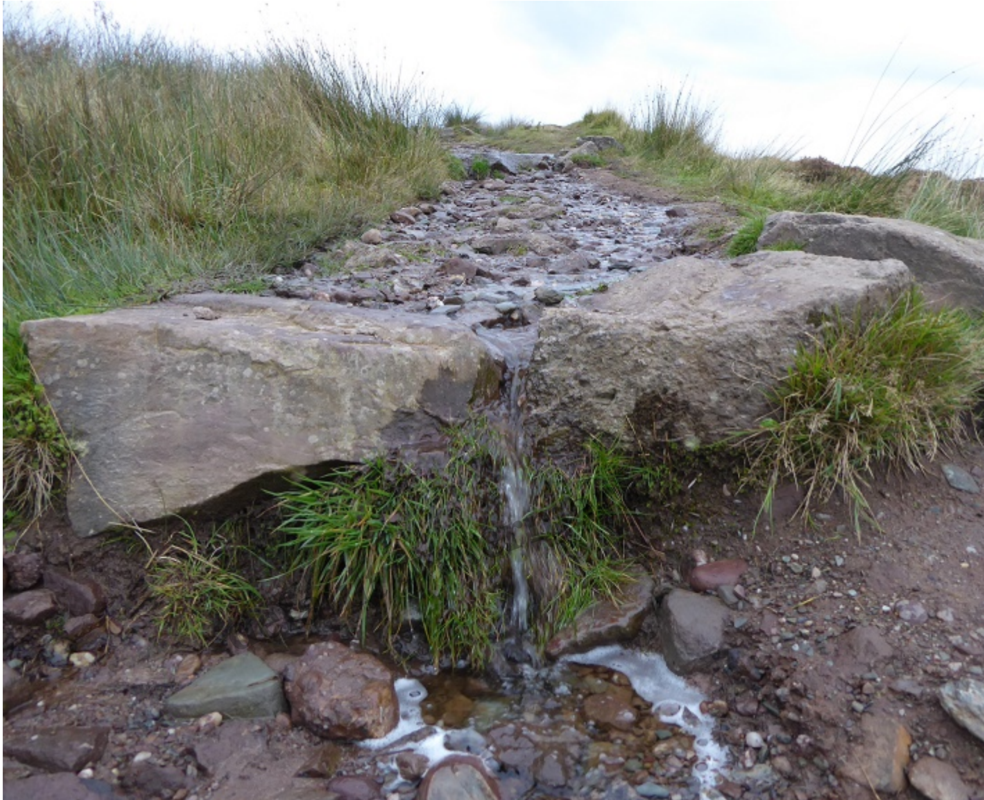
In places the path is now a burn, with mini waterfalls and impassable steps. Photo October 2020.
