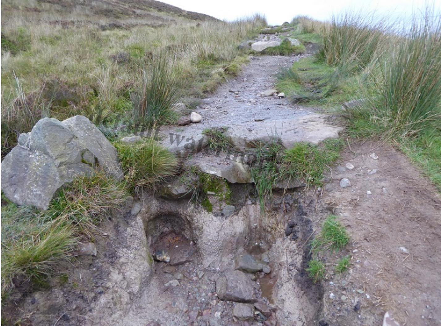
Filling up the hole with aggregate will not solve the problem, this needs stone pitch steps plus the creation of effective waterbars. Photo October 2020
