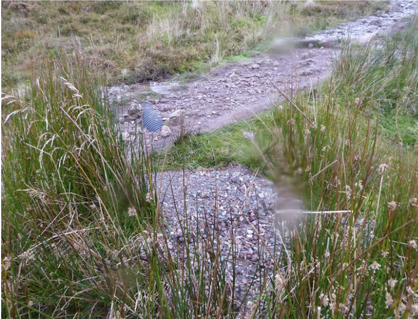
Evidence of surface wash out. Some of the finer material is likely to have found its ways down into the Burn of Mar and the River Endrick Special Area of Conservation
