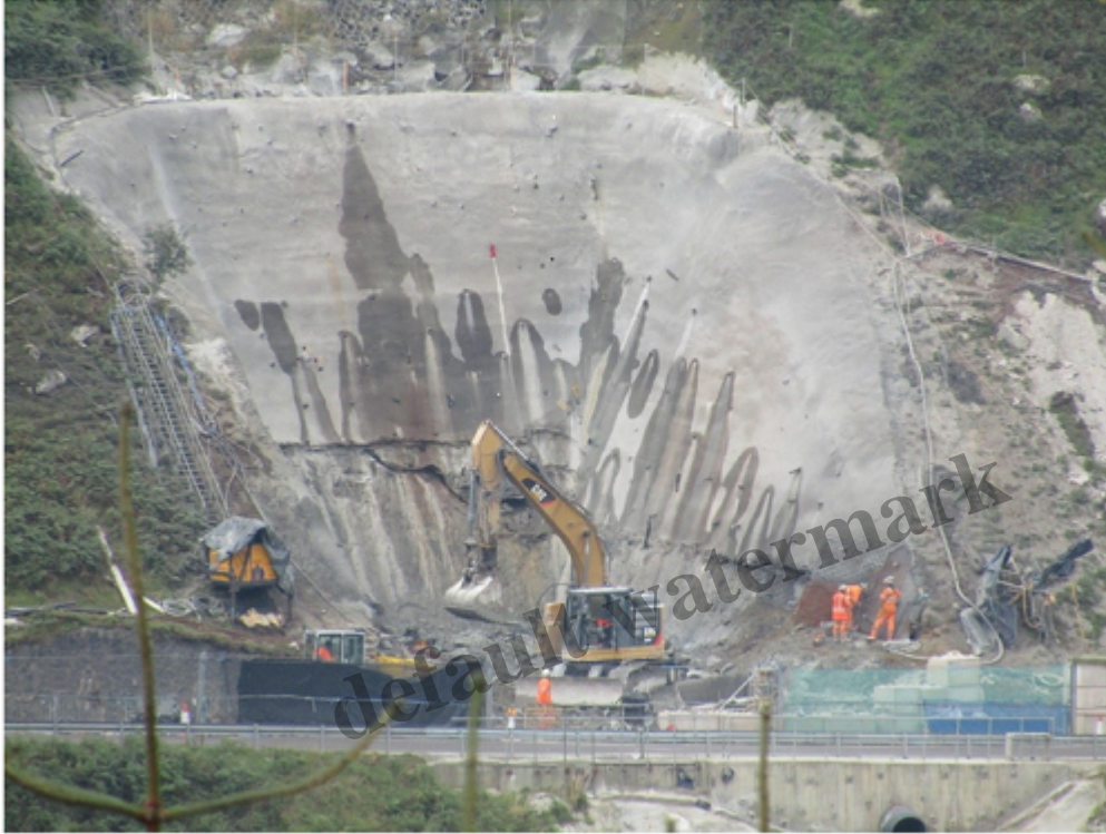
Catch-pit 3B construction progress in September 2022
