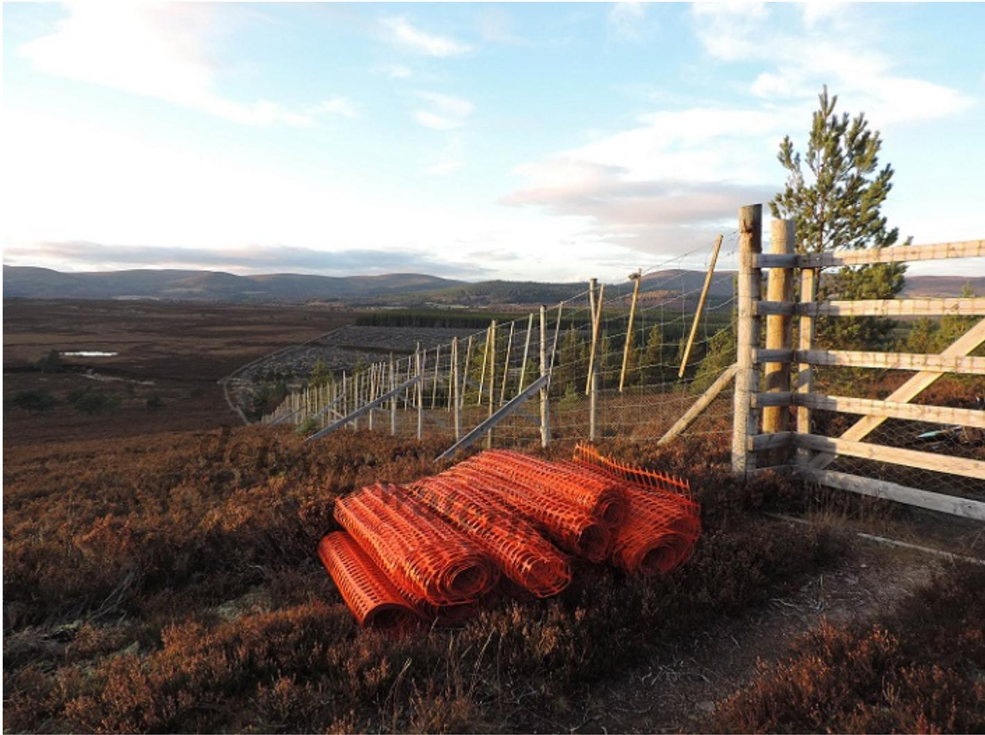
Are the batons that have replaced the netting close enough for capercaillie to decide there is no way through? The challenge with this location is that it is exposed to the wind and if there is too much marking on the fence it risks blowing over. Photo November 2022.
