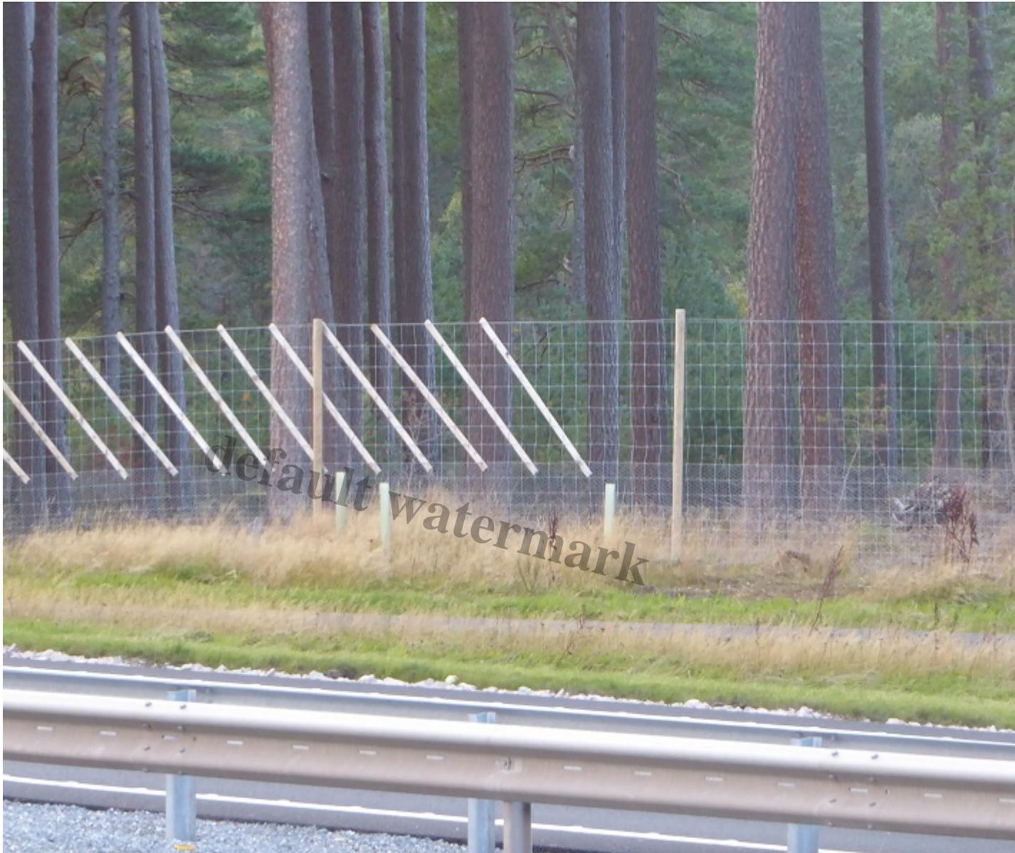
New marked and unmarked fencing October 2018 along the A9 dual carriageway between Aviemore and Kingussie. The wooden batons in the photo are close together and extend onto the bottom half of the mesh which should help reduce but not eliminate birds collisions
