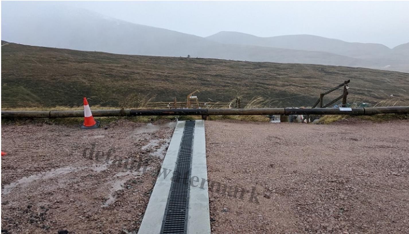
Unfinished work with the drain line protruding above the surrounding ground. Note how water is already eroding the surface on the left.
