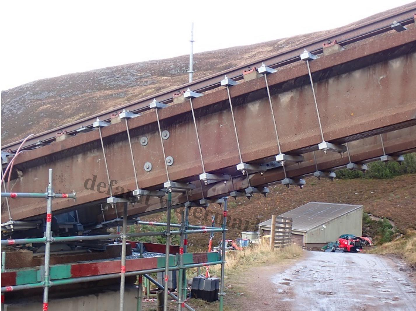
Metal braces to strengthen the concrete beams. Note there are seven braces on the beam in the foreground but only six visible on the one to the rear.
