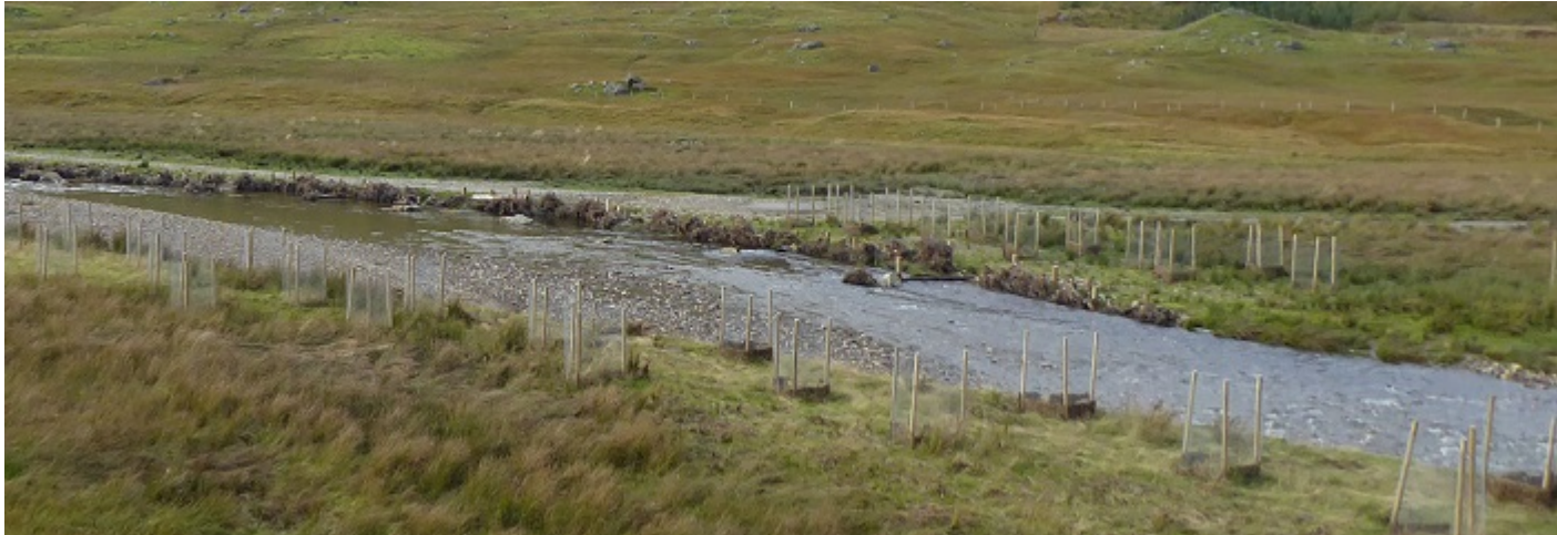
Works to stabilise the river bank visible left of centre
