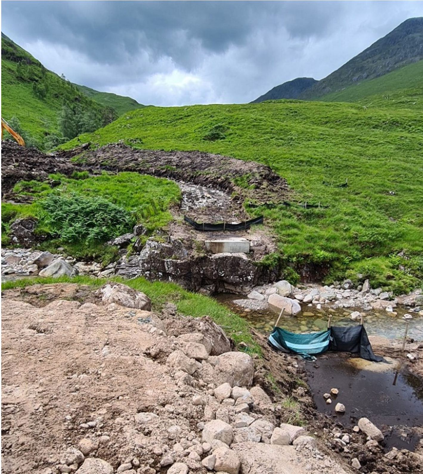
Construction track through peat to the intake with concrete foundation for bridge
