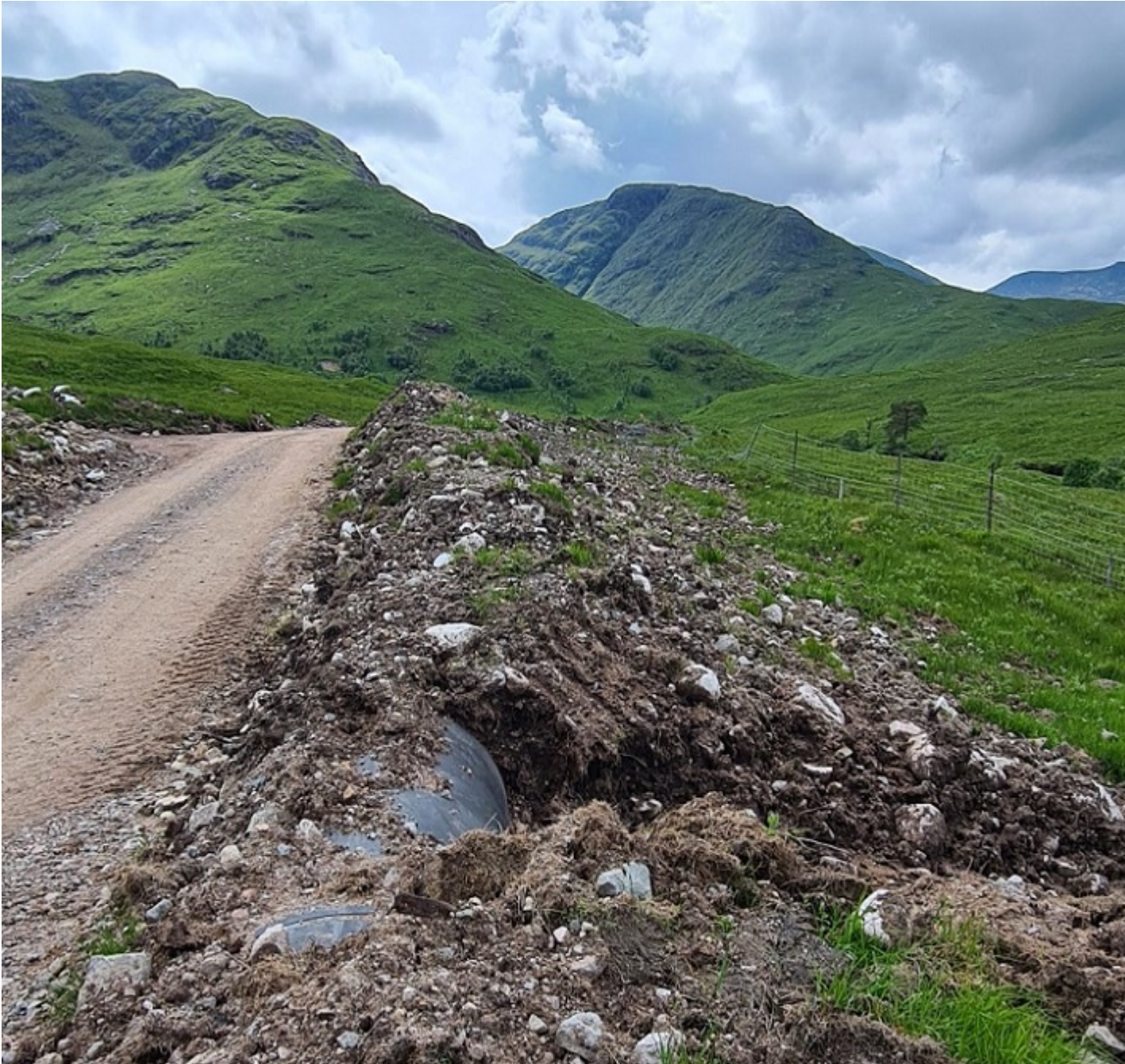
The construction track and pipeline to the intakes.
