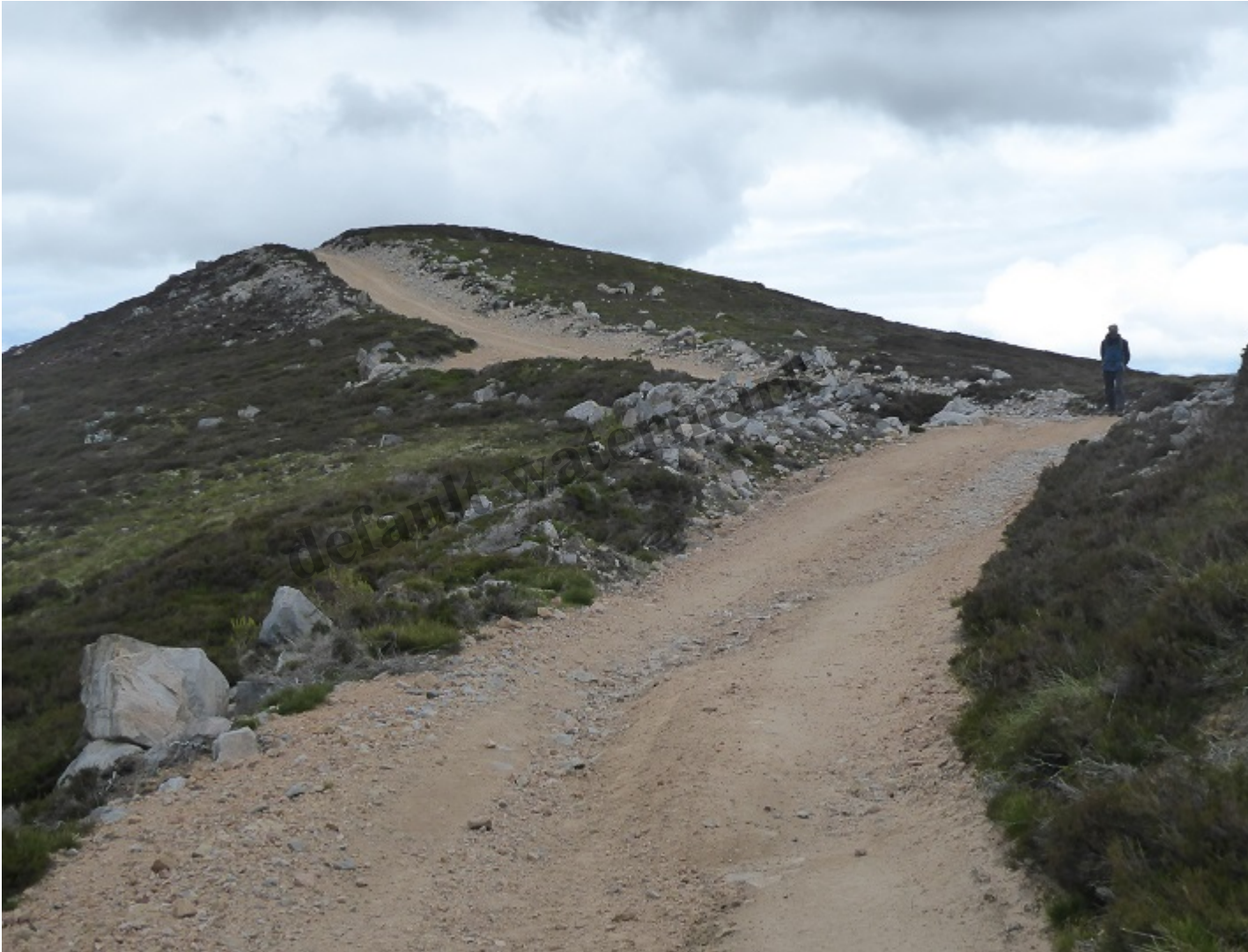
The upgraded road over the knoll north of Creag n'h Iolaire within the National park boundary
