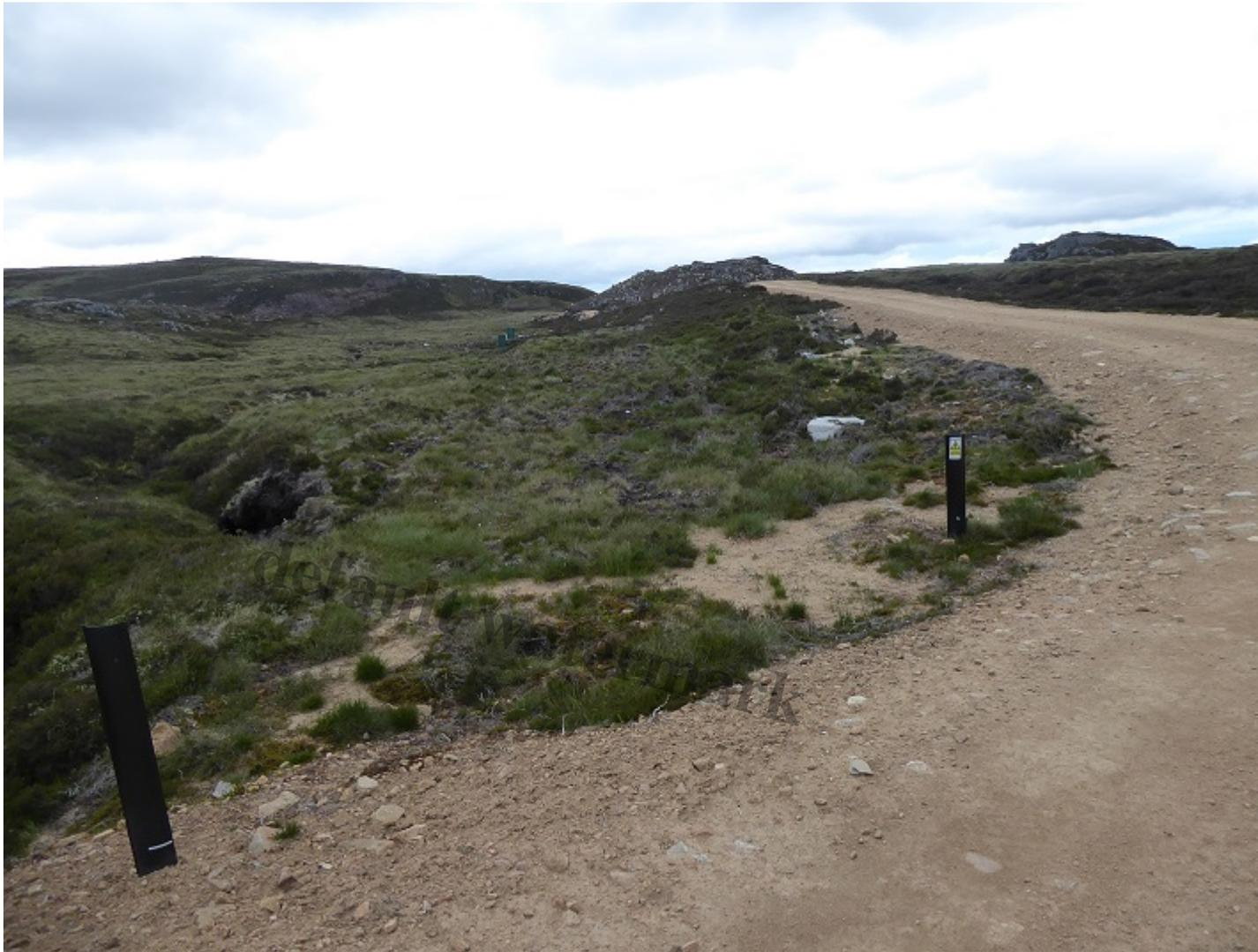
Two electricity boxes are just visible in the middle distance beyond the plastic line markers. Note how silt and grit from the road is being washed down onto the peat.
