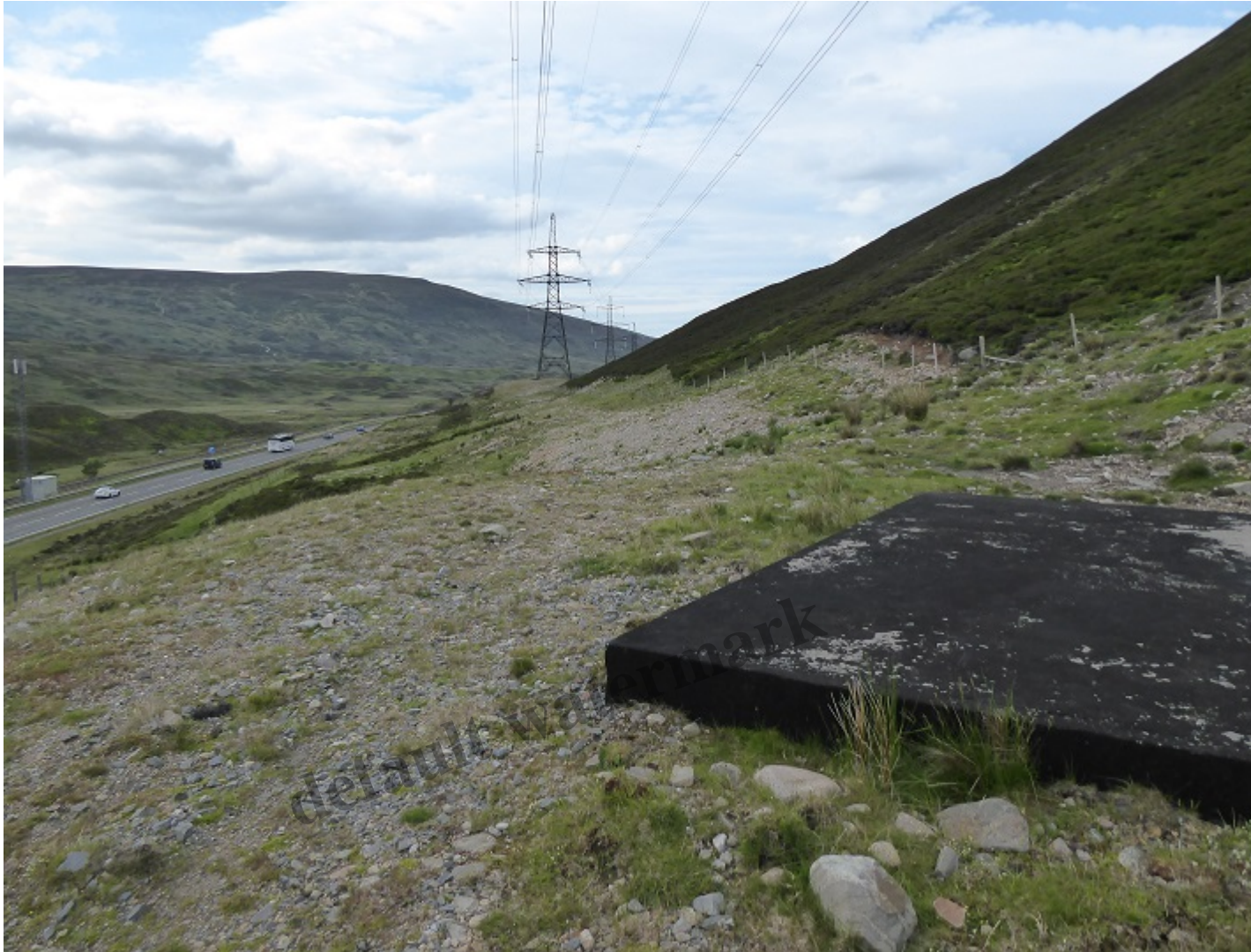
View back from tower 144 to tower 143. The extent of the construction impact here is hidden from the A9 below because of shape of the slope
