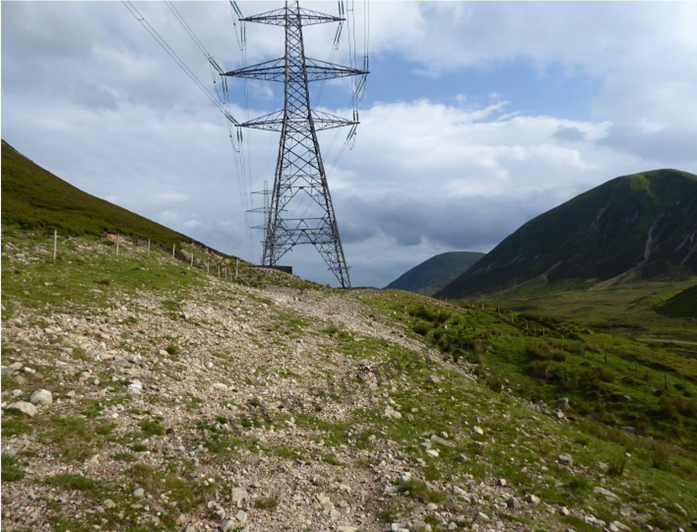
Approaching tower 144 with the line vehicles have driven still visible.
