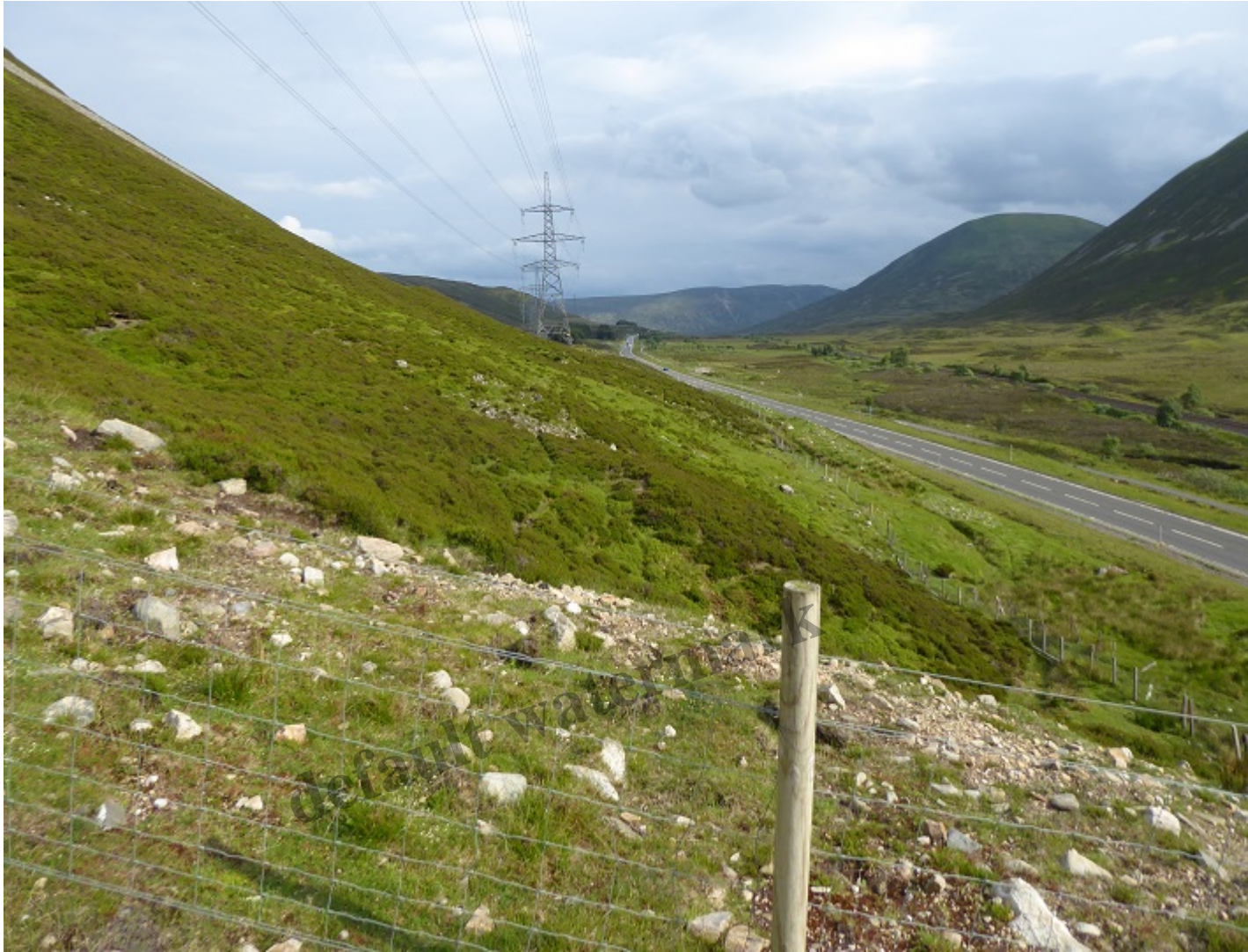
View from edge of stock fence and tower 145 to tower 146
