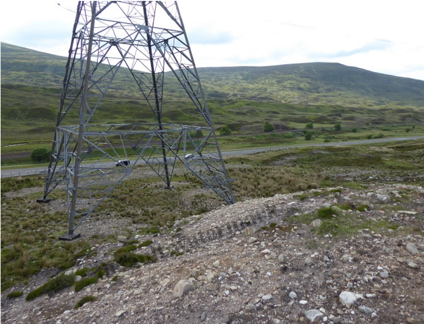
The area around tower 141
