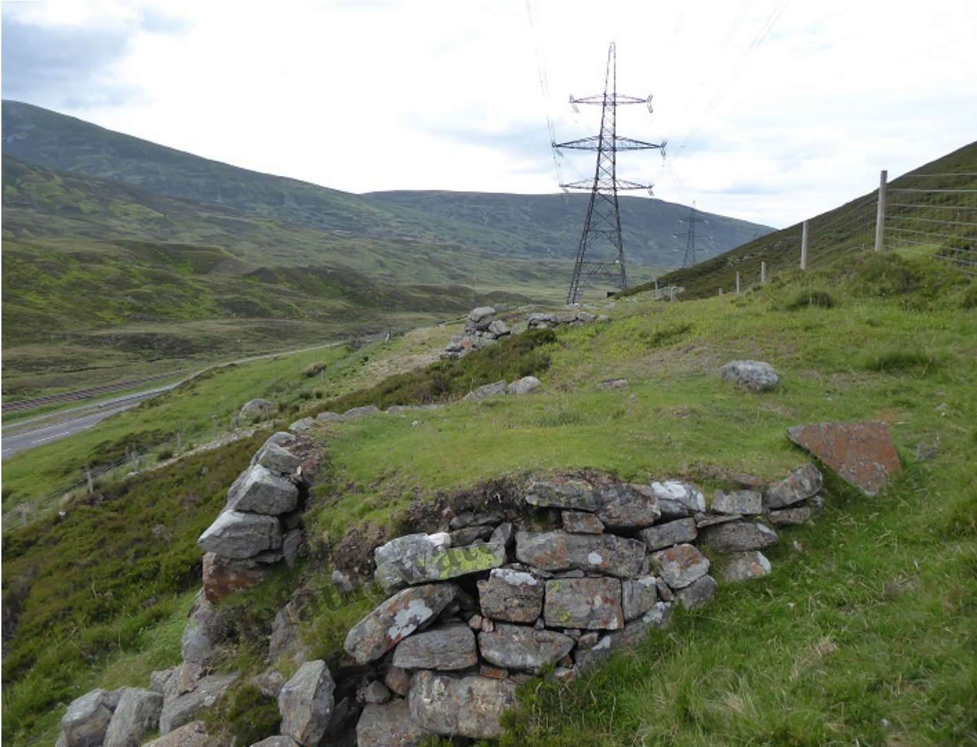
View back towards tower 144 with the footings for the old powerline towers in the foreground
