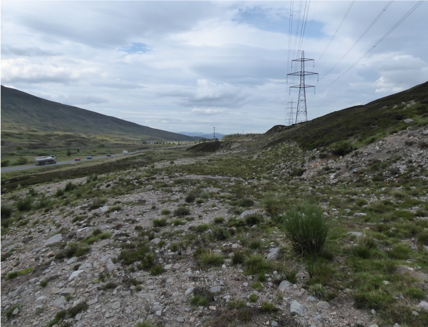
View from tower 141 to 140. This part of the trial restoration area is visible from the A9 and forms the start of the long landscape scar that runs to the policy woodlands around North Drumochter Lodge
