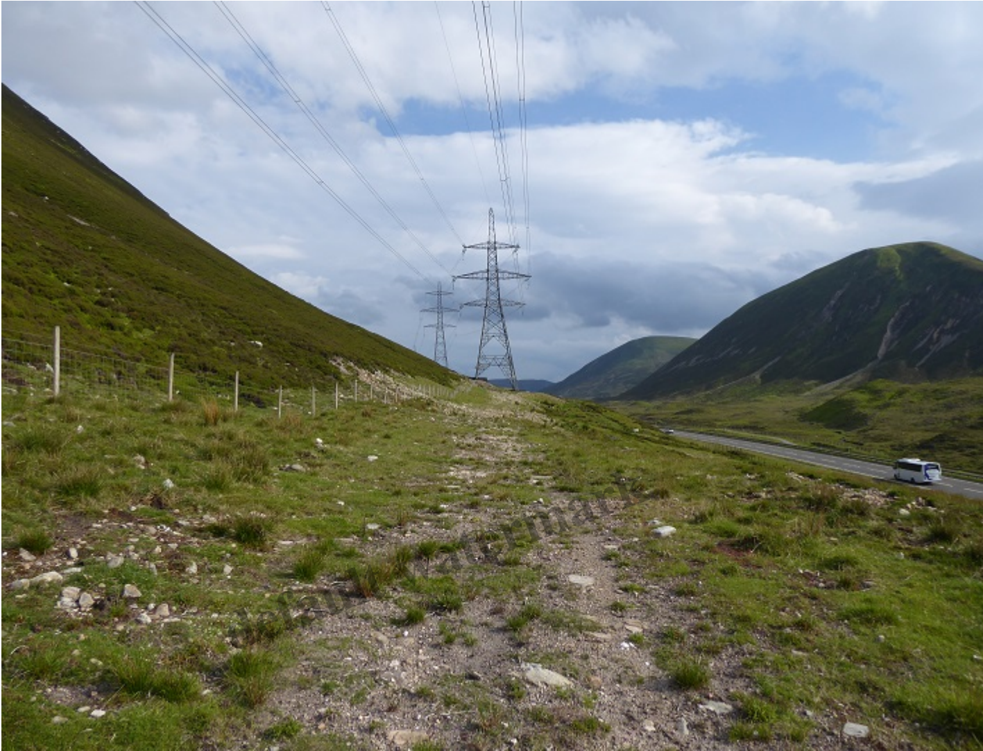
ATV track line running along the Beauldy Denny construction track towards tower 144
