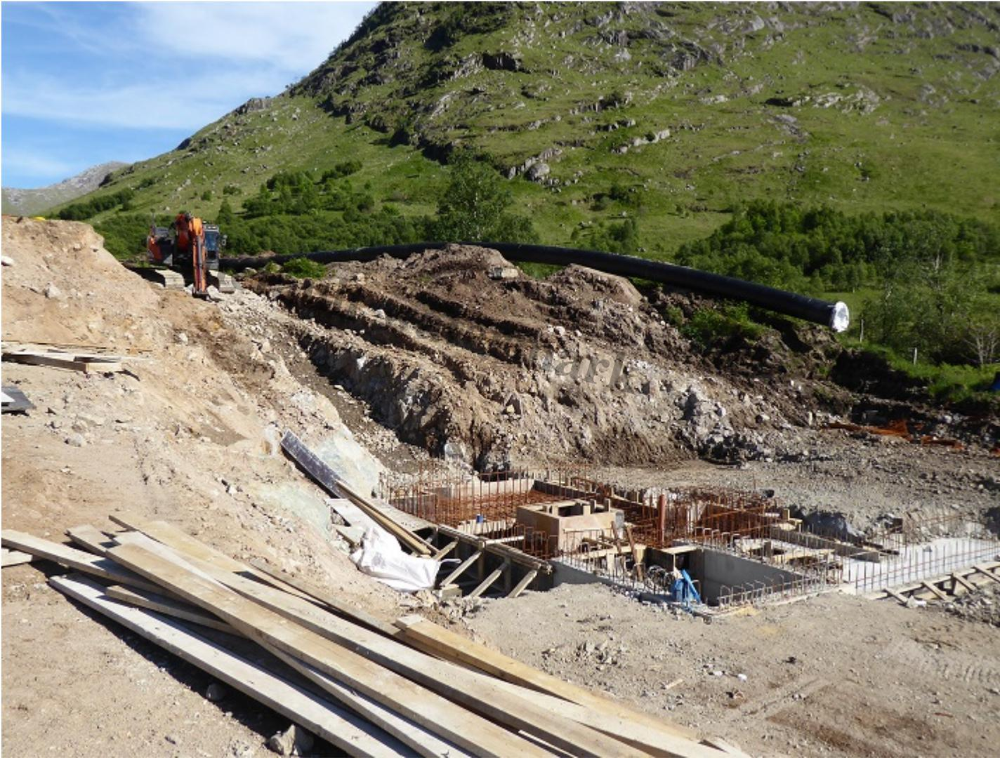
The Allt Ceitlein hydro powerhouse under construction. The pipe has been placed prior to being buried in the trench that has been excavated through the rocks above the foundations.
