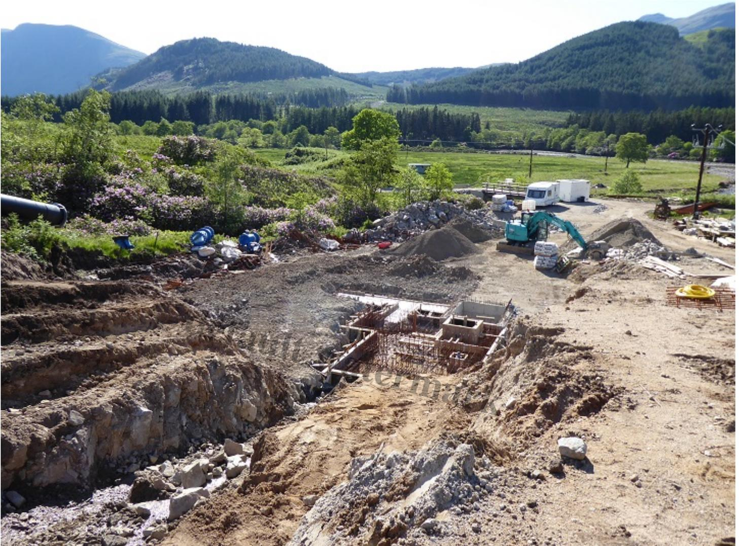
Back to the beginning, the pipeline trench through the rock viewed from above. The intake area looks absolutely dire at present but in the medium term the presence here of trees and invasive rhododendron means it is likely to disappear from view far more quickly than the Allt Ceitlein hydro intake.
