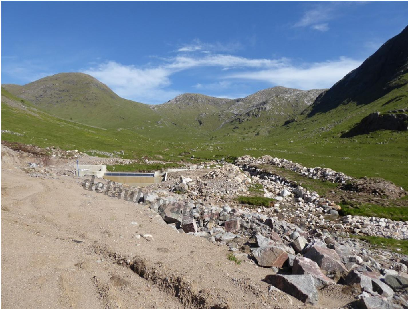
View of the intake from below, with the temporary diversion channel to the right. The rocks in the foreground sit above the pipeline.
