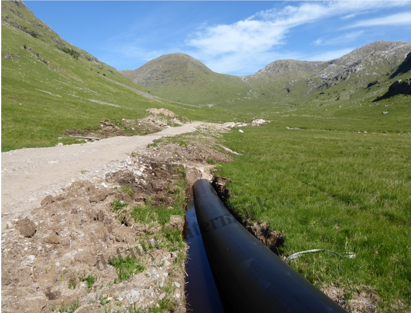
Looking back from where the pipe is about to be buried
