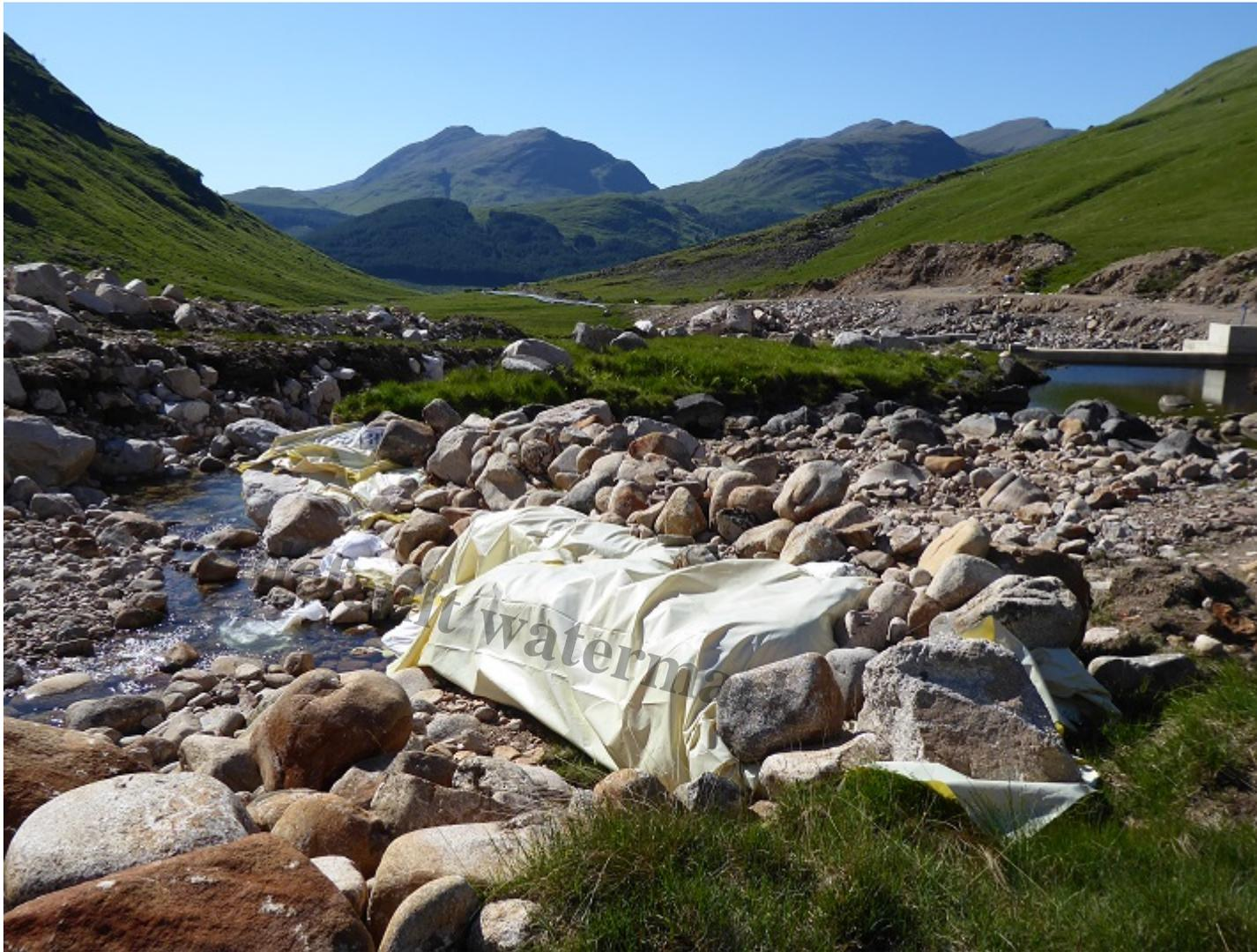
Approaching the Allt Ceitlein intake from above. The river has been diverted from its original channel to enable the intake dam (right) to be constructed. Once the intake is finished the plastic and boulder blocking the original channel will be removed and the temporary channel blocked up.
