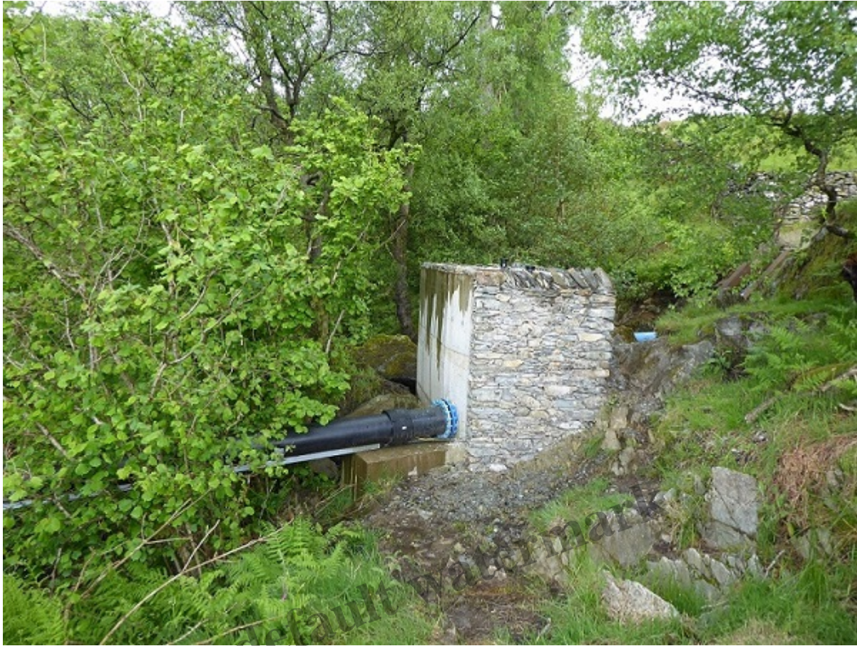
The start of the pipeline
