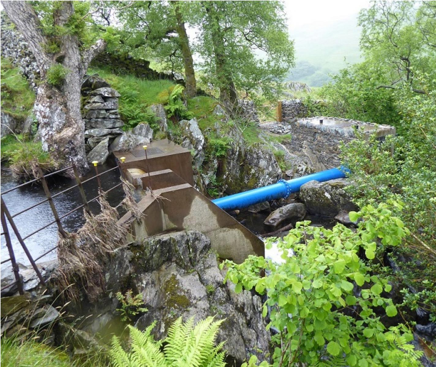
The intake was cleverly located and hidden among trees while the intake chamber was clad in stone about the blue penstock!
