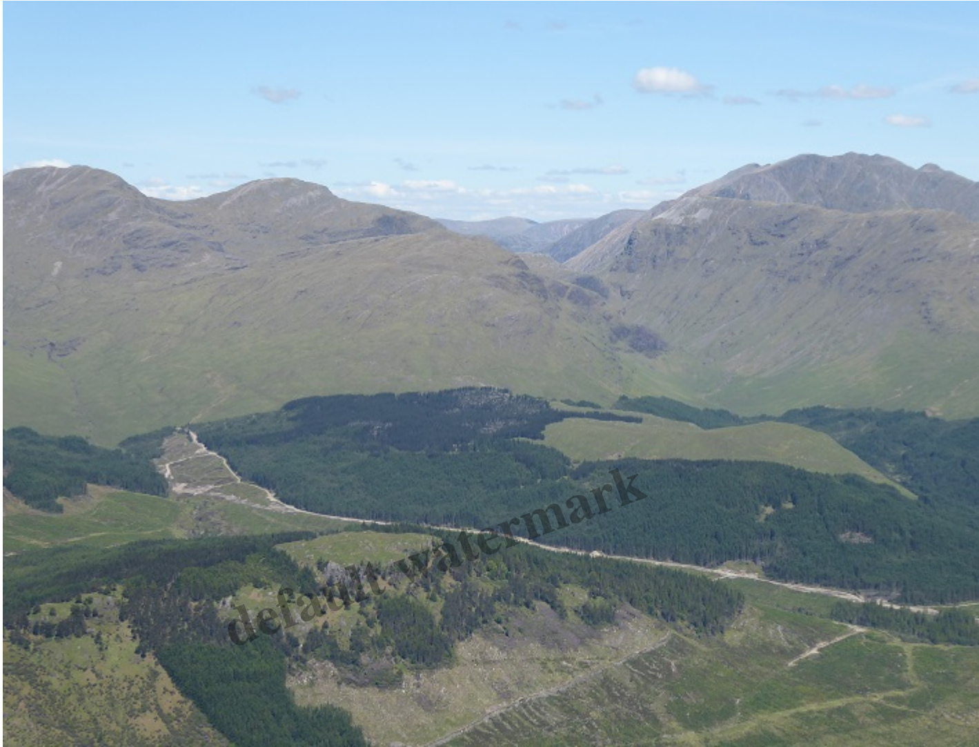
The enlarged forestry track (5) leading to the Allt Gaoirean hydro intakes, with a section of restored pipeline (4) visible bottom left. Beinn Sgulaird is on the left and Bidein nam Bian on the right.
