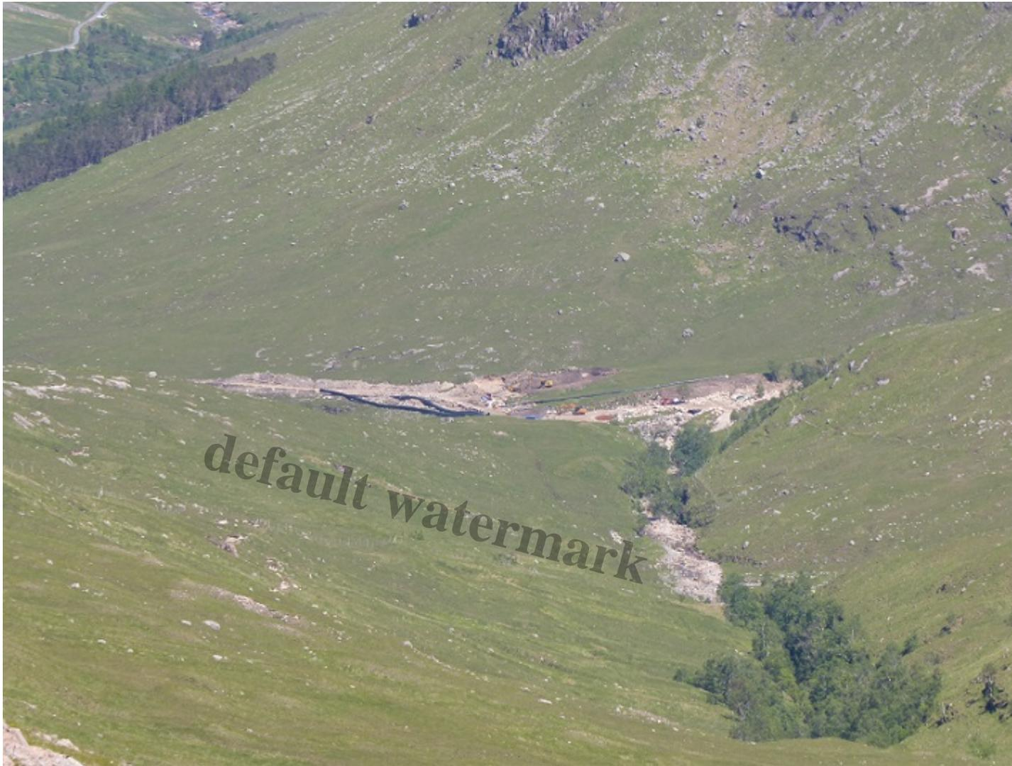
The Allt Chaorainn intake – note the vehicles and pipeline yet to be buried – and a section of the access track constructed through granite slabs viewed from the slopes of Beinn Ceitlein
