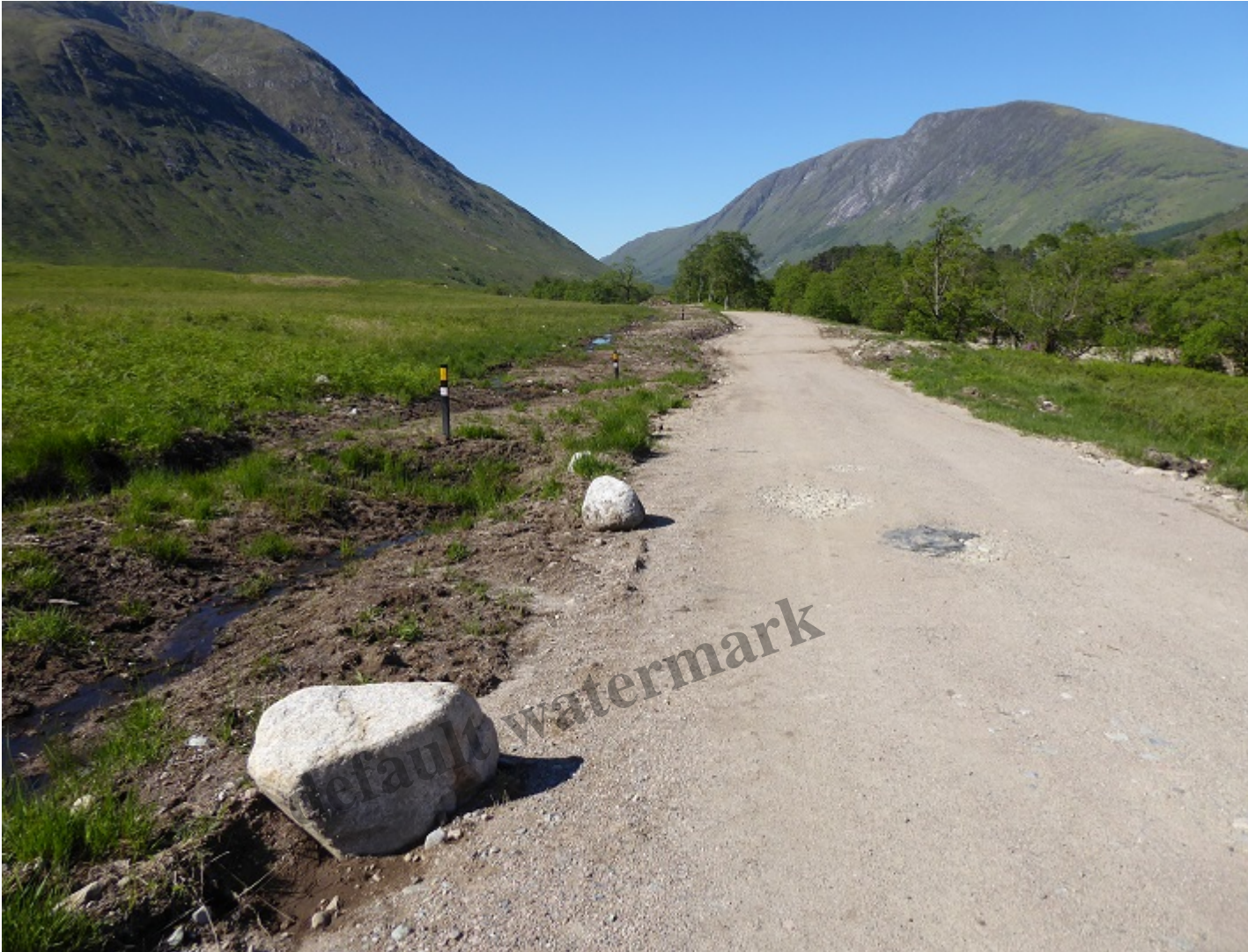
The new track to the Allt Mheuran power house (1 in top photo), in part “floated” over peat bog. The plastic poles on the left, an intrusion into a once wild landscape, mark a section of under-grounded power line.
