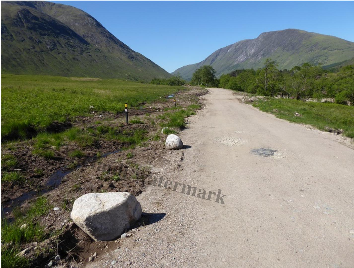
The new track to the Allt Mheuran power house (1 in top photo), in part “floated” over peat bog. The plastic poles on the left, an intrusion into a once wild landscape, mark a section of underground power line.
