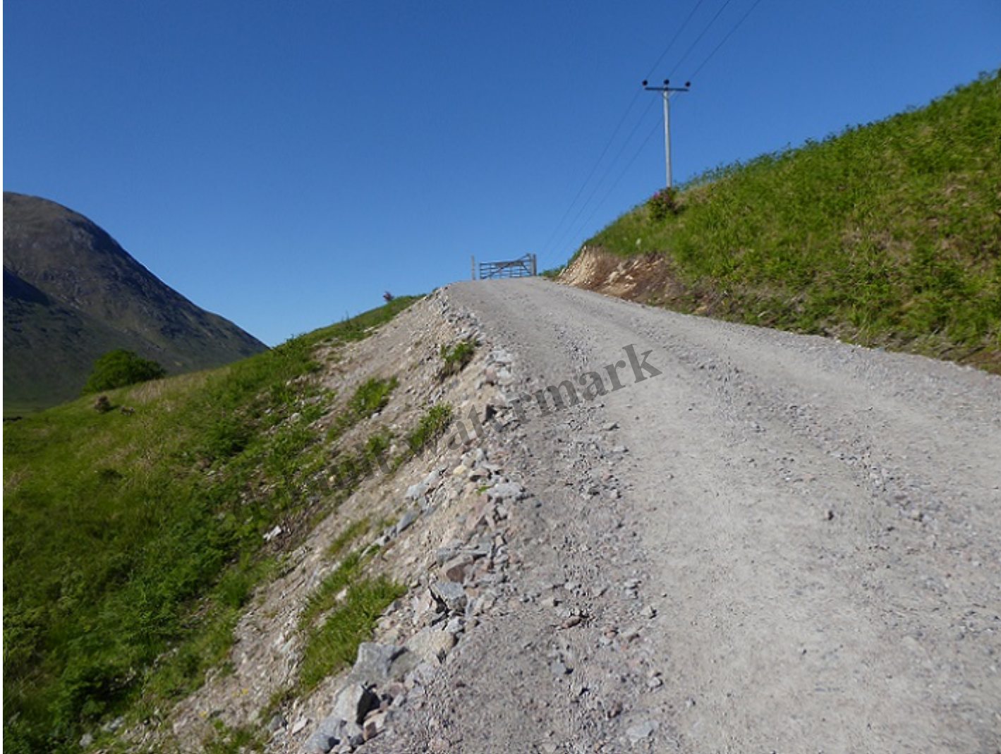
Looking back up to the start of the enlarged access track
