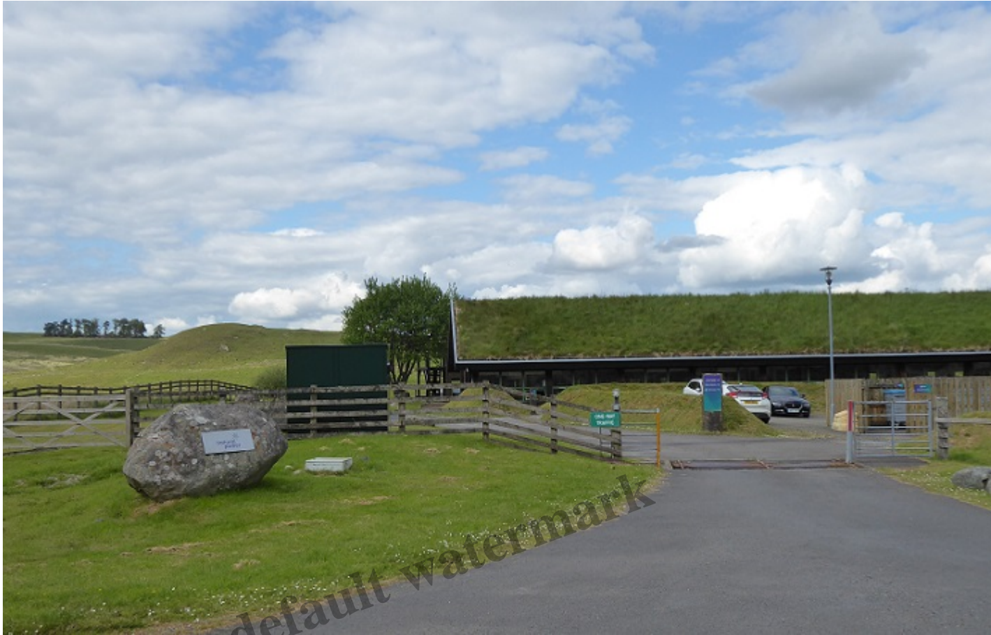
The green headquarters of Natural Power on the Forrest Lodge estate
