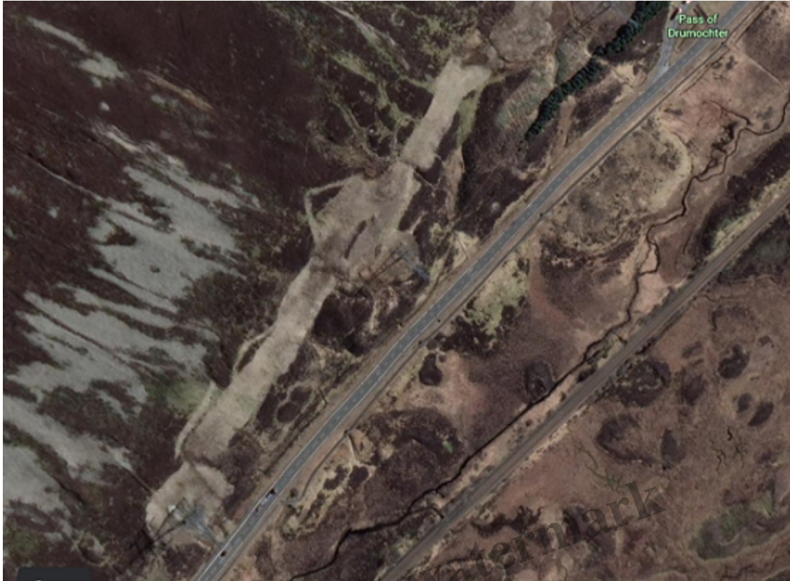
Section of Beaully Denny just south of layby by Drumochter summit. Photo 21/04/21 credit google earth
