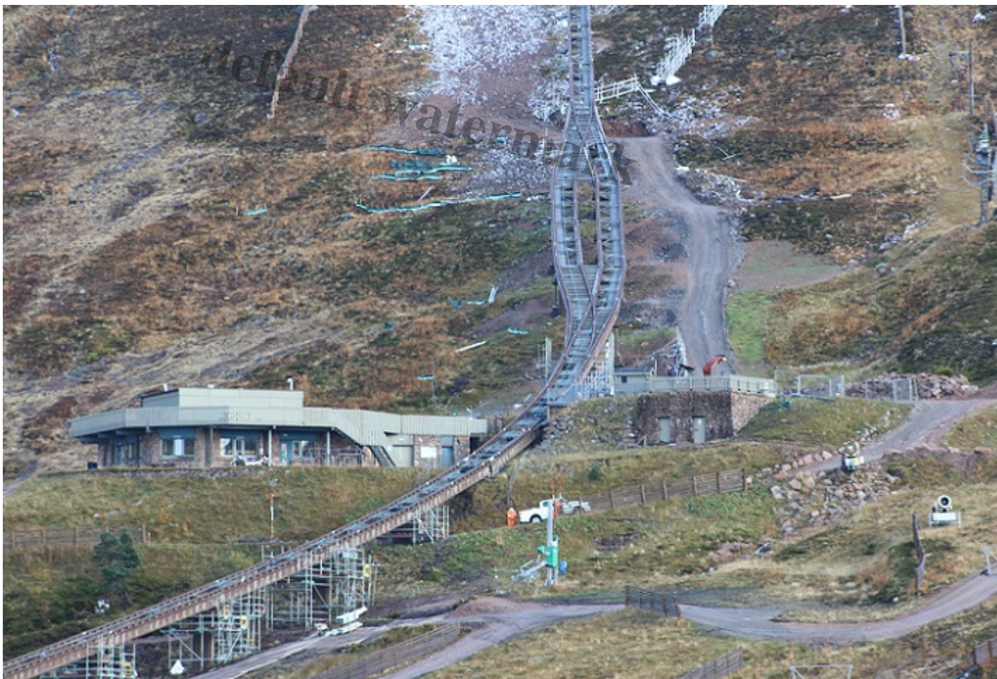
More temporary repair track and restored ground above (on left of funicular). Photo credit Gordon Bulloch 4th November 2021
