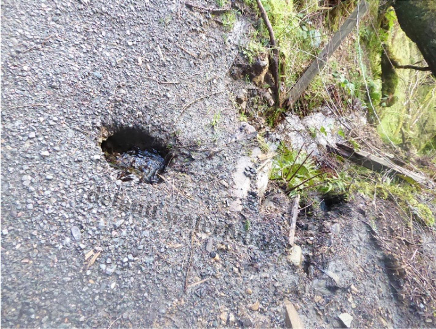
Road surface eroding from below
