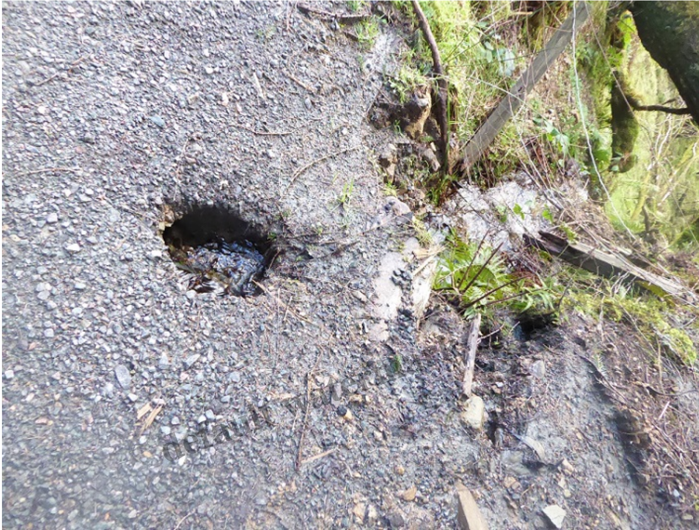
Road surface eroding from below
