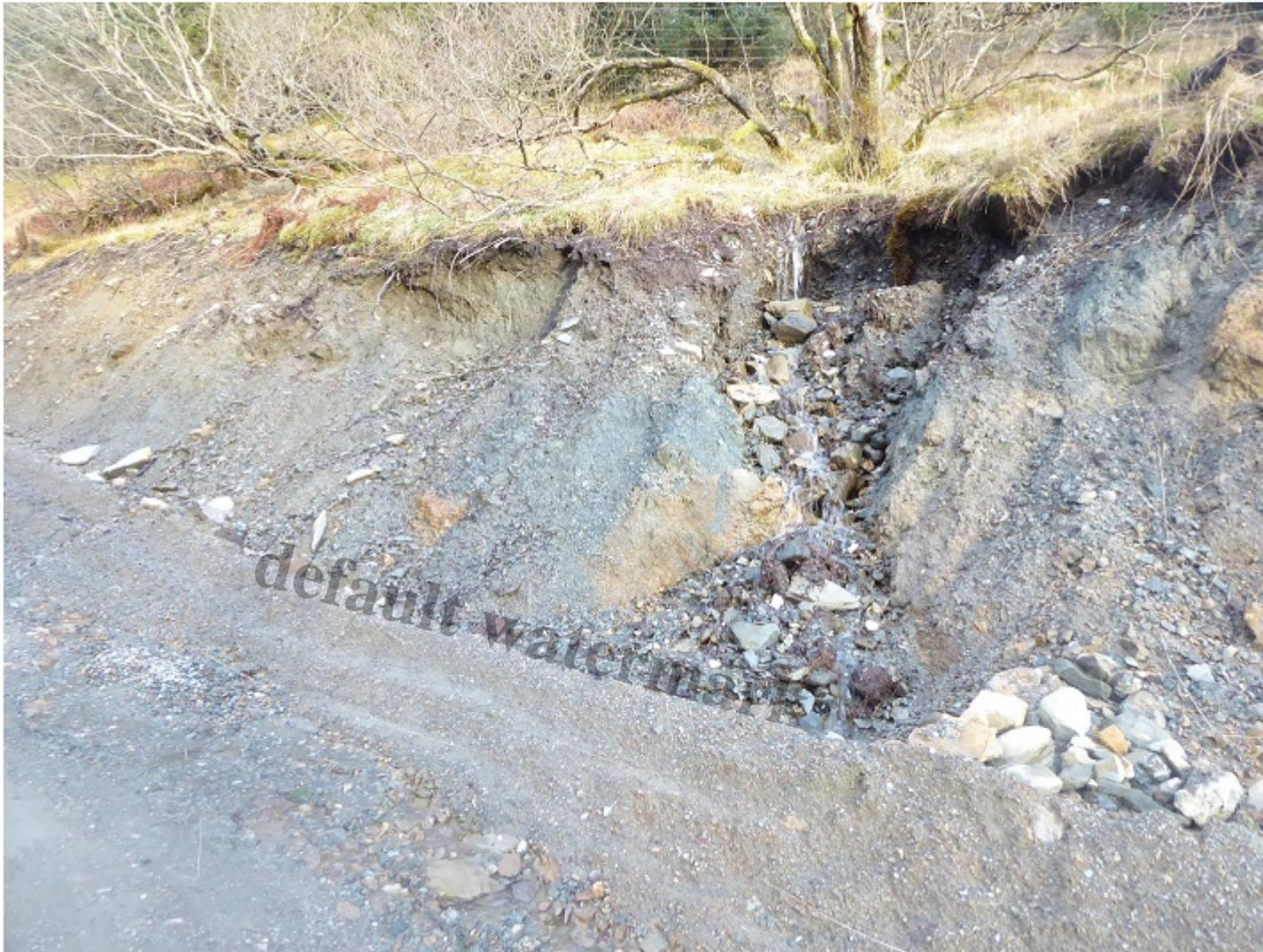
No grading and part of the batter is being actively eroded by water
