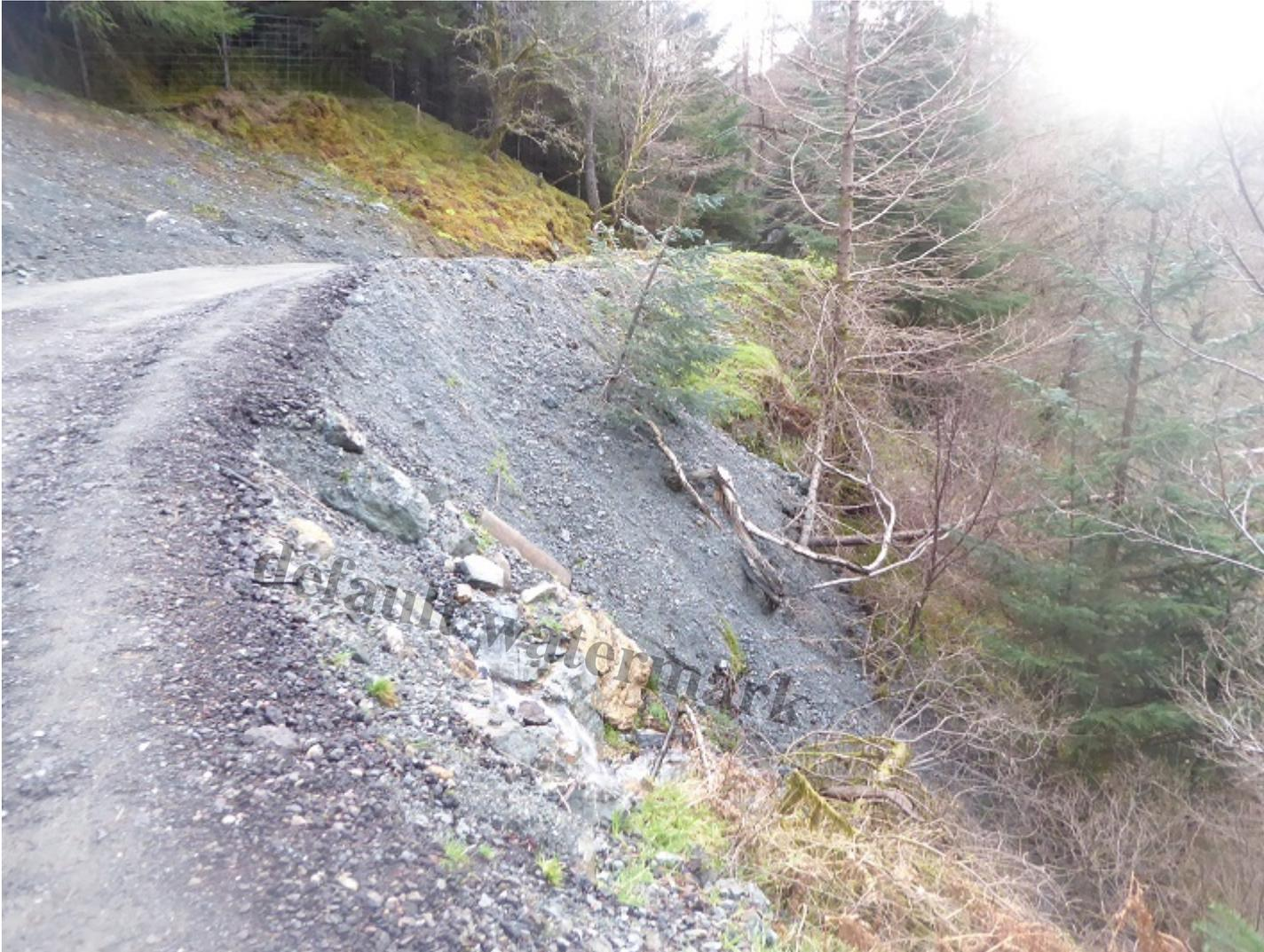
Bare edge of track eroding down towards the burn below - note the old abandoned concrete culvert
