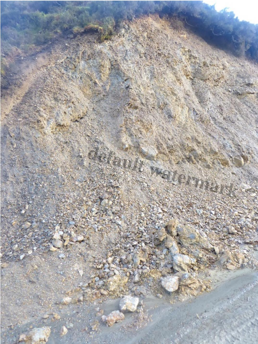
Where possible, the tract from A-B will be extended without cutting new batters into the hillside, but due to the localised topography and terrain, it will not always be practical or viable to do this; therefore small new batters will need to be formed where the track is to be widened by 0.5-1m.
