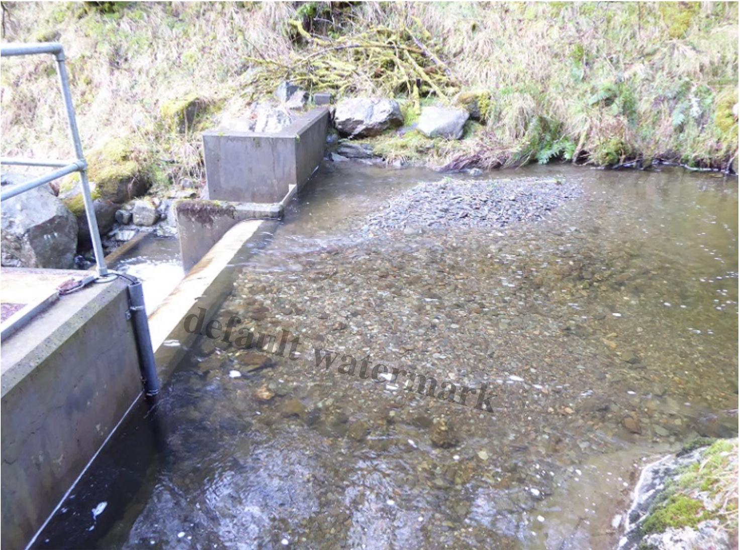
While run of river hydro intakes do gradually fill in over time, it appears that the Ardchullarie intake may be filling up quicker than one might normally expect.
