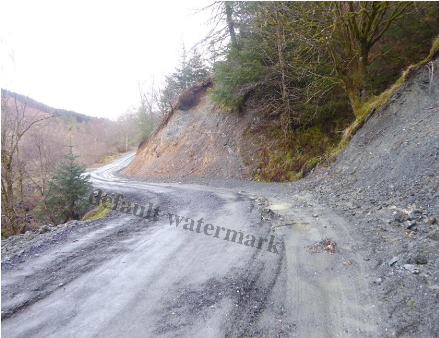
The grassy patch, that helped hold the slope together has shrunk, the detritus from the landslip removed and the cutting scraped back further. Small rocks have continued to erode out of the bank the right.
