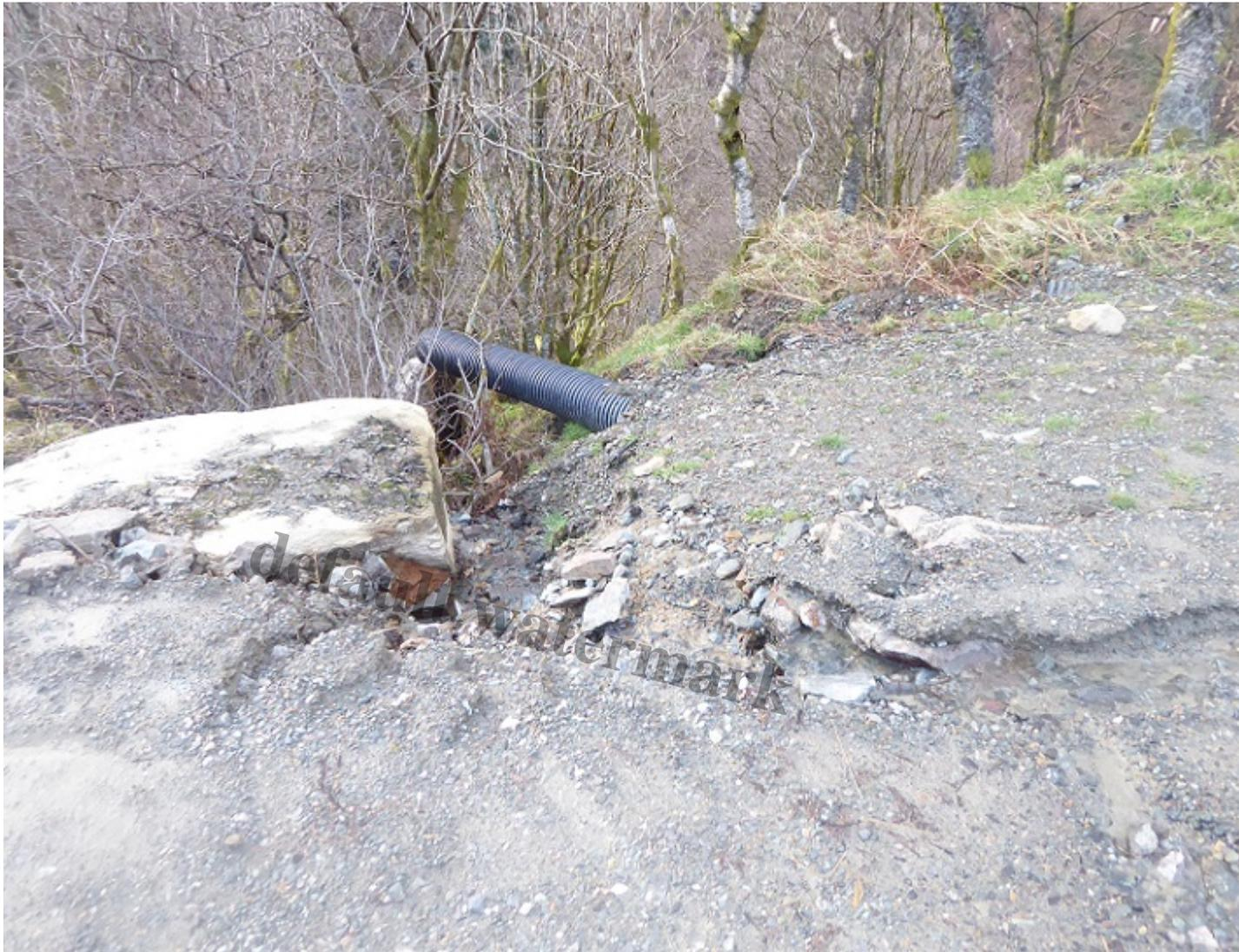
Inconspicuous? Note how the water flowing down the road has taken silt with it add that to the Ardchullarie burn
