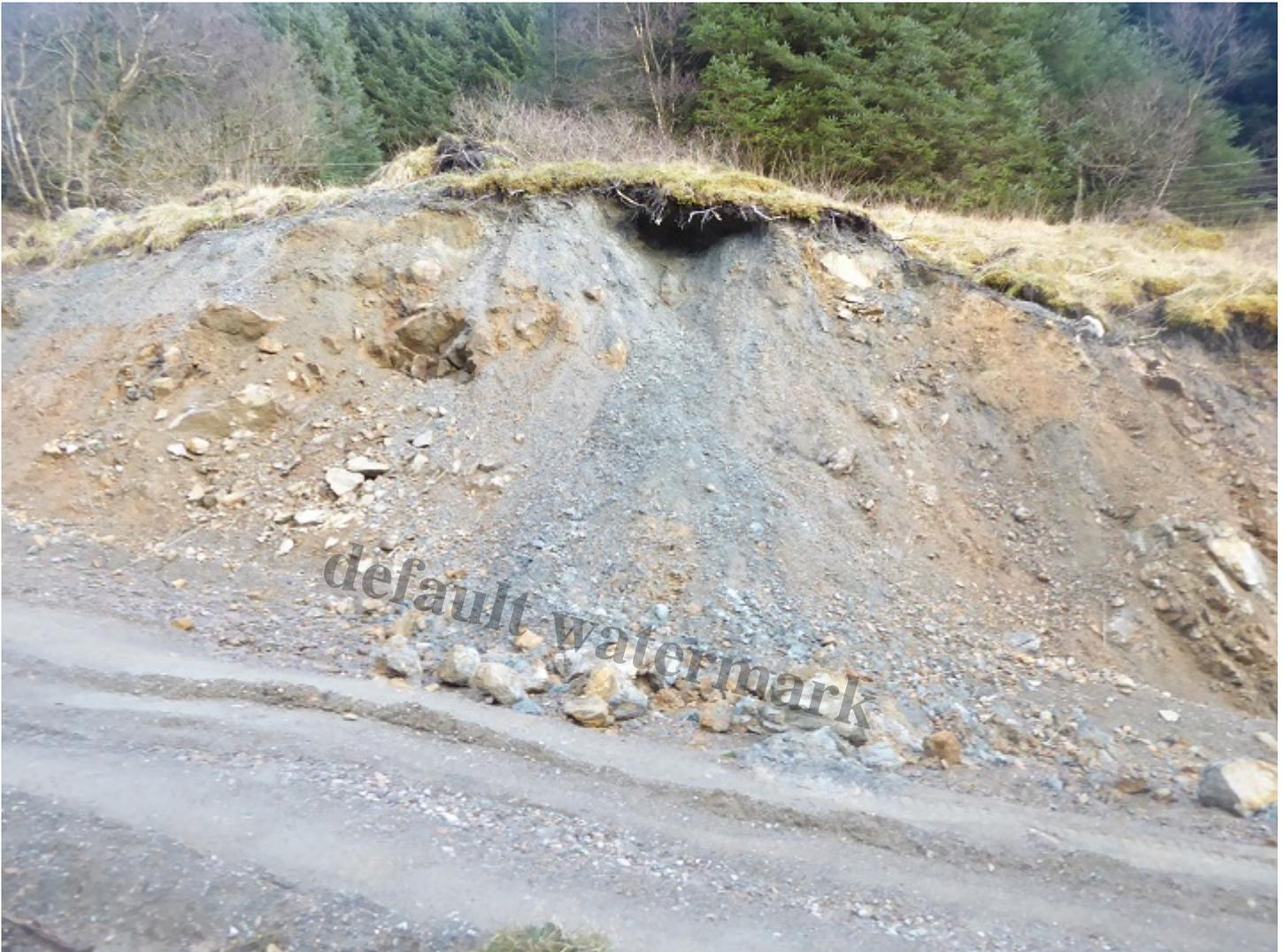
• *Batters are proposed to be graded to a stable angle and feather into the original slope profile*•
