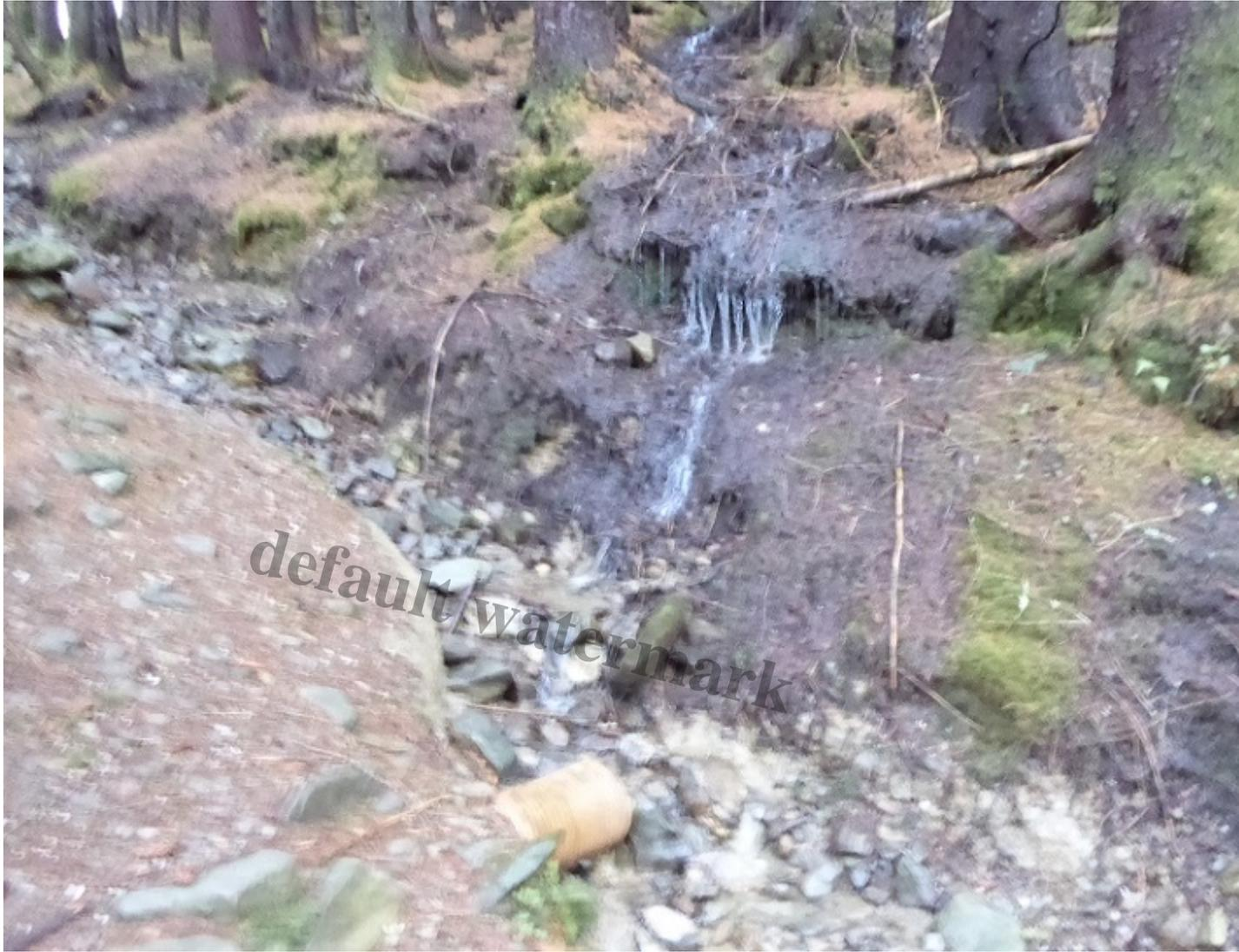
The culvert was presumably intended to take the water flowing between the trees. That water is now eroding the path below. Note too the large trench that has eroded at the side of the path above.
