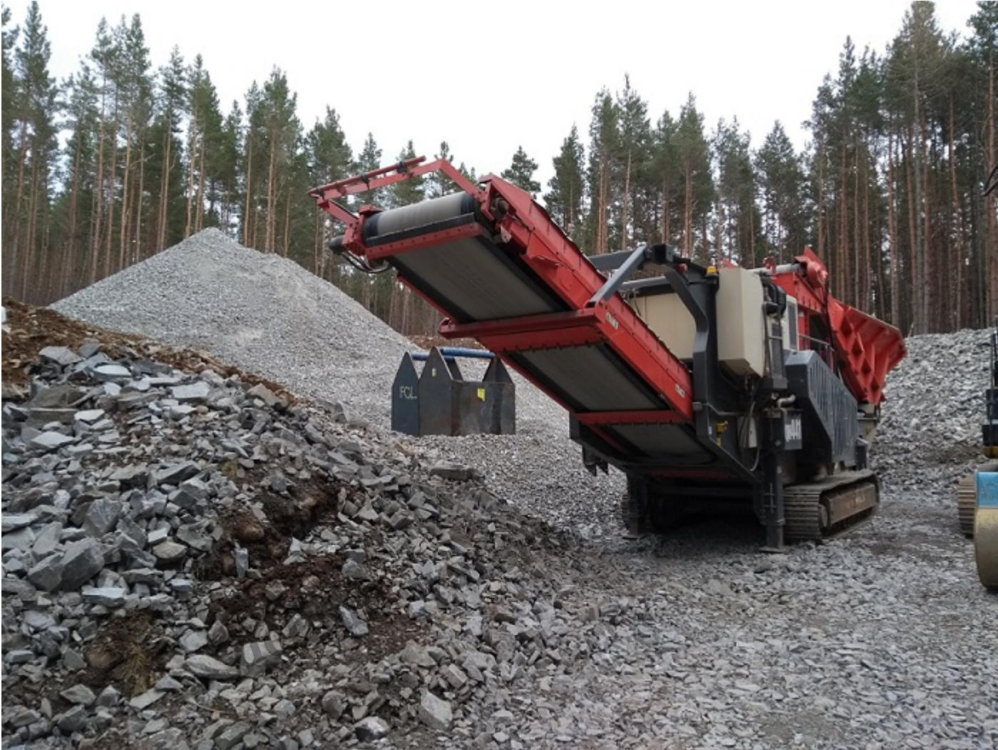
The Borrow Pit 20th March 2020. Photo credit Dick Webster.
