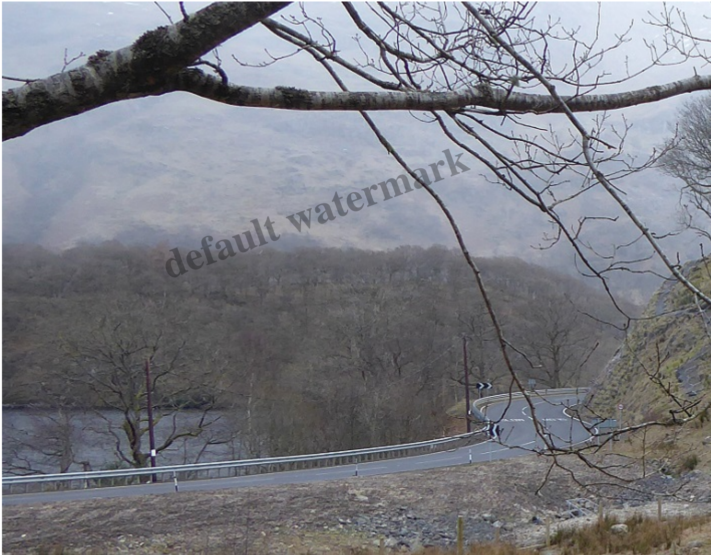
The upgrade viewed from Pulpit Rock soon after completion: sharp bends and no cycle path/walkway along most of it (there is a section of disconnected walkway).
