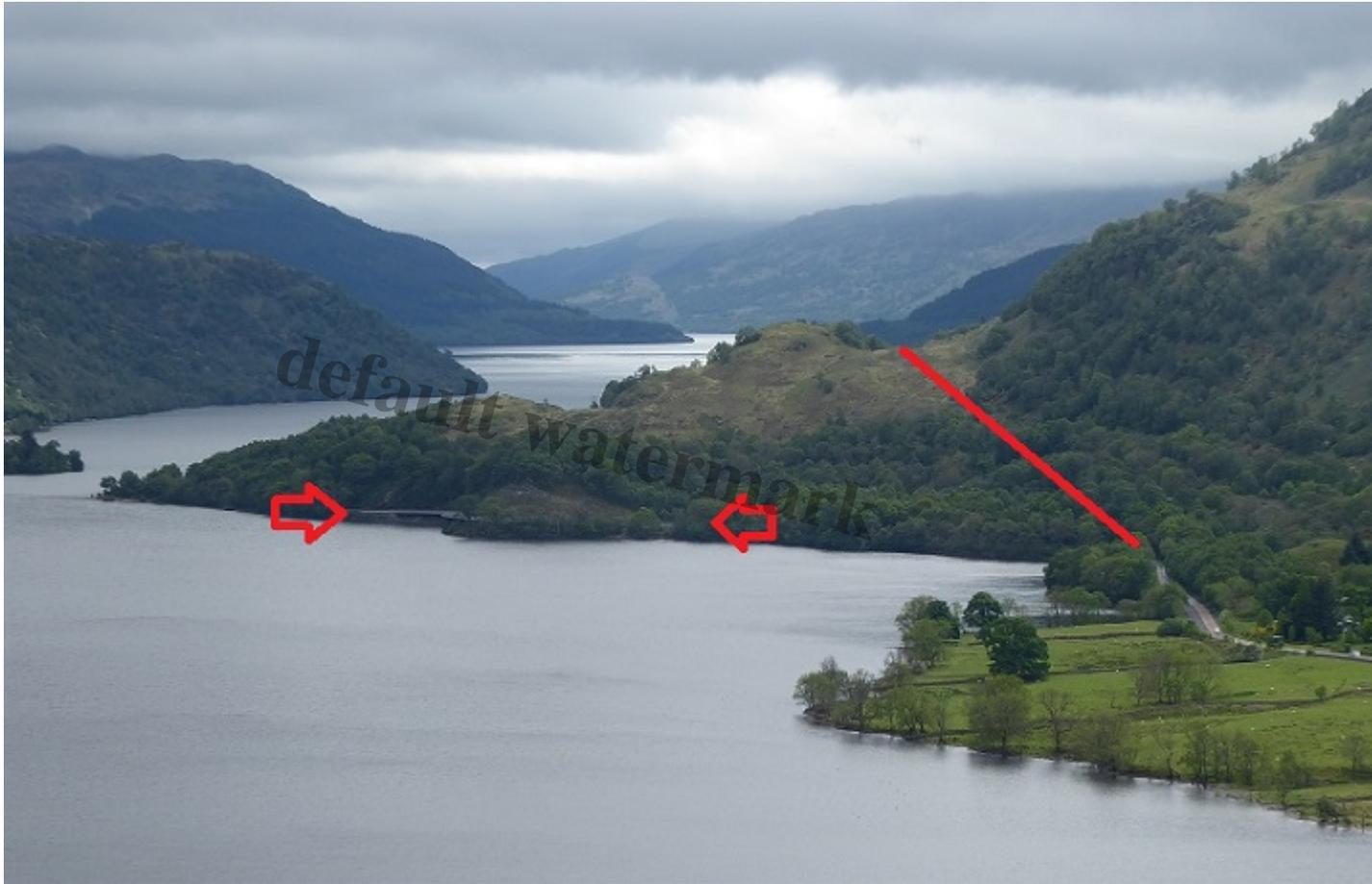
Arrows point to section of A82 widened by Pulpit Rock, the red line the potential for a more direct route whether through a tunnel or higher level
