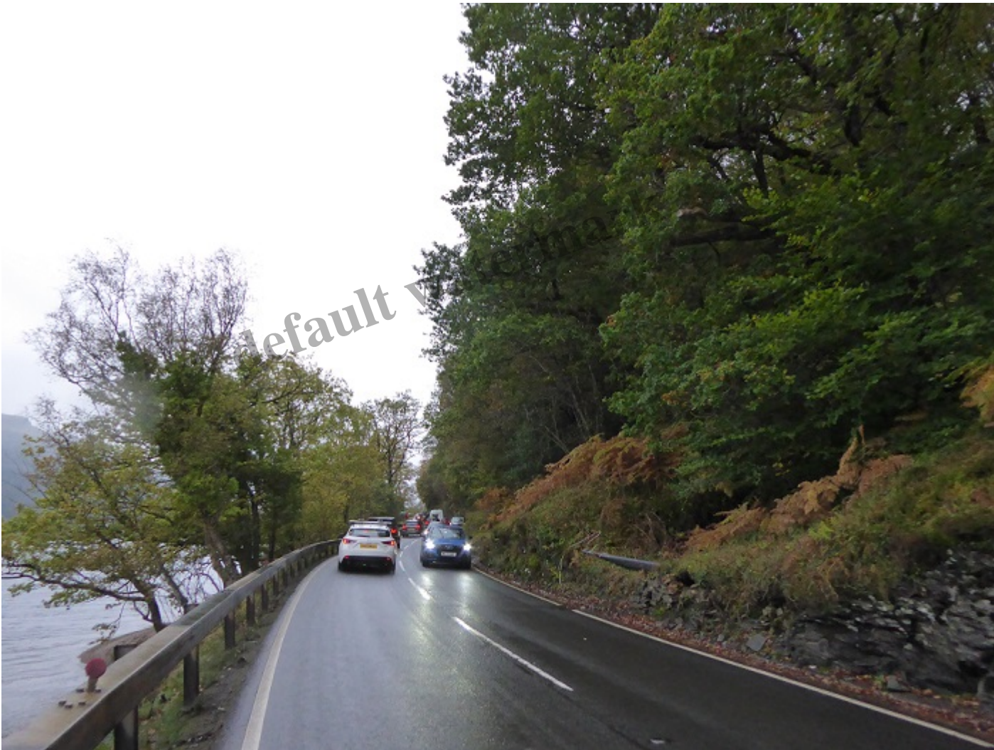
The challenges of widening the road in sections like this AND incorporating a cycle path 2.5m wide AND a verge 2.5m wide as per modern standards are considerable
