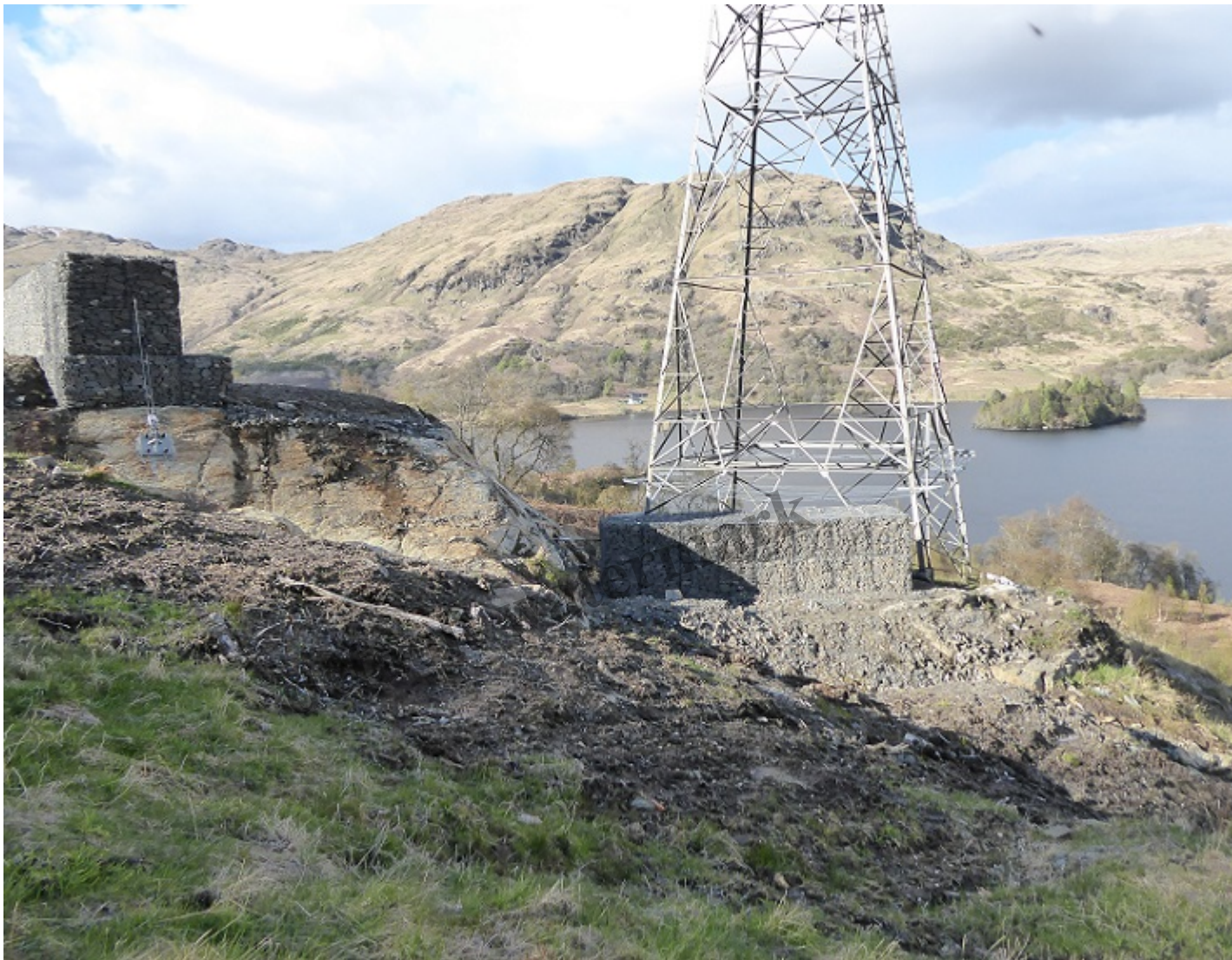
New landslip defences above the pylon. The size of the walls is an indication of the severity of the landslide risks around Loch Katrine. Photo credit author.
