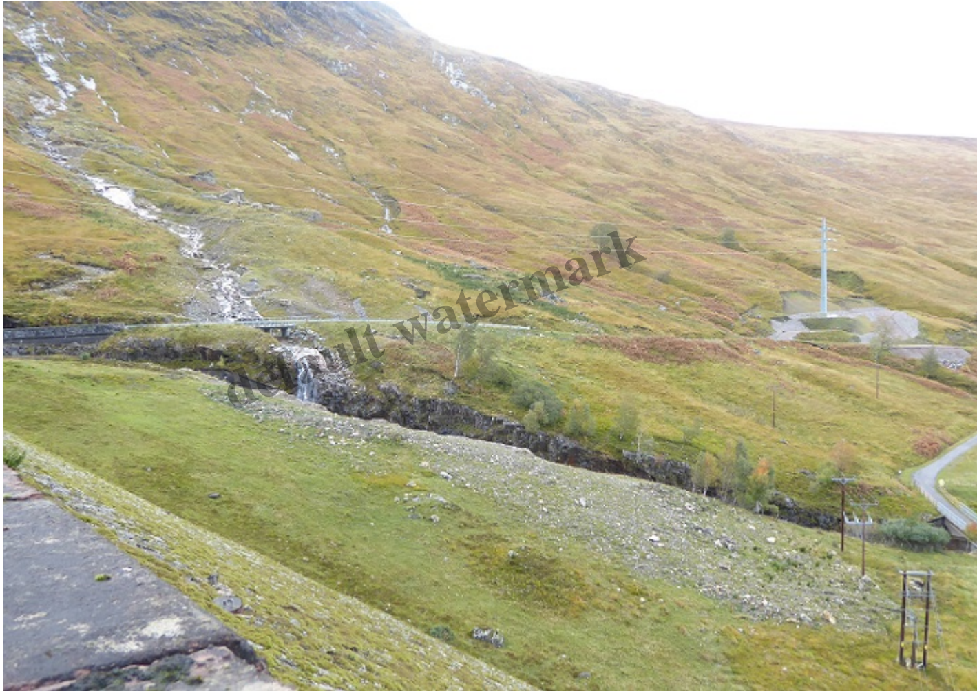
Landslide debris below the Loch Quoich spillway viewed from the dam and easternmost of the 3 new pylons . Note the landscape impact and damage caused by the construction.
