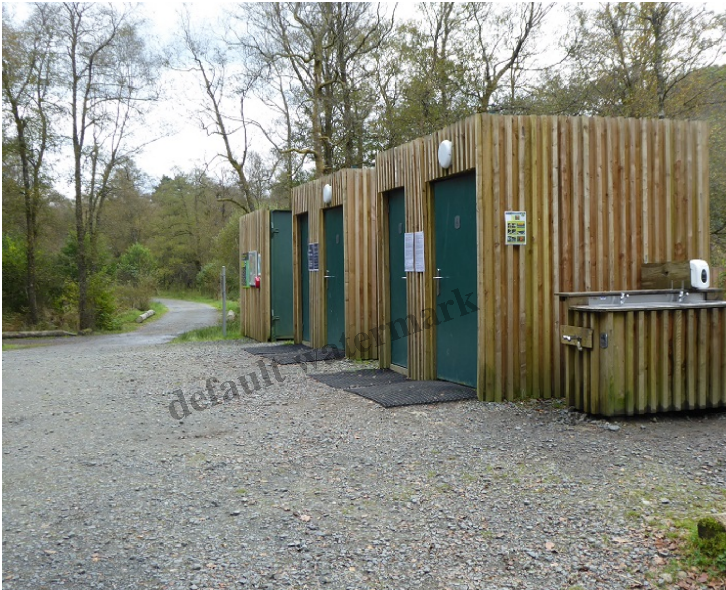
The toilets at Loch Chon, a wasted resource
