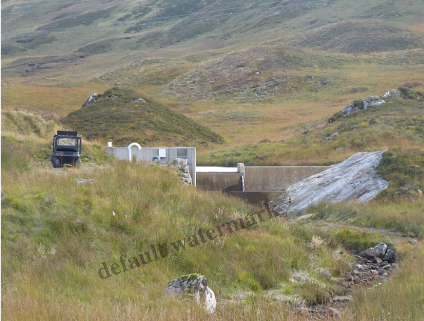
Second hydro intake, with pool behind and half empty burn below. Photo credit Louise Brimelow.
