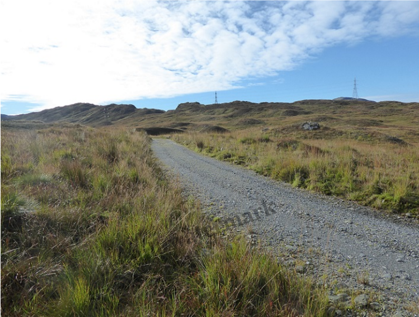
A section of the horizontal section of the hydro track below the intakes. The wheel marks show it is far broader than was needed for vehicles to access the site. Photo credit Louise Brimelow.
