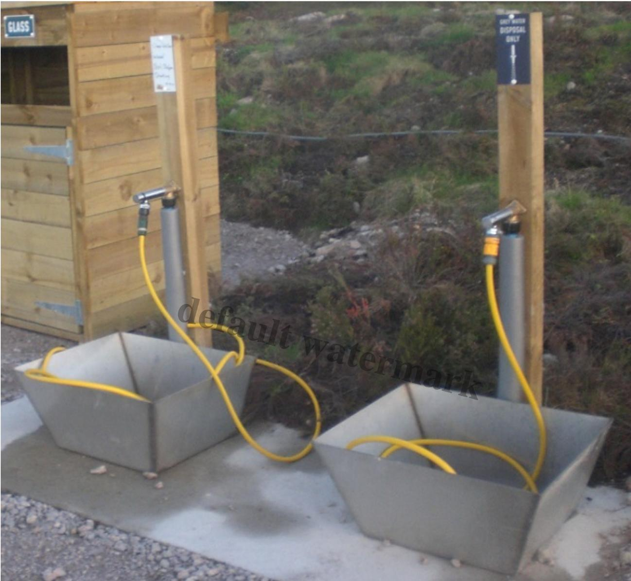
Nothing however has yet been done to separate the drinking water (left) from the grey water disposal point, although its good to see the drinking water now appears to have been tested and the sign (visible on the left hand tap) removed:
