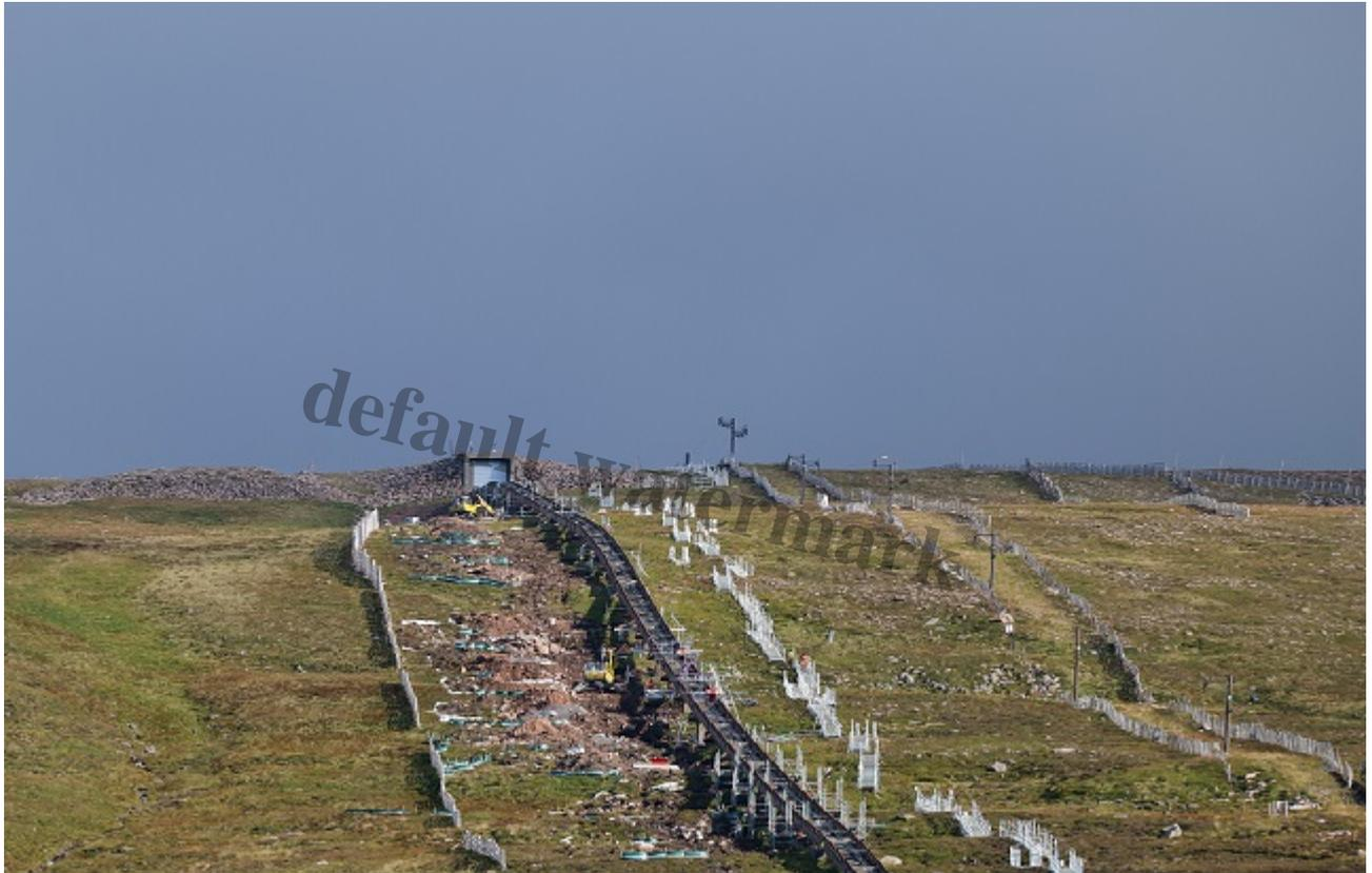
Repairs on upper part of funicular mid-September. Note the numerous blue silt traps across the hillside, an indication that spoil is being washed down the hillside. Photo credit Parkswatch reader.
