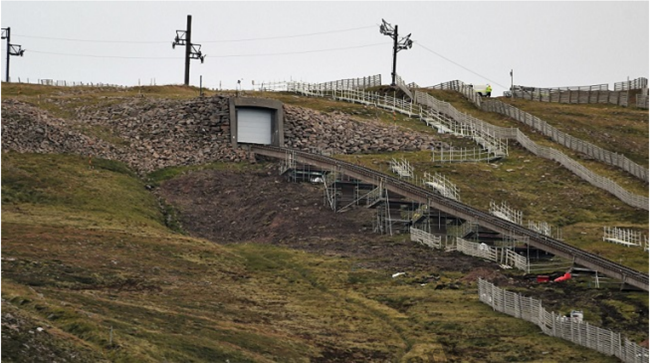
“Restored” ground below the tunnel showing the extent of the tunnel and little evidence of turves having been saved and replaced as required by the planning consent. Photo credit George Paton September 2021.
