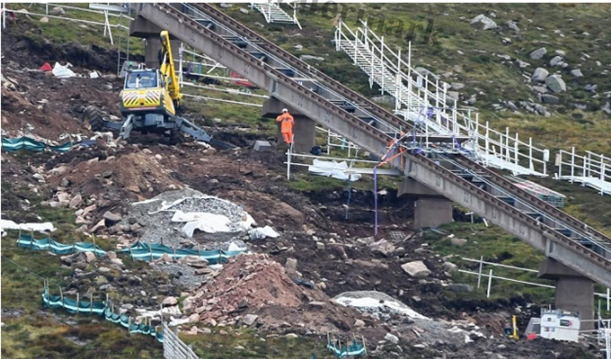
The sheer amount of the earthworks and imported materials provides evidence that the repairs are significantly greater than originally planned. Photo credit George Paton September 2021
