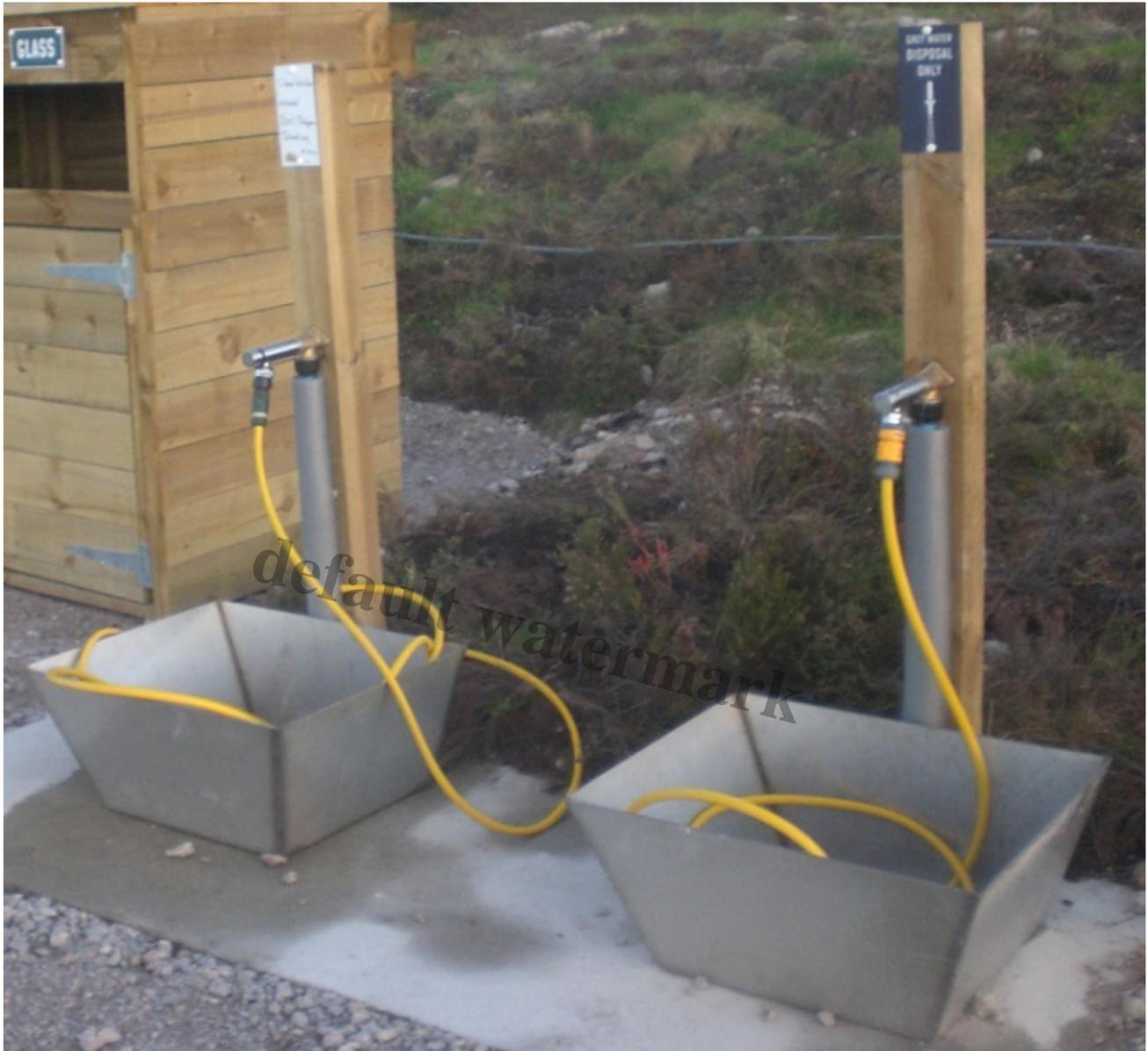
The 'clean' water facility on the left, the grey water disposal facility on right
