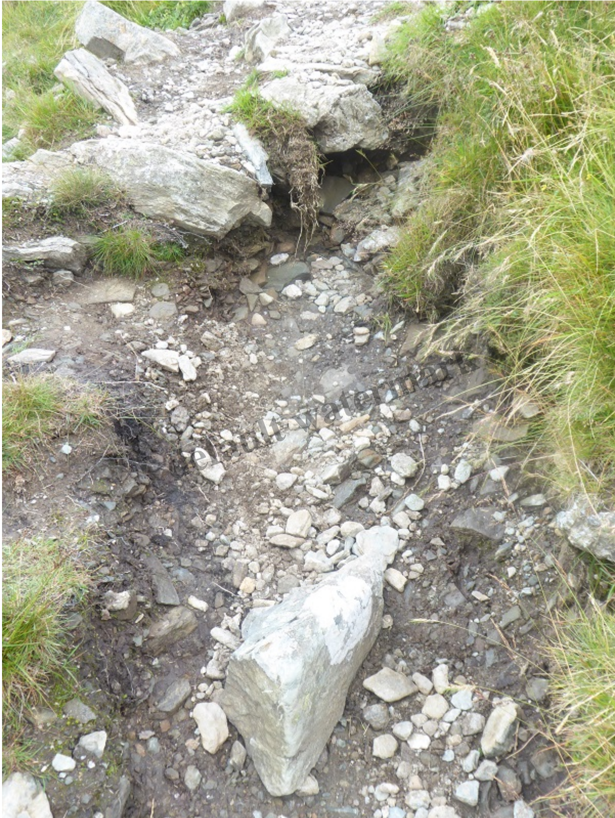
Note how the boulder in the foreground, which once formed a step, has been eroded out of the path.
