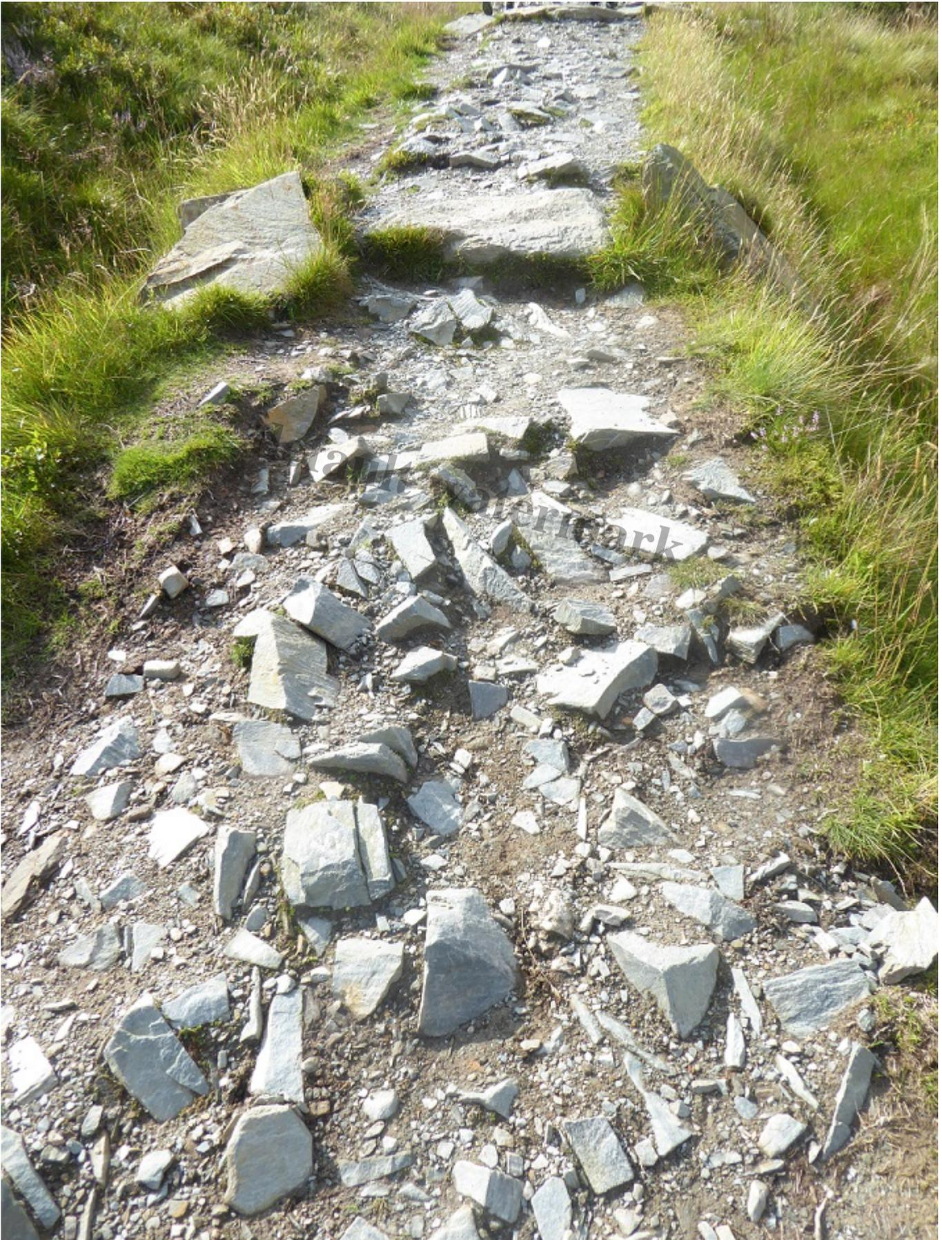
But there are also slightly steeper sections where the aggregate surface has been washed away. According to the Upland Path standards, if properly designed this shouldn't happen. This has made the path unpleasant to walk on so people have taken to the verges and they are now starting to erode.
