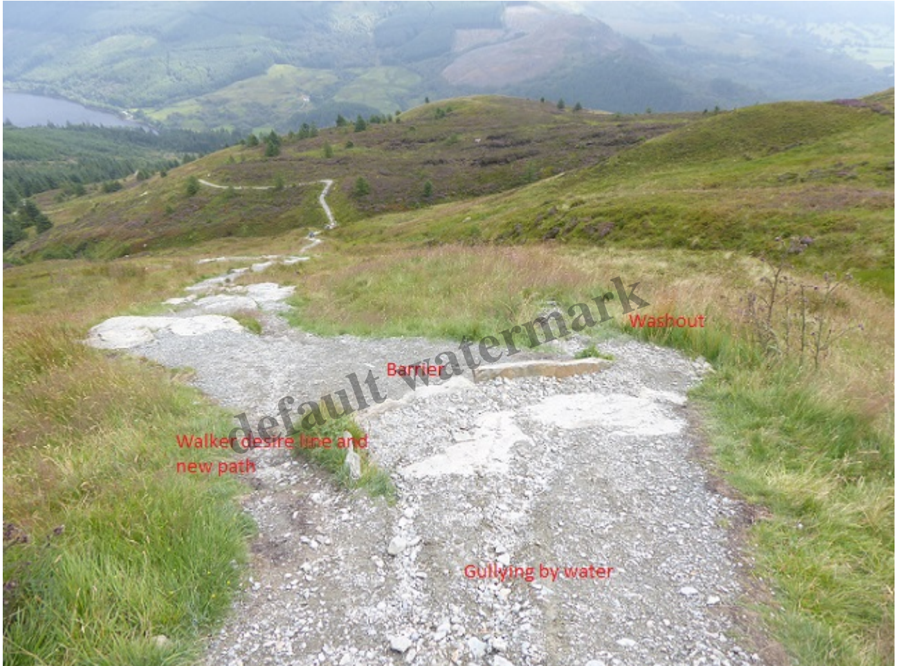
A path gone wrong. A section of the tourist route up Ben Ledi, August 2021, Loch Lubnaig behind
