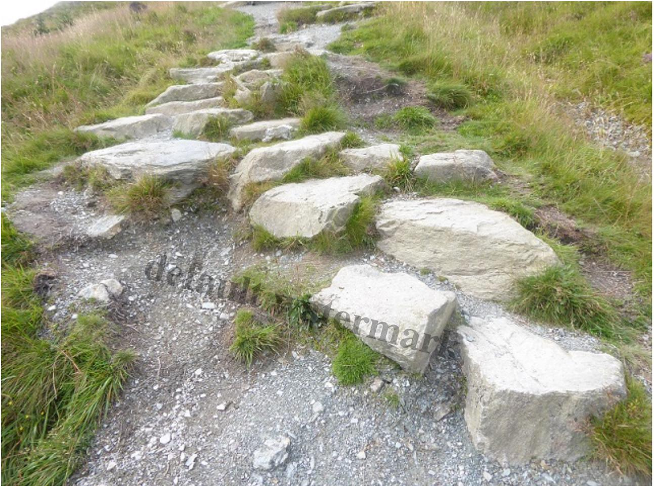
Interpretation. It appears that initially people avoided the steps on the right because they were too high and chose instead to walk directly to the large flat boulder on the left, eroding the ground below which is now starting to gully. As the height required to step onto that boulder increased, people started avoiding them completely, eroding the ground on either side.
