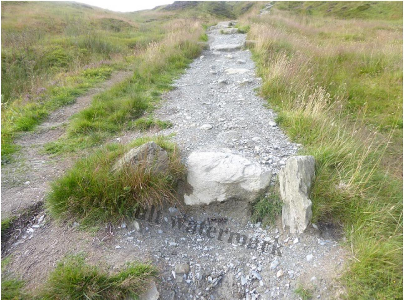
The raised path should have shed water but is now starting to gully and water is being erected over this step eroding it further. How long until it collapses?
