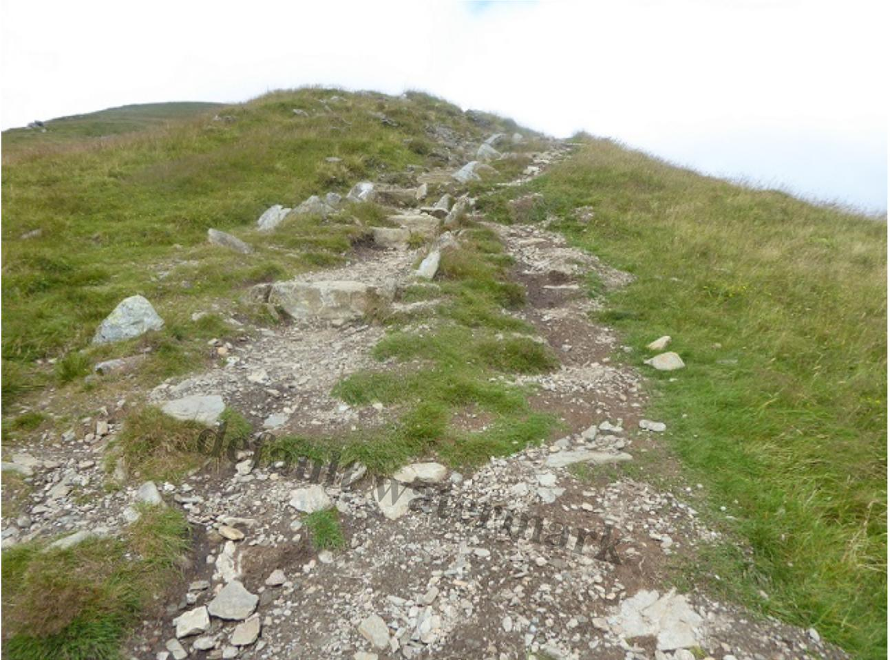
Close up of first steep section showing remnants of former path work. The height of the first step has deterred walkers from accessing the steps above and resulted in the erosion of the ground on the right.
