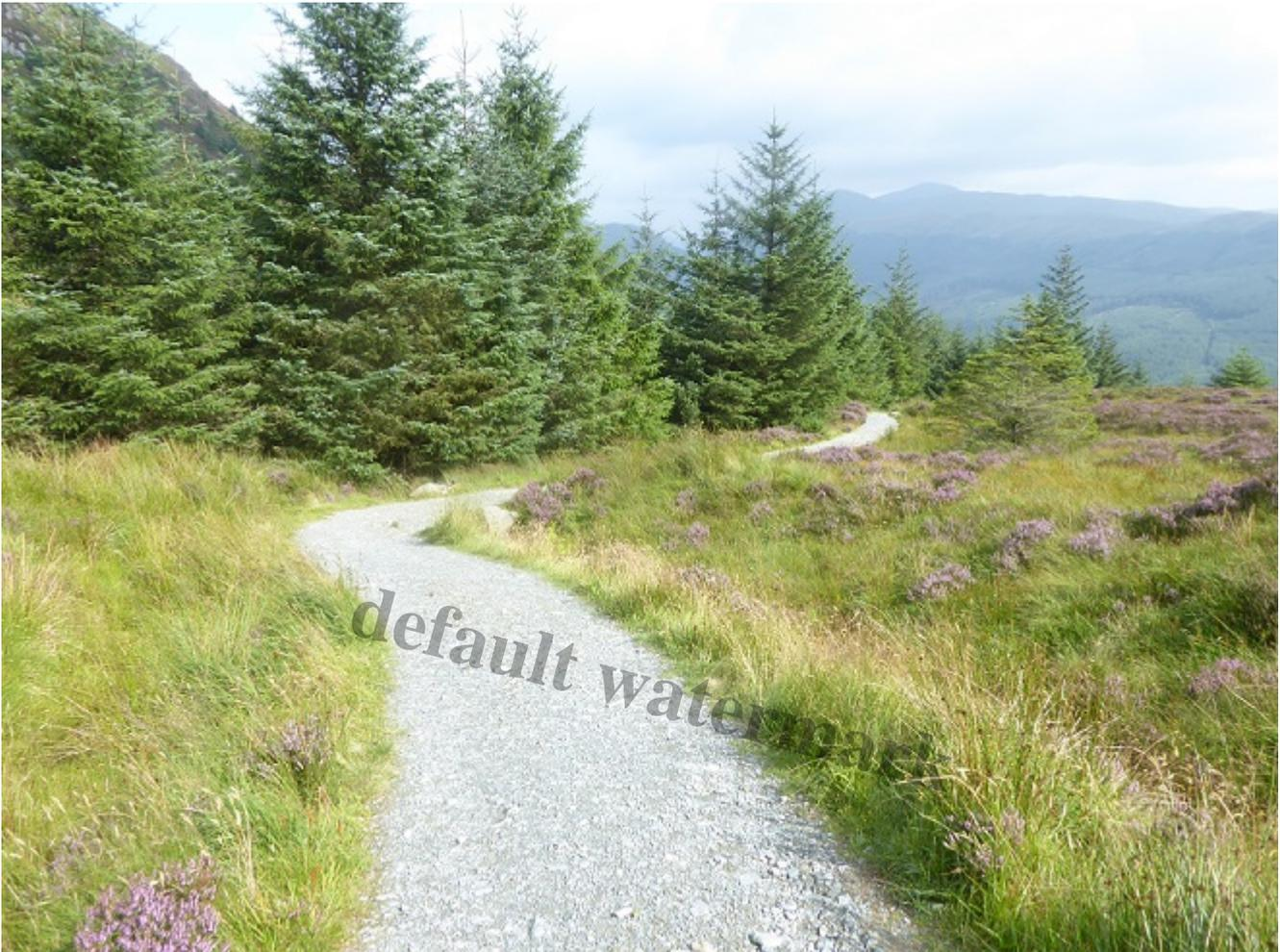
There are similar sections along the main path which have held up well since construction and where the vegetation on either side has regenerated successfully.
