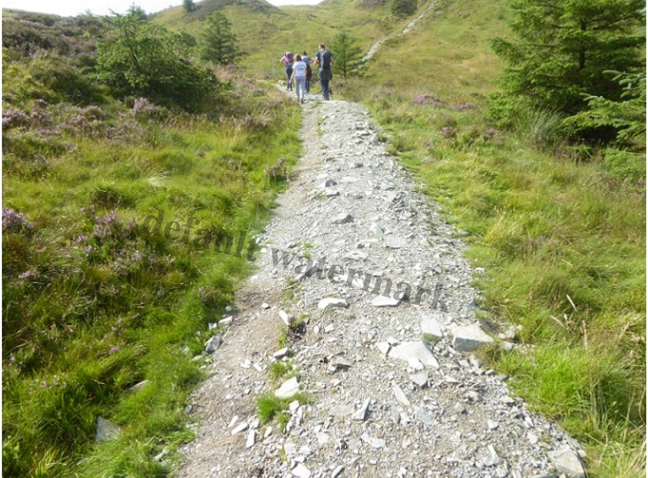
As the raised path has eroded, a new path has been created to the left of it. If this continues the edge of the ditch further to the left could start to collapse
