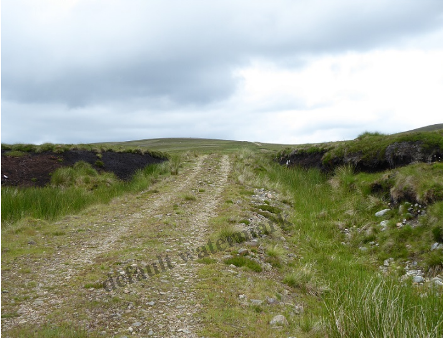
Exposed and eroding areas of peat by the track (location marked by black arrow on map above)
