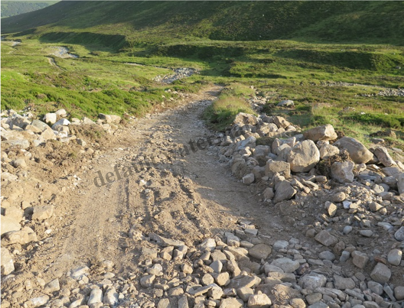
The repaired track by the Allt Fionndrigh
