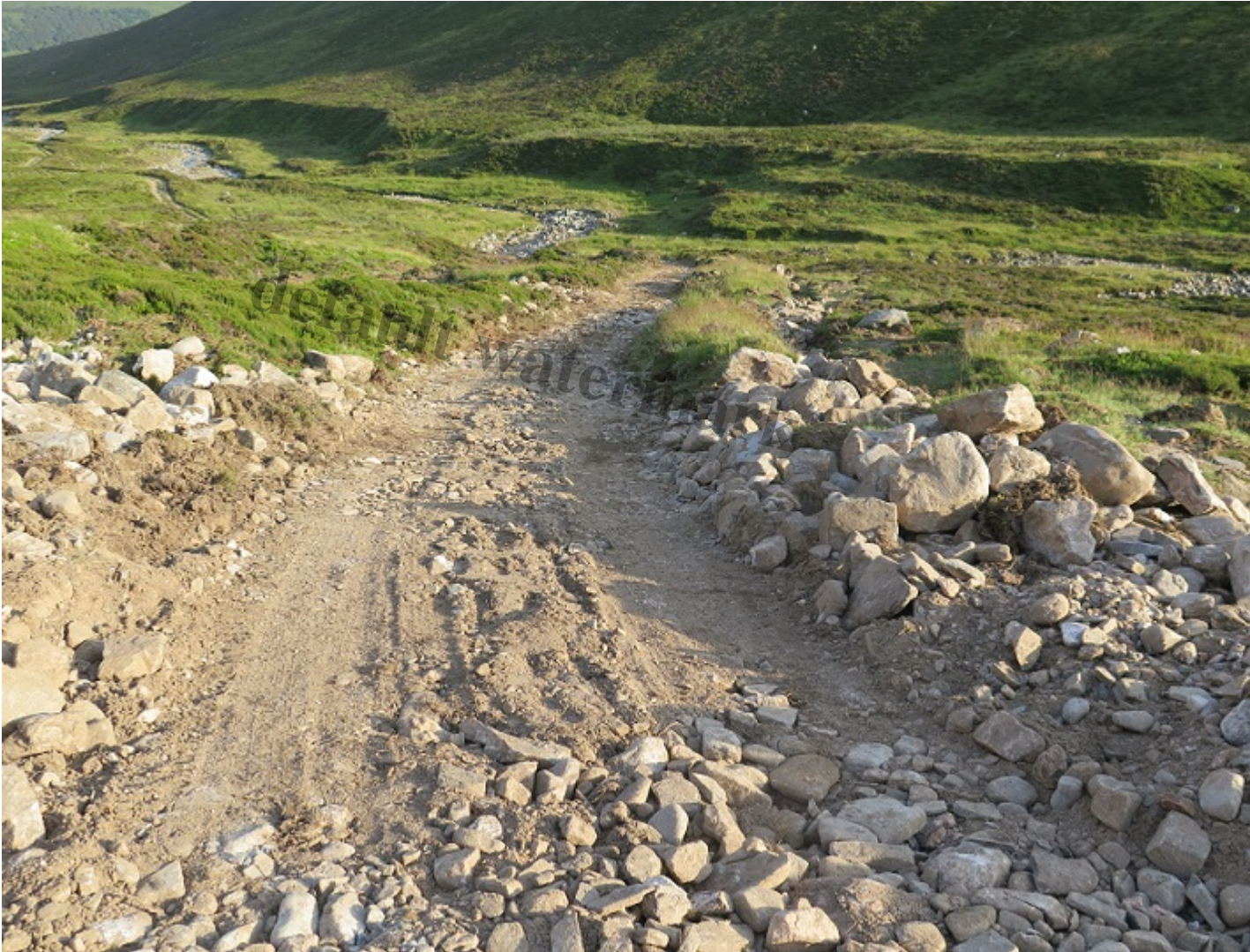
The repaired track by the Allt Fionndrigh
