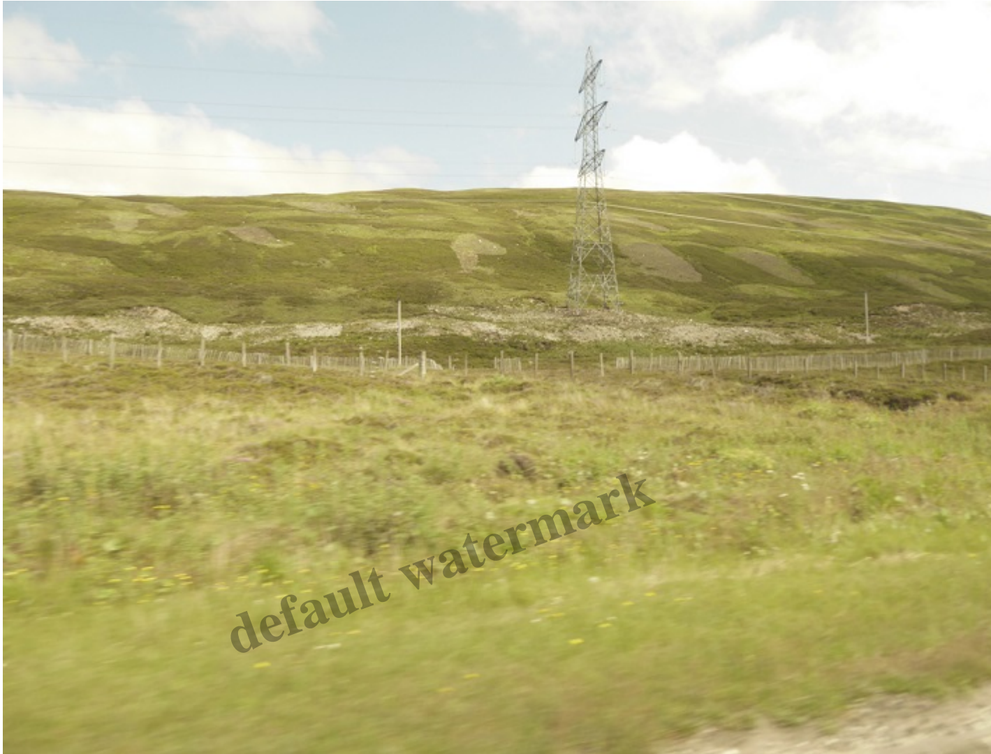
View of section of Beauly Denny access track taken from the car 17th July
