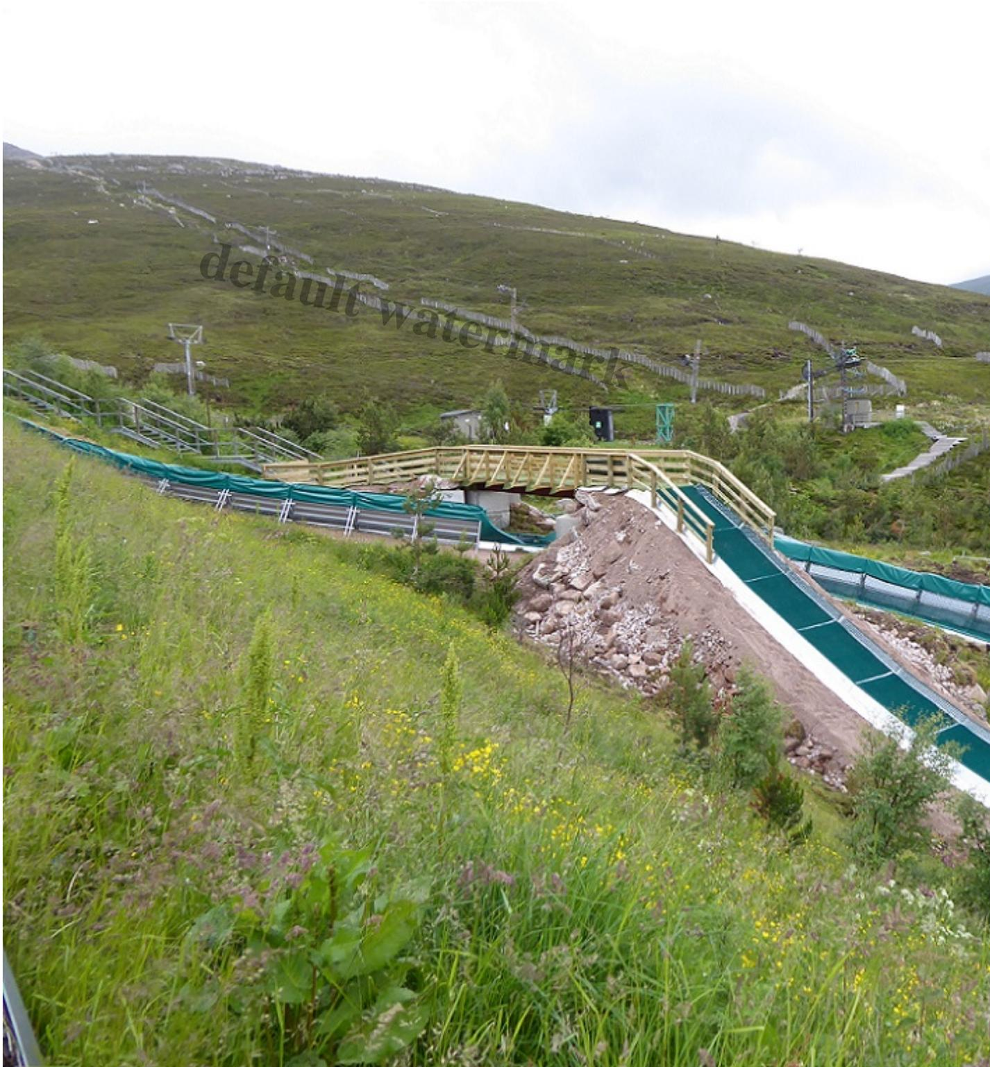
Note how the steep sides of the tube slide by the bridge have already started to erode
