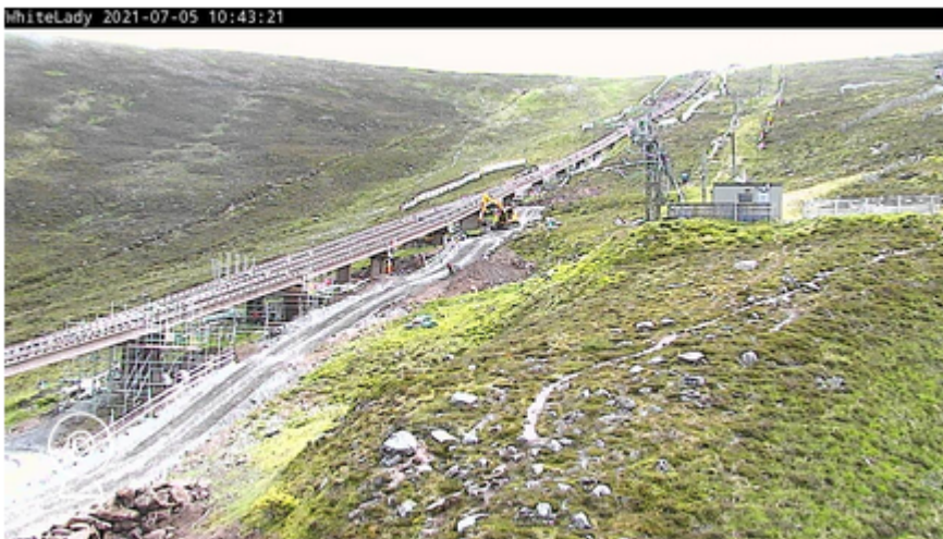
The minor earth works at the passing area earlier today
