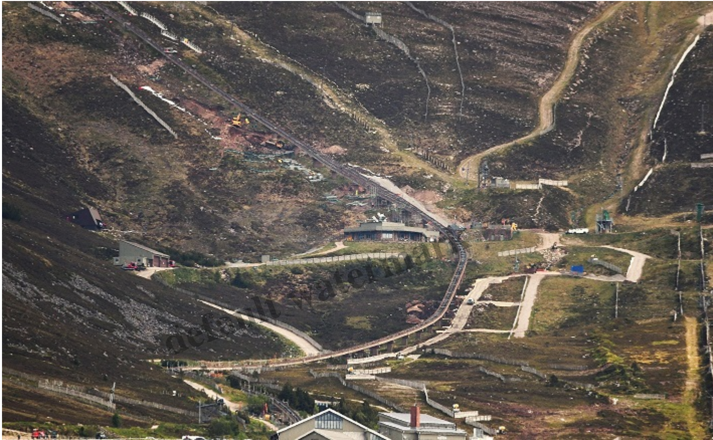
View of middle section of funicular repair work showing temporary access tracks on righthand side of track and extensive earthworks by and above the mid-station. Photo credit George Paton mid-June
