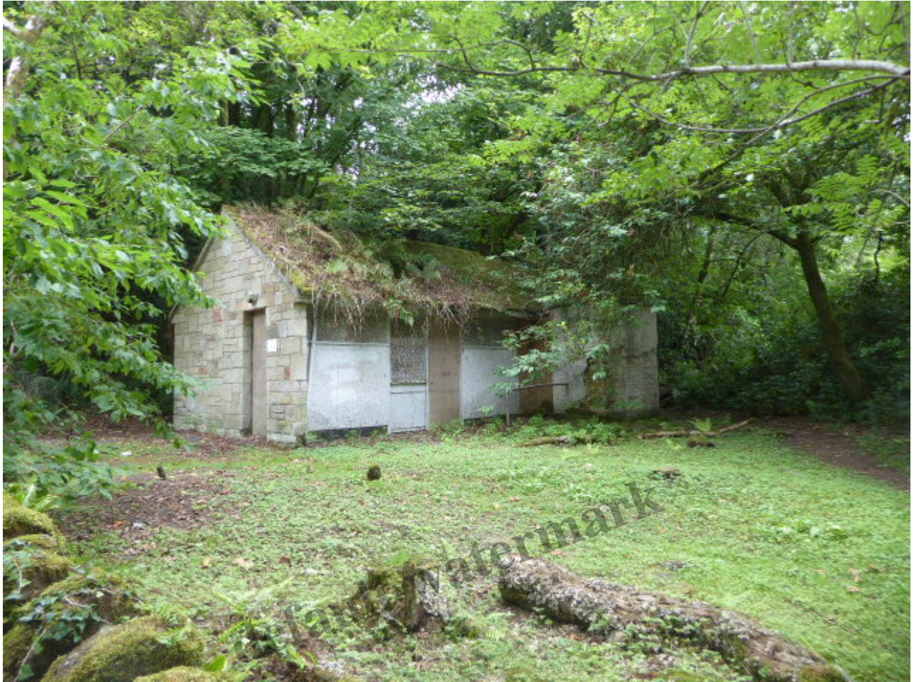
The abandoned public toilets at Duck Bay
