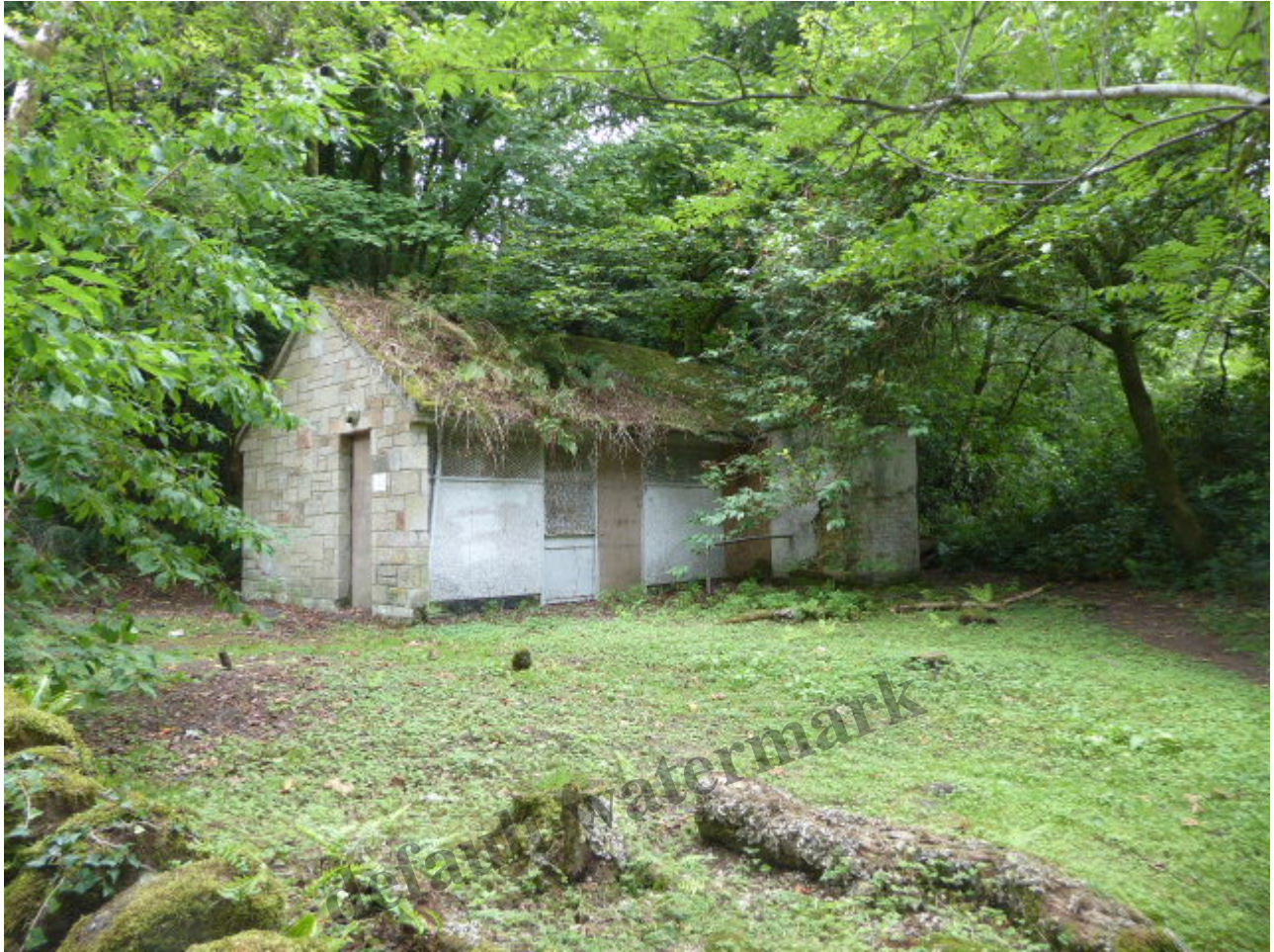
The abandoned public toilets at Duck Bay
