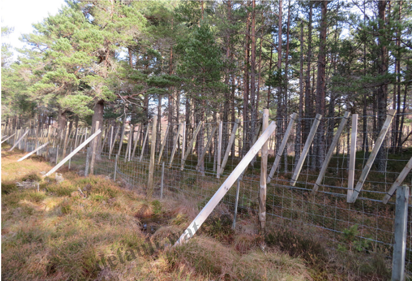
Reinforced fencing with wooden droppers attached with plastic ties. Photo credit parkswatch reader
