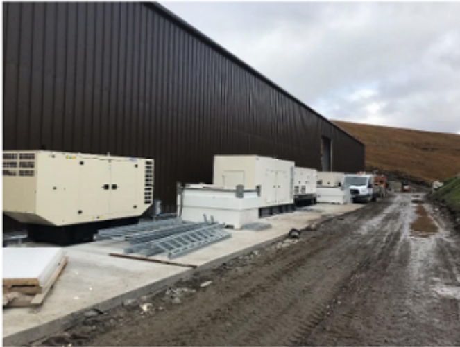
Plant Platform - Front of the processing building the area for Fuel storage tanks and generators (all generators are integrally bunded). Heavy duty protective barrier system to be installed
