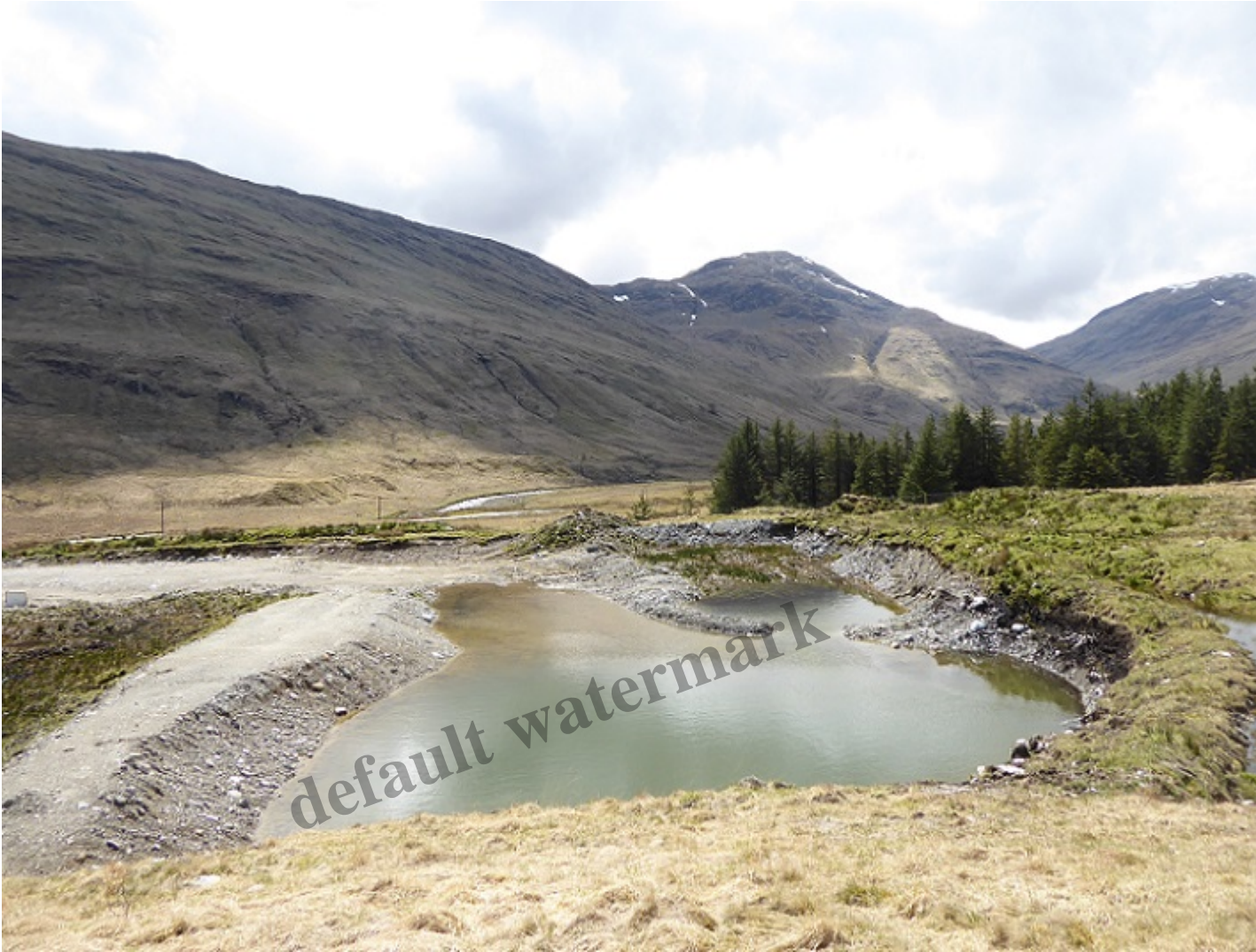
Peat storage cell B, with Ben Oss behind. Note the turves heaped up, one on top of the other, on the far side of what is now a pool.
