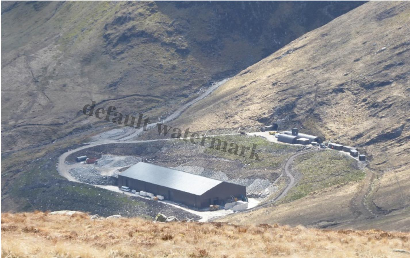
The new platform and bund (embankment) at the Cononish gold mine designed to screen the enormous shed from view. Note how peat has been placed on the bund and the steep slopes surrounding the shed contrary to the original planning consent and how only a proportion of the slopes have been covered with turves (see below).
