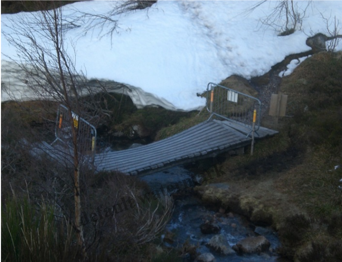
The Bridge over the Allt na Ciste, below the Ciste carpark
