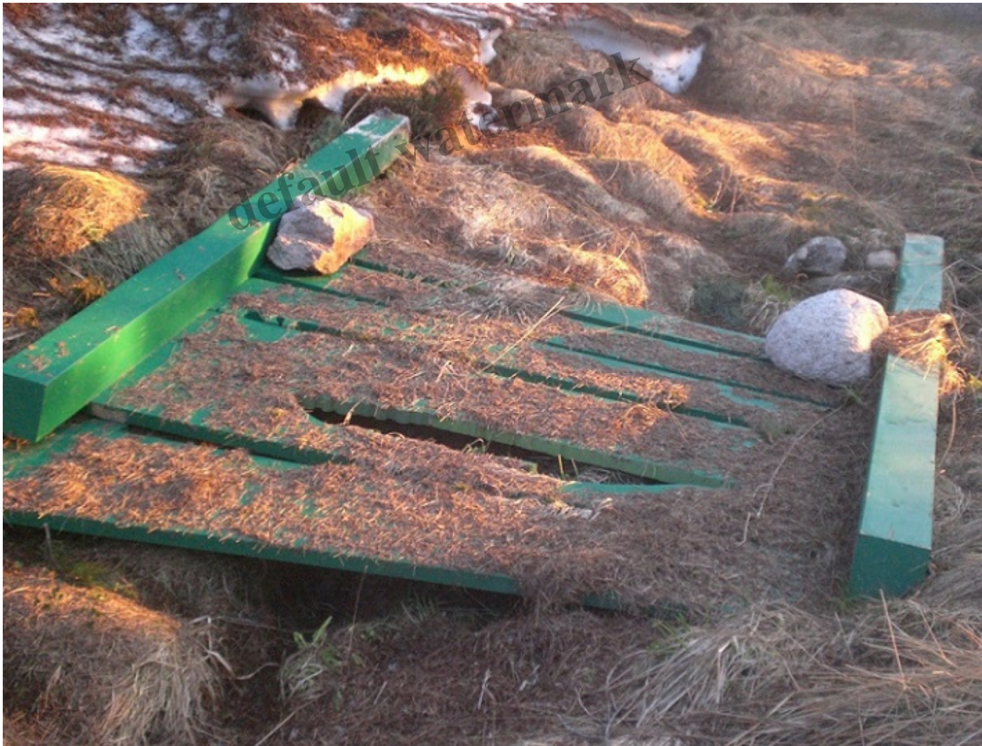
Broken sign which lies on the ground just beyond the Sugar bowl car park
