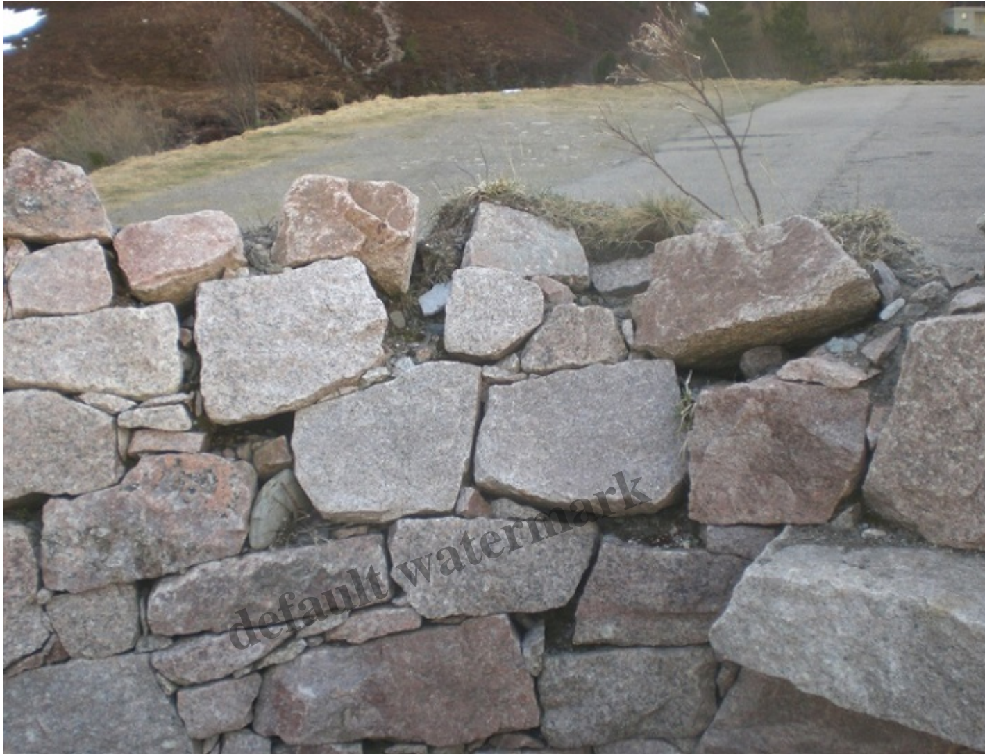
The Ciste car park Grouse Butt.
