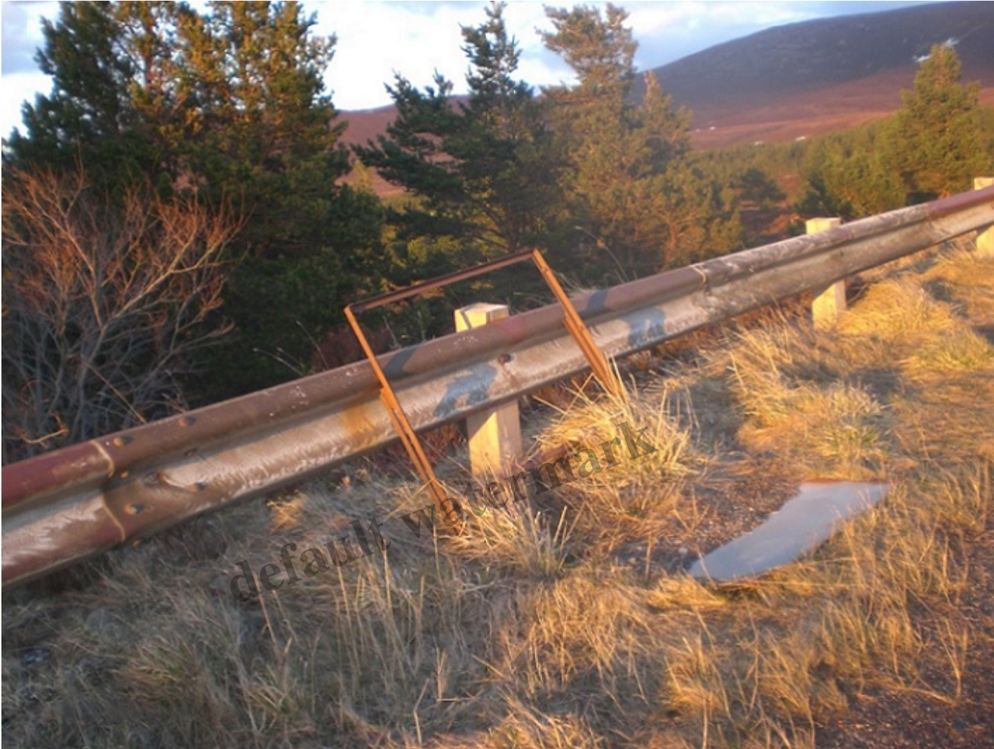
A rusty metal road sign frame with the sign now buried under vegetation and grit.
