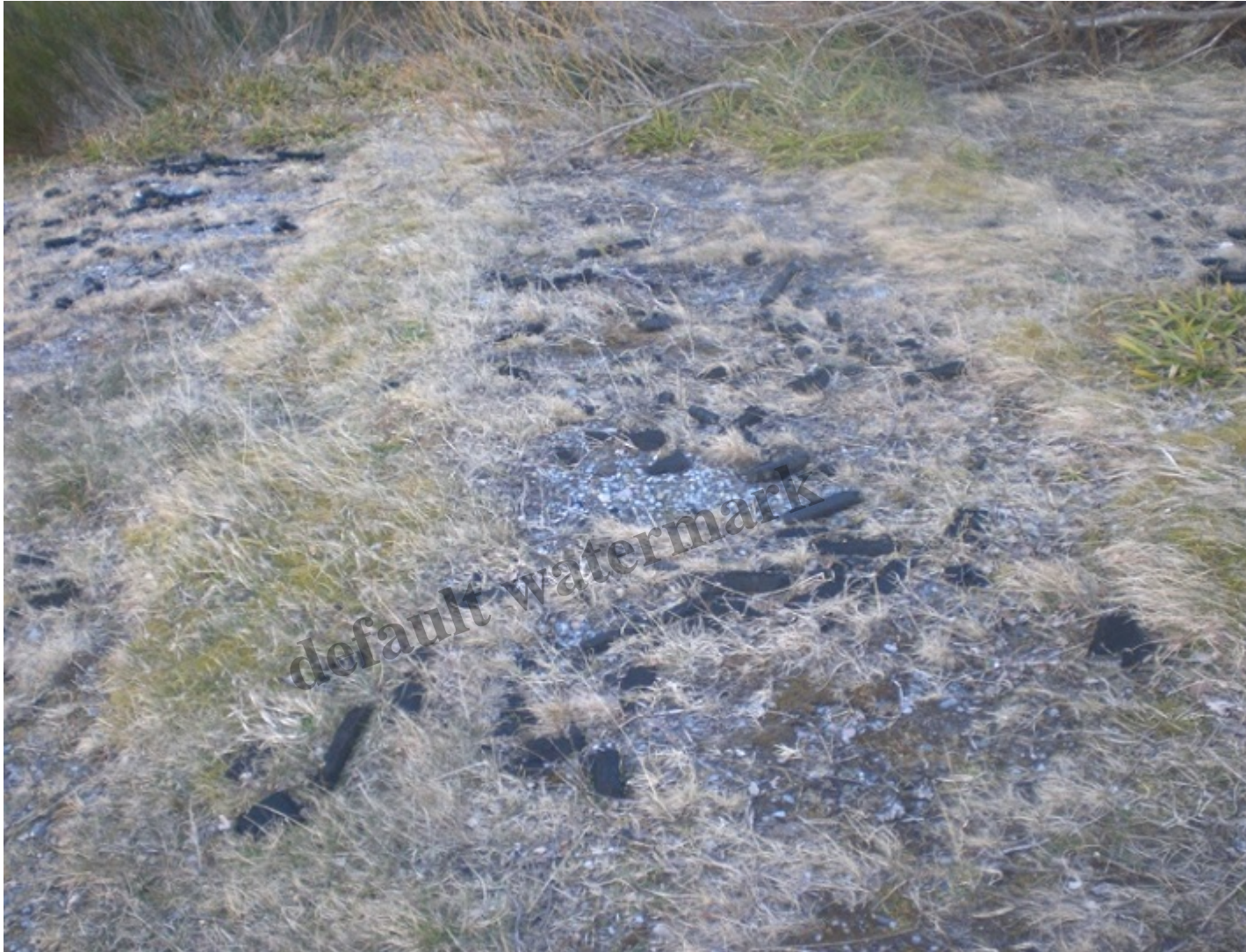
Perished rubber that has fallen off the Ciste chairs that were stored below the former chair lift for years
