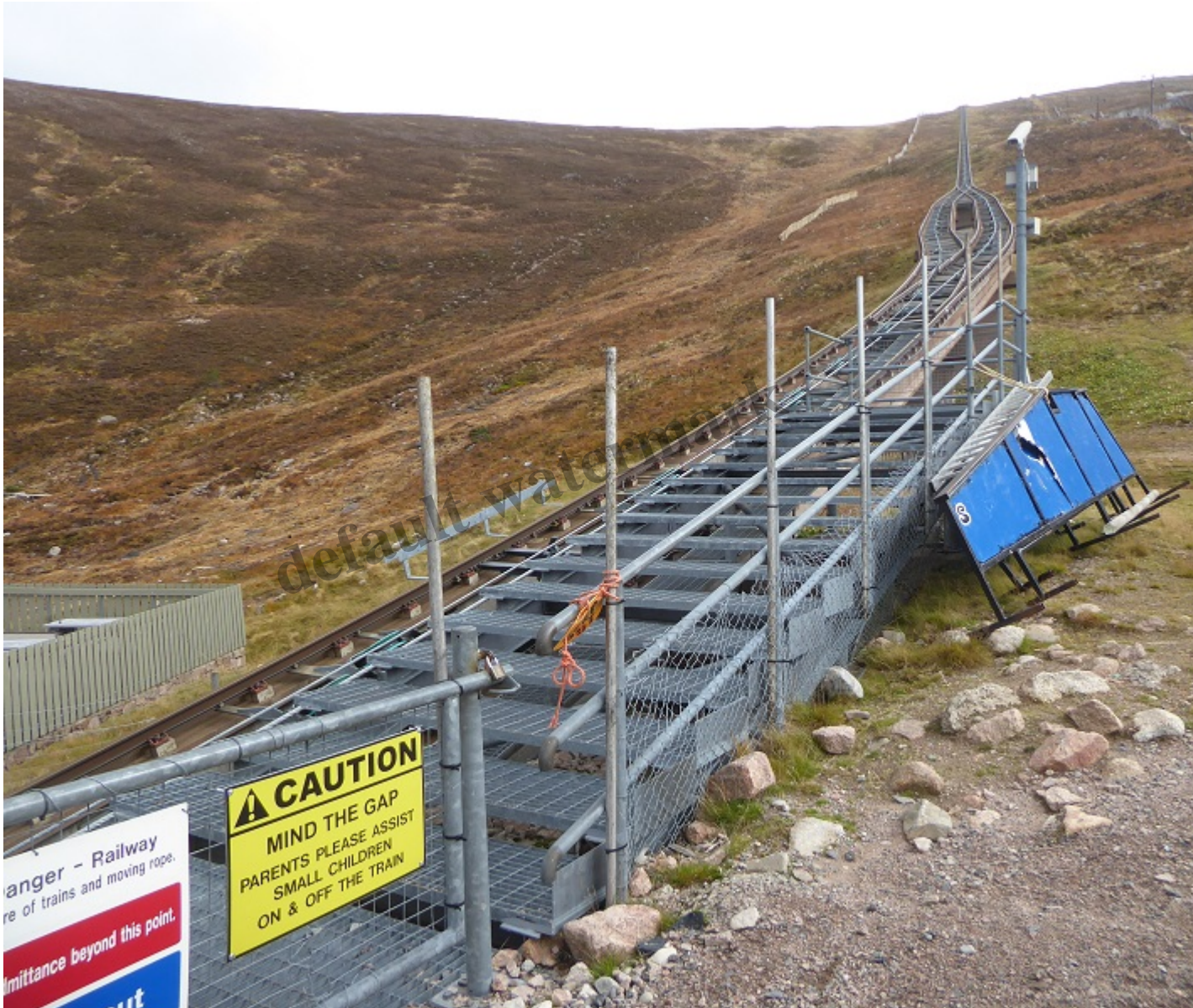
The mid-loading station October 2018, with the passing loop above
