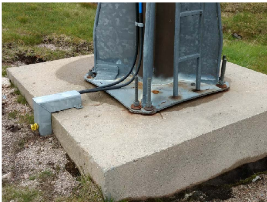
Photo 1 – base plate deformed by ice action.
