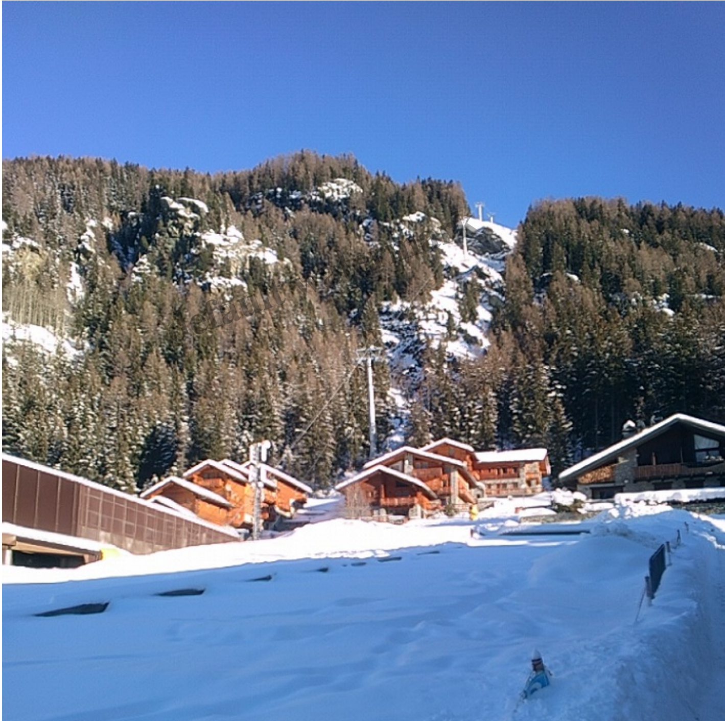
The replacement gondola at Champoluc, off the Aosta valley, in Italy. Four of the seven pylons are visible in the photo.
